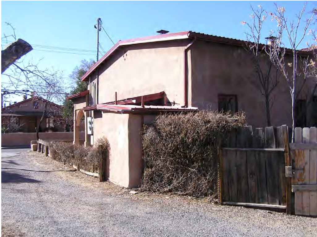
7 - North Façade (northeast corner)
