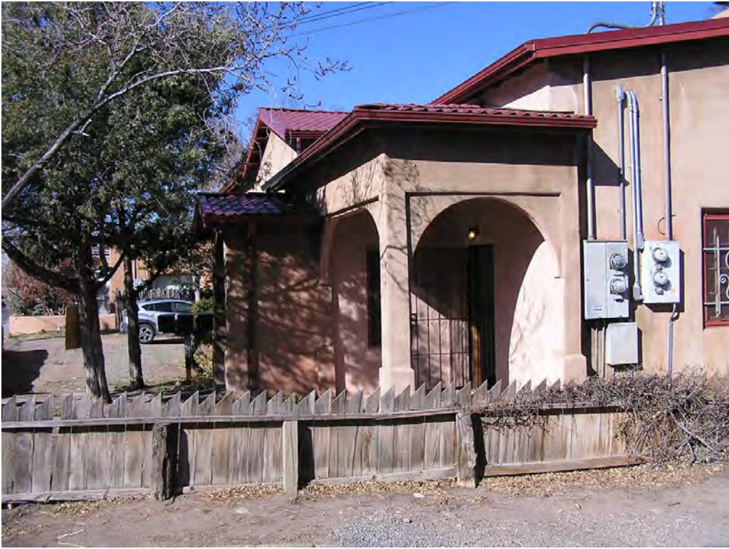
5 - East Façade (southeast corner)
