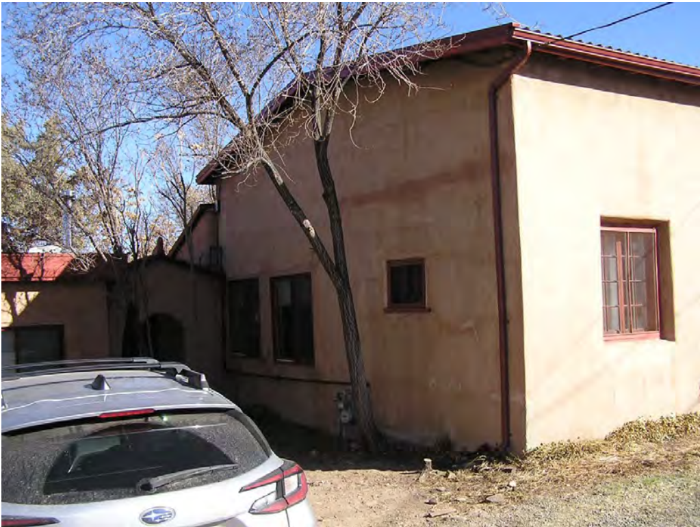
2 - South Façade showing west face of structure
