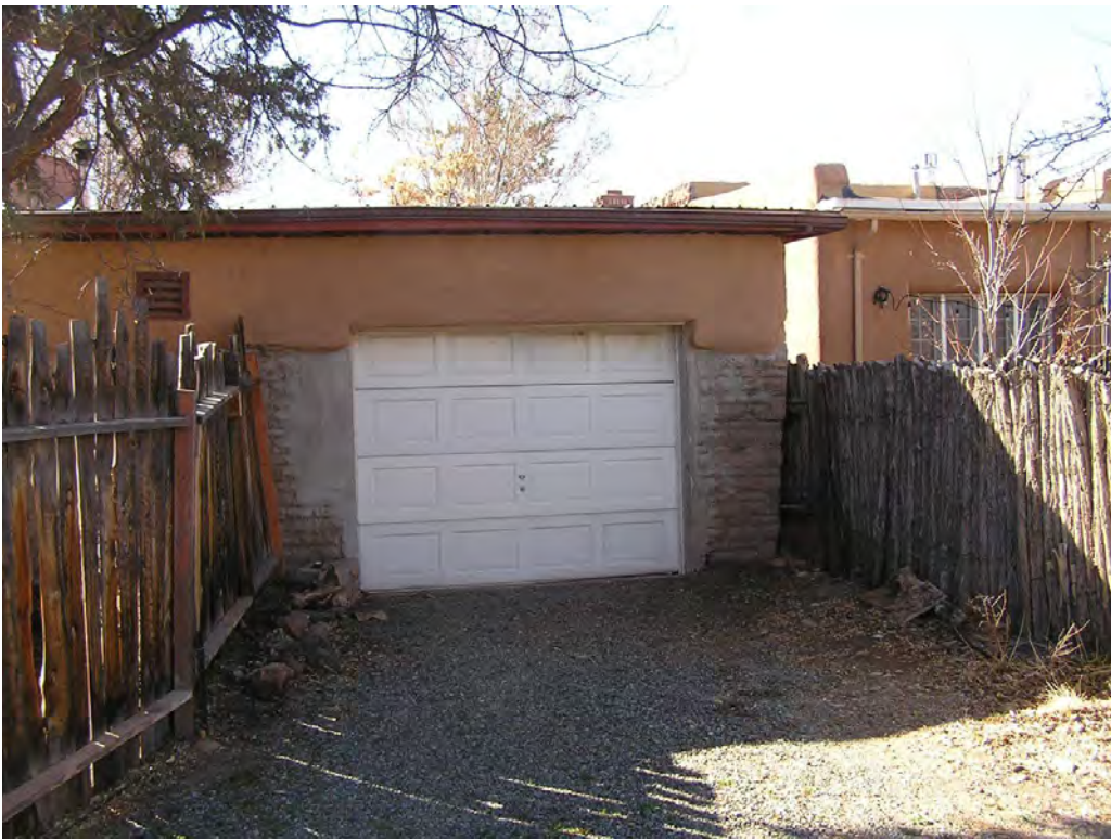
12 - North Façade (northwest corner)
