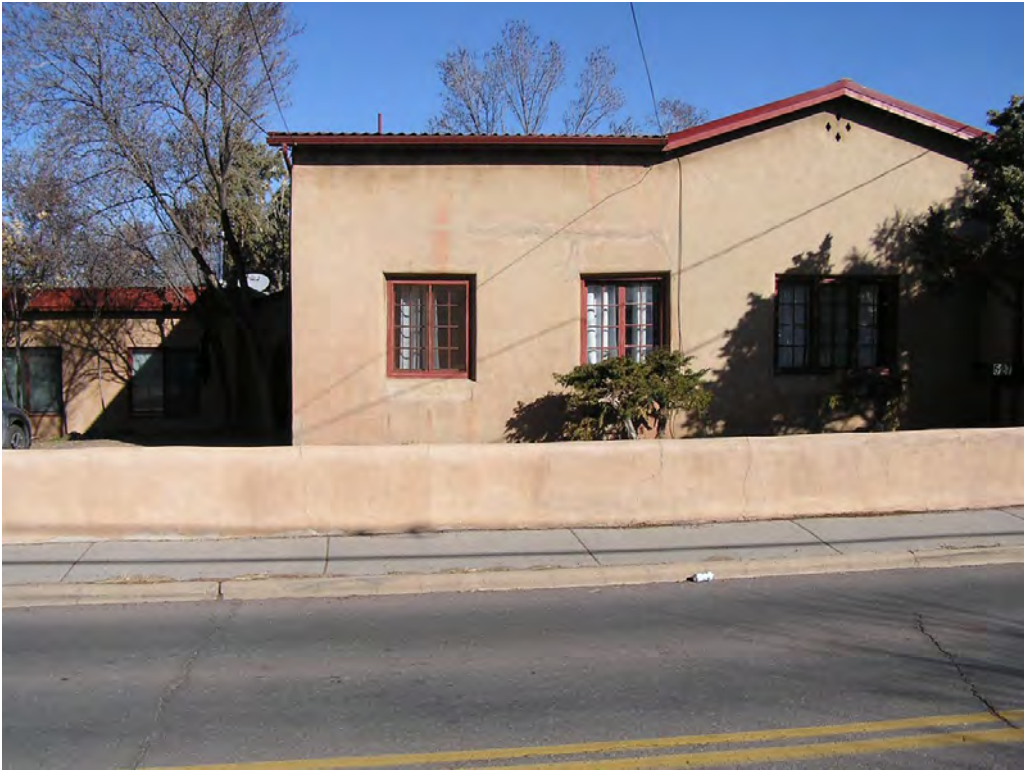
3 - South Façade (facing Agua Fria)
