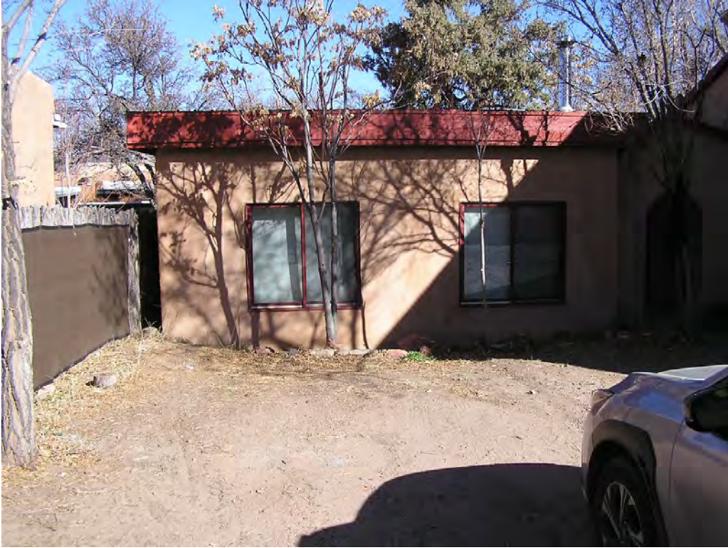
1 - South Façade (facing Agua Fria)
