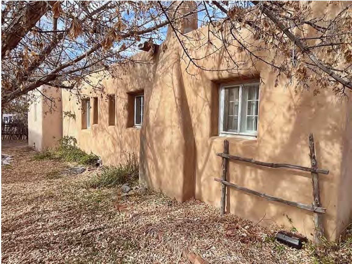
Photo 12: South elevation, east end. Camera facing northwest.
