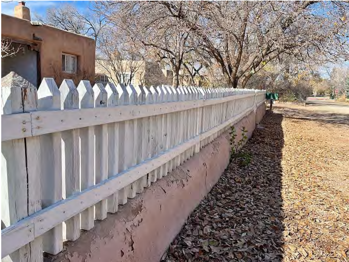
Photo 17: Fence/Wall. Camera facing northwest.
