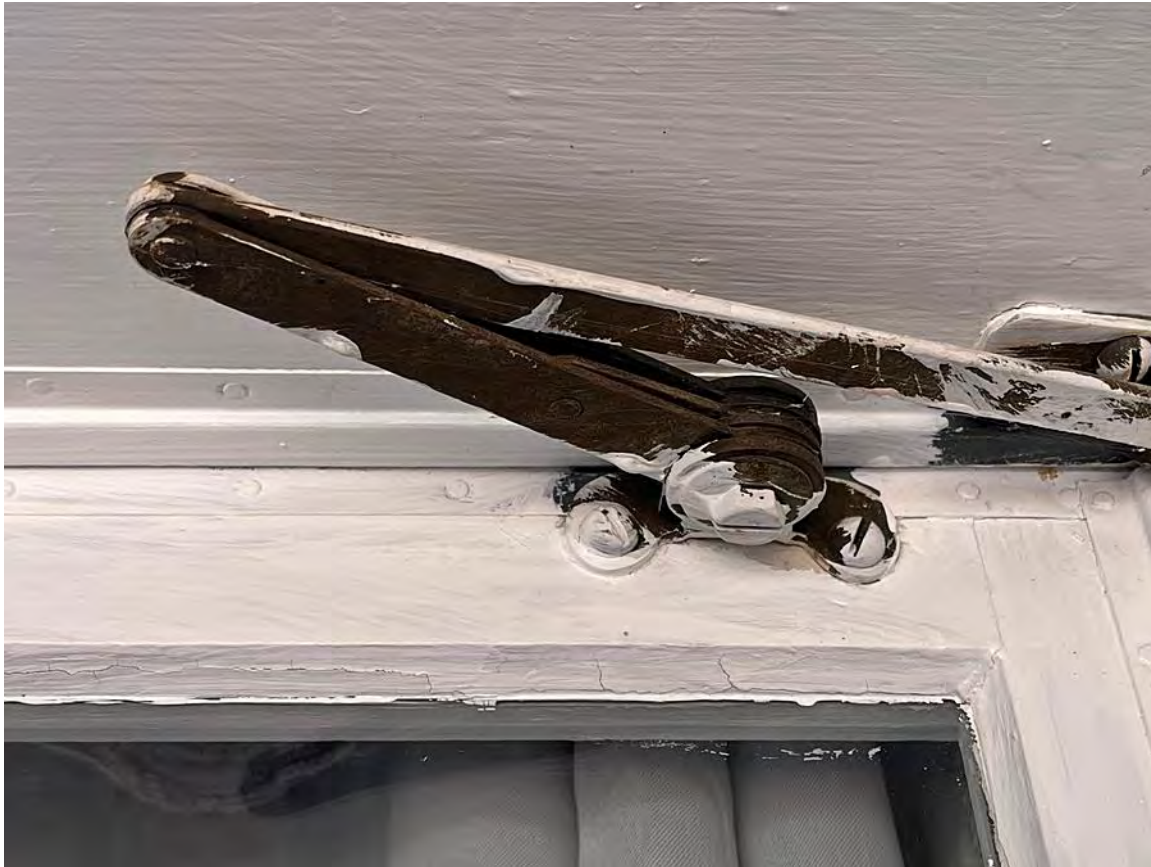
Photo 6: East (front) façade. Casement hinge. Camera facing up.
