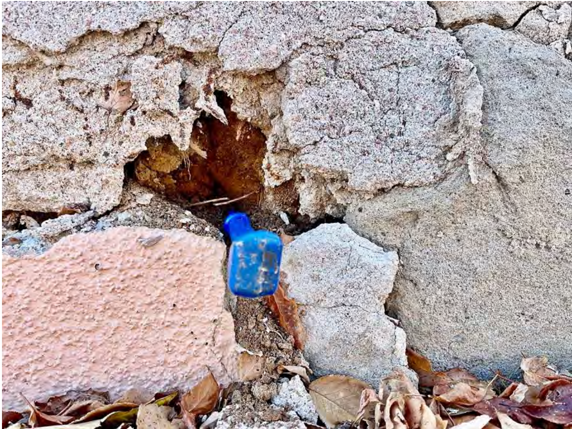
Photo 18: Fence/Wall. Adobe construction and stucco layers of base wall. Camera facing down.
