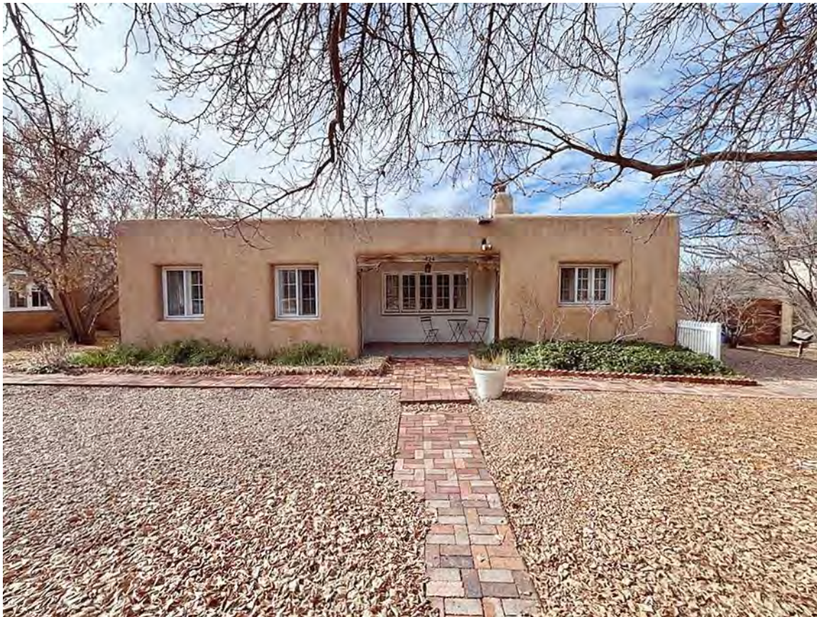
Photo 3: East (front) façade. Camera facing west.
