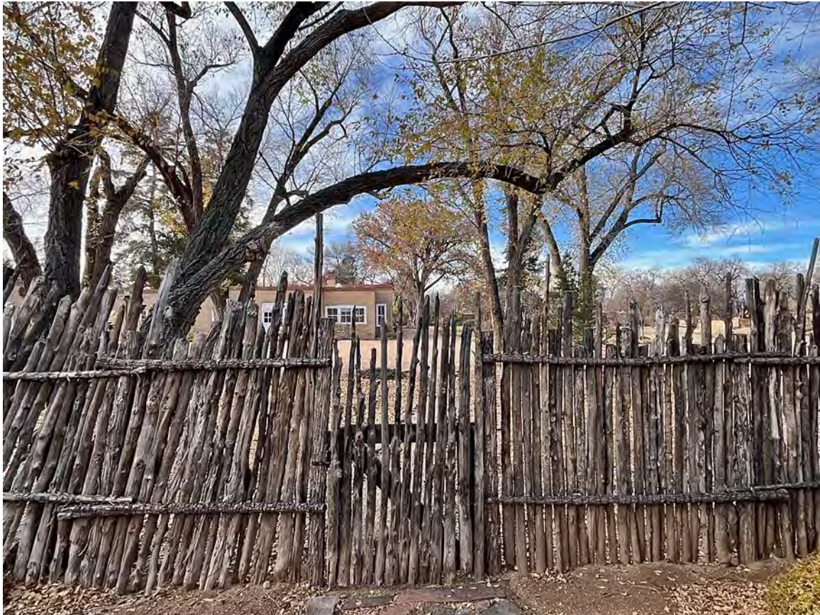
Photo 4: Coyote fence at rear of the lot. Camera facing west.
