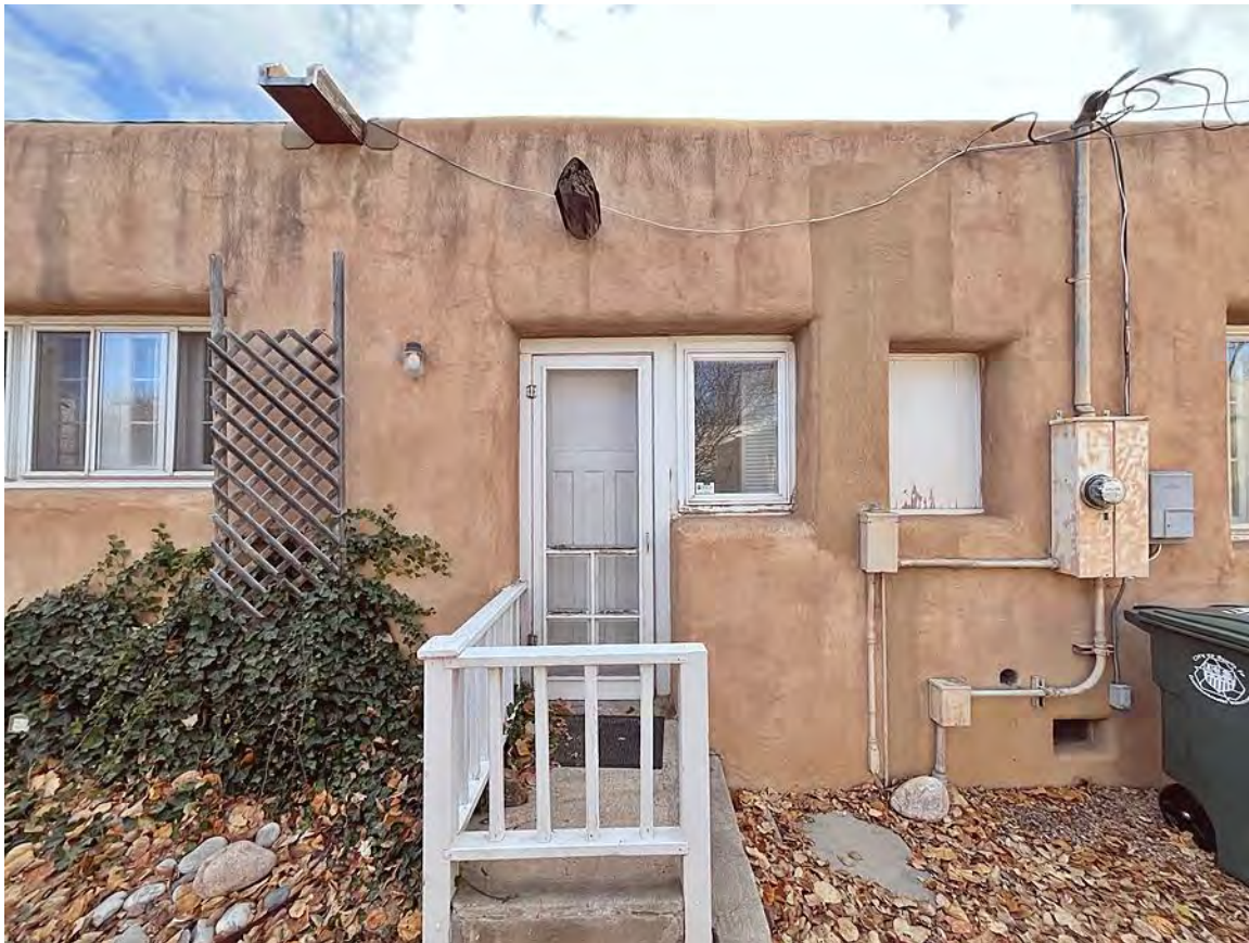
Photo 10: North elevation. Entry door. Camera facing south.
