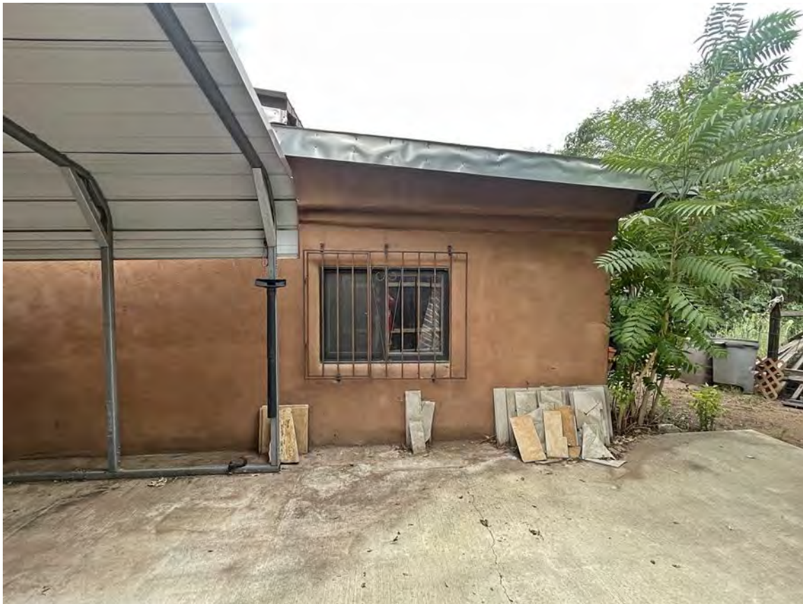
Photo 8: North elevation. Camera facing south.
