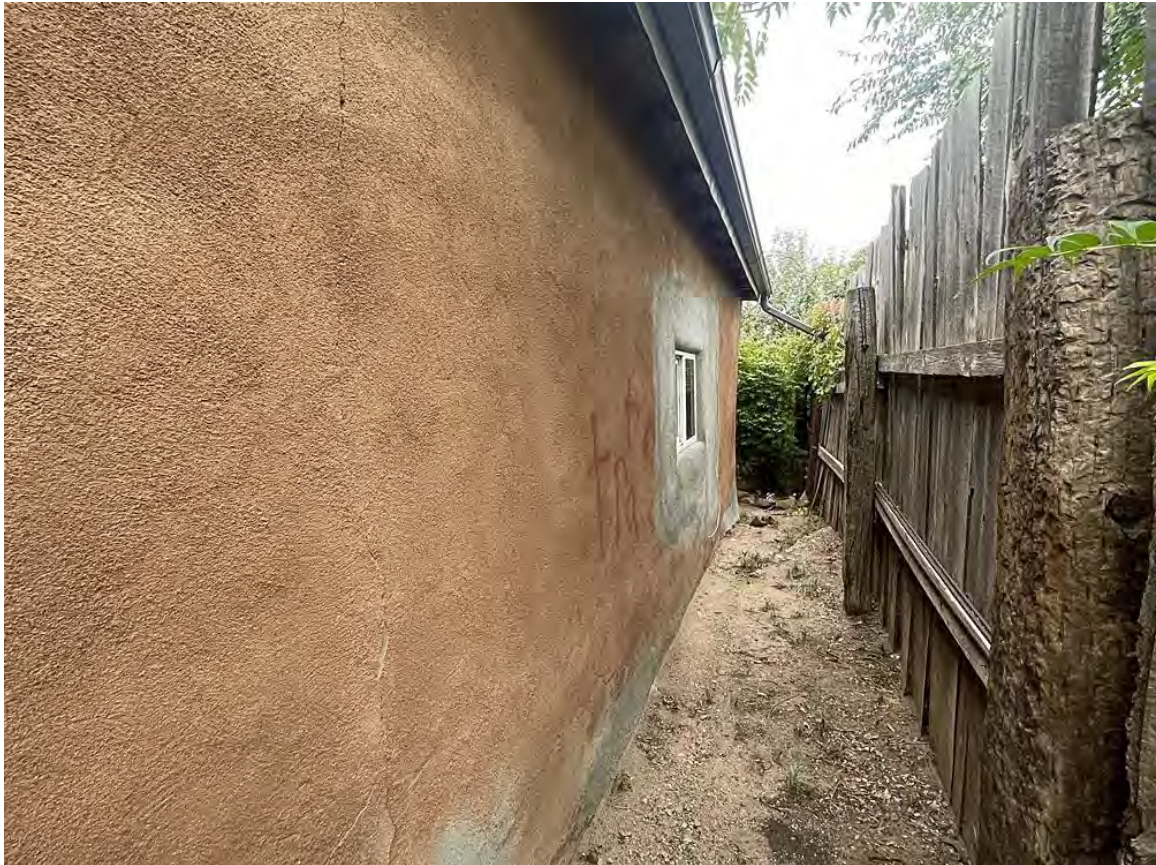
Photo 11: West elevation. Camera facing southeast.
