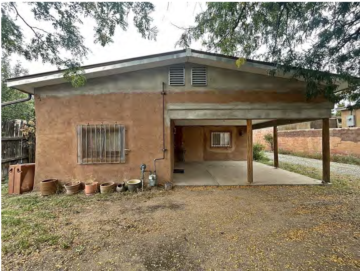
Photo 3: South (front) elevation. Camera facing north.
