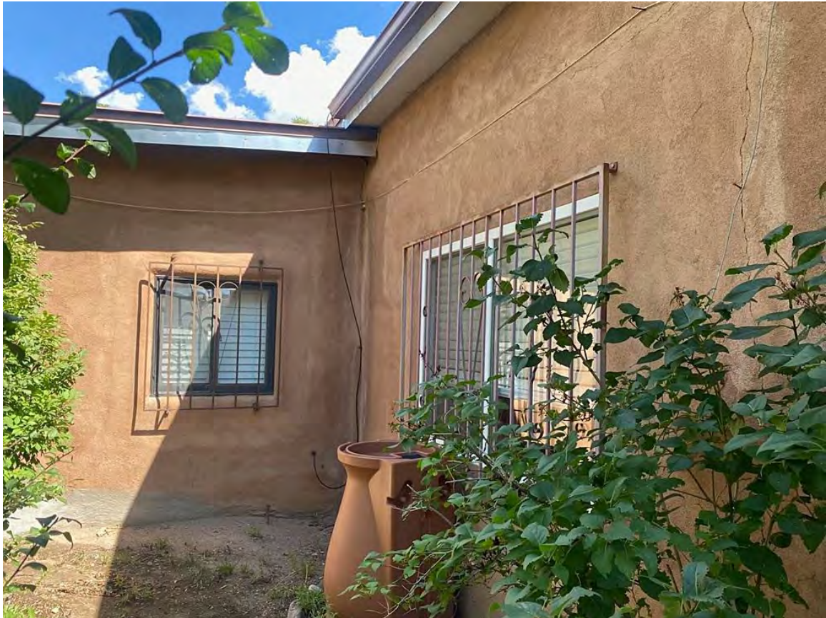
Photo 10: West elevation. Camera facing northeast. Photo by Kris Murphey, September 12, 2025.
