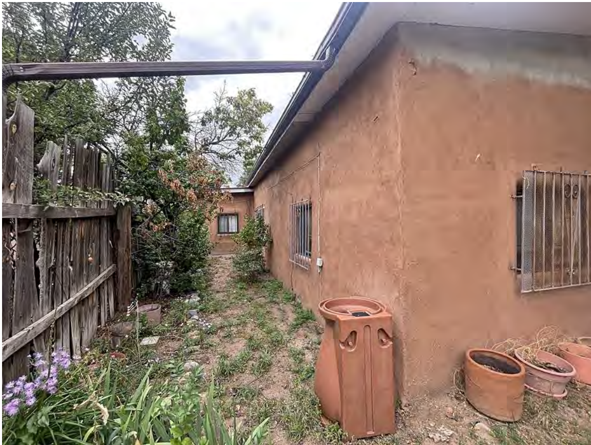
Photo 9: West elevation. Camera facing north.
