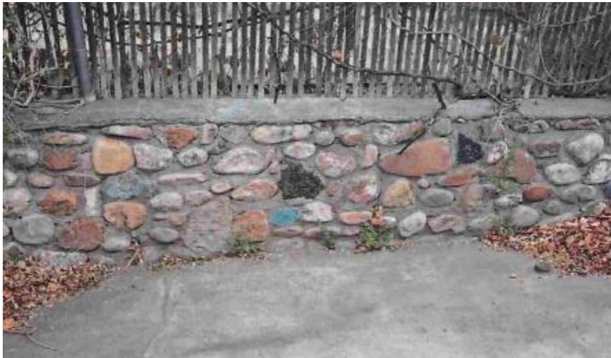
Figure 3: North Retaining Wall
