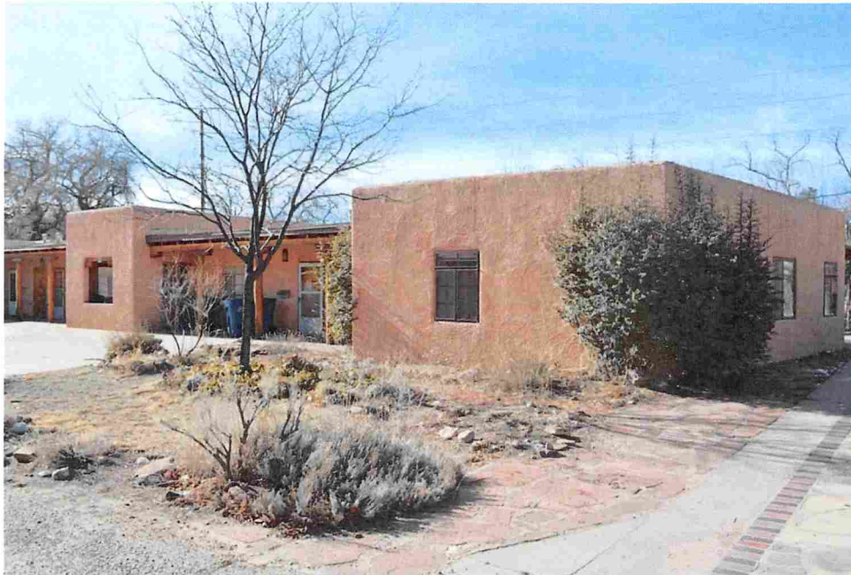
Photo 1: Street and north elevations, facing southeast.
