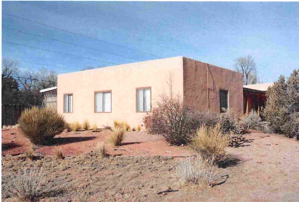
Photo 2: South elevation, facing north.
