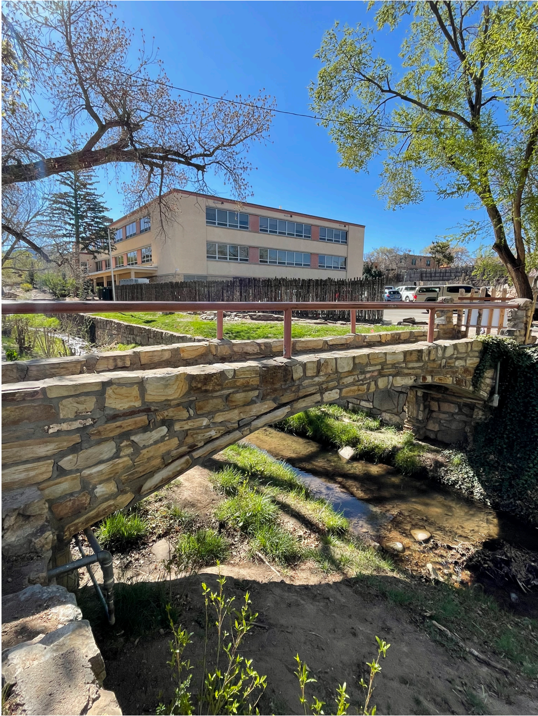
Figure 2. Shelby Street Footbridge, west elevation, view east.
