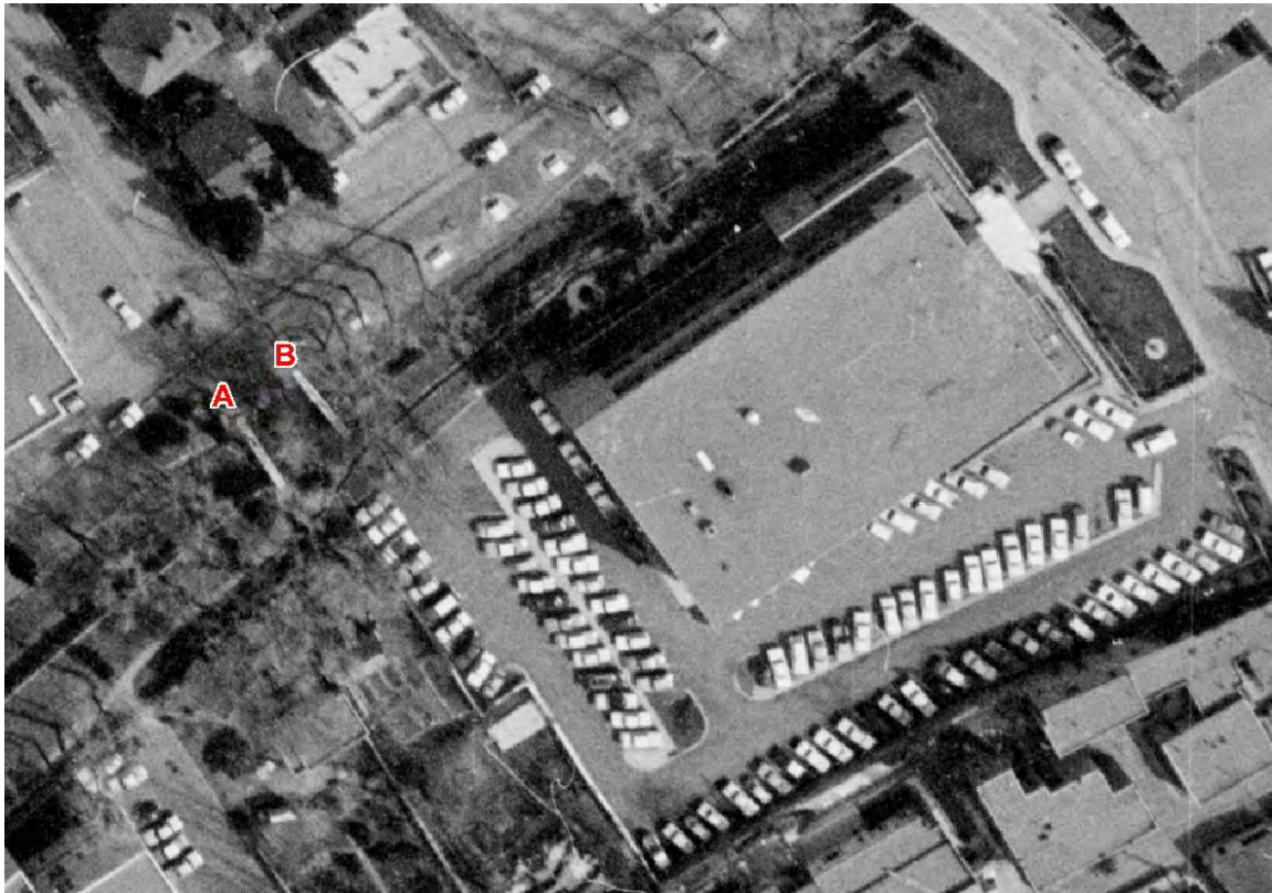
Figure 5: February 2, 1968, aerial photograph showing two bridges at the Shelby Street crossing. A. is the bridge erected 1968; B. is likely the CCC -constructed built in 1934.
