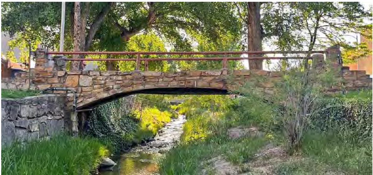
Figure 2: Side view of Shelby Street Footbridge.
