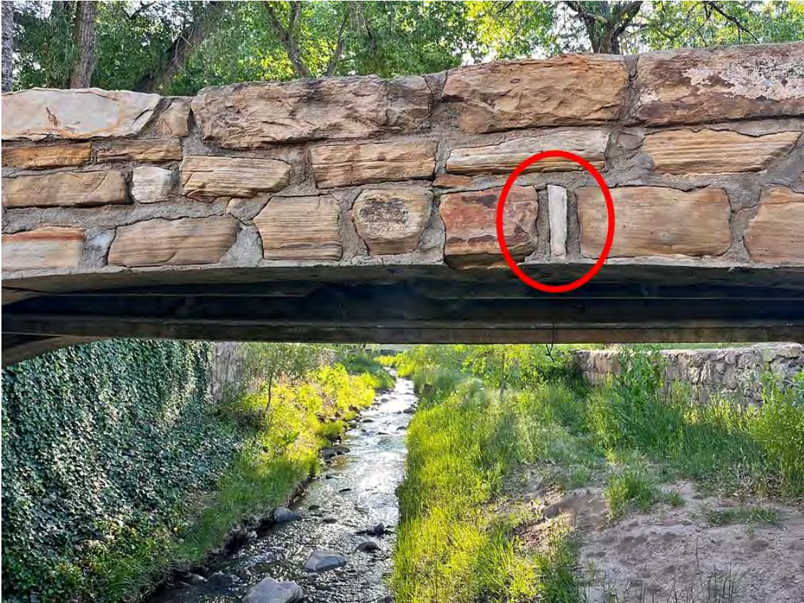
Photo 7: Crown of false spandrel wall with “keystone” highlighted.
