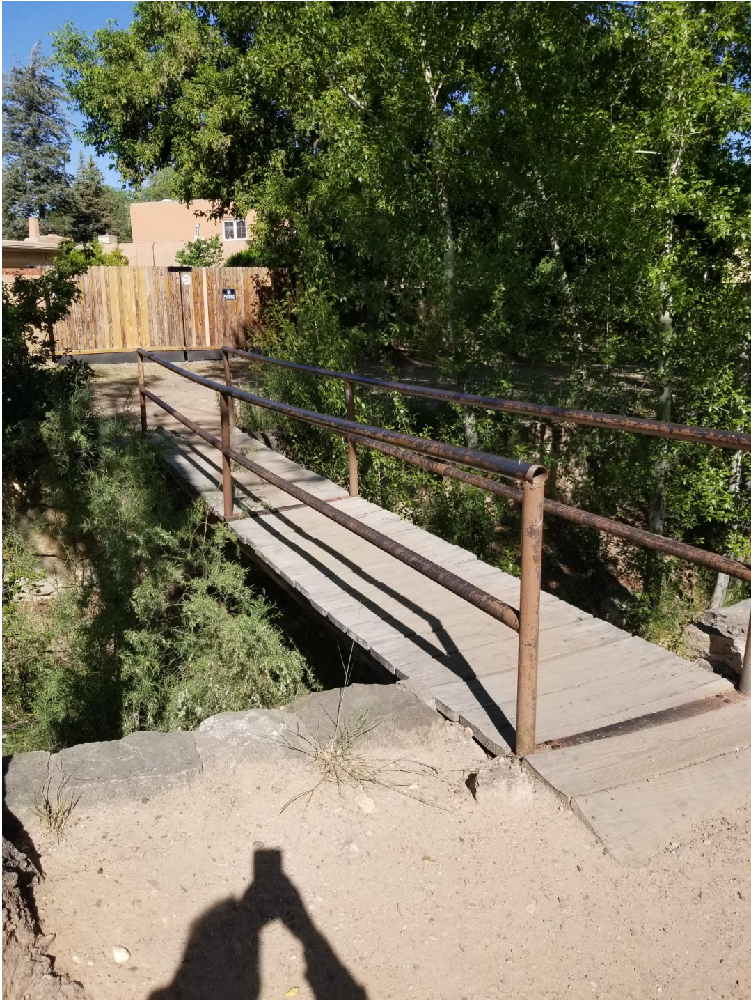
Figure 4. Bridge Style 1, metal pipe railing with narrow wooden deck.
