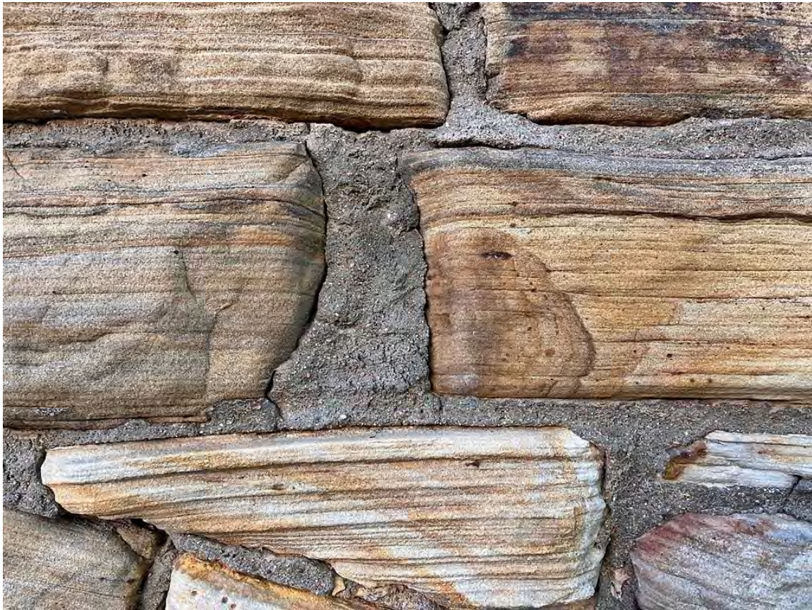
Photo 6: Exterior stonework of false spandrel wall.
