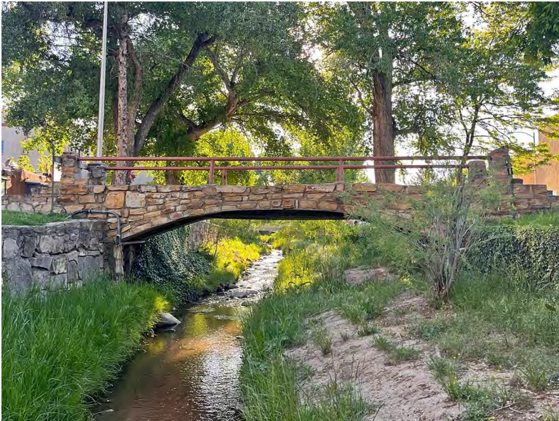
Photo 3: River and channel context. Camera facing west.
