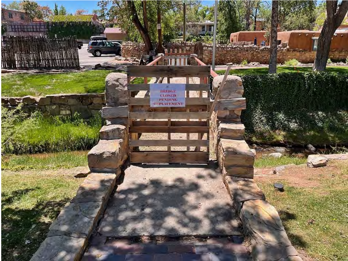
Photo 10: North approach. Camera facing south.
