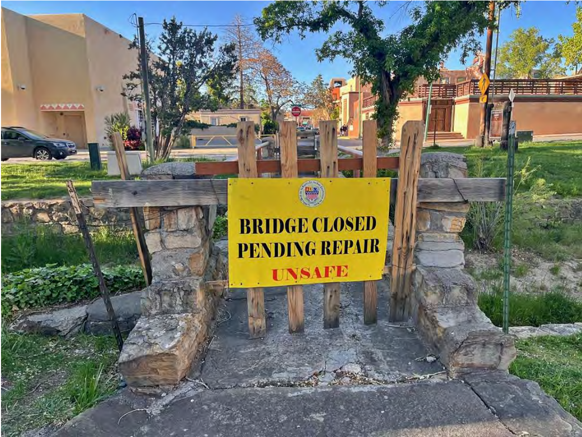
Photo 2: South approach. Camera facing north.
