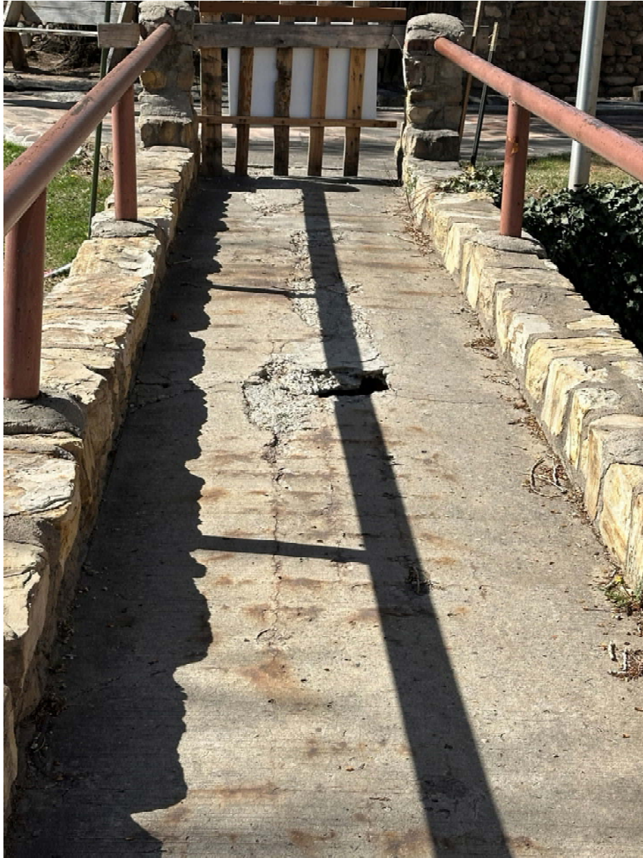
Figure 4 – Top of flange damage
