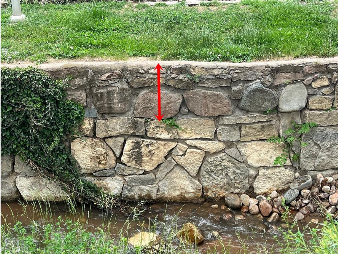
Figure 4: Contemporary photograph showing where the river retaining walls were extended in the early 1950s to create the Santa Fe River Park.
