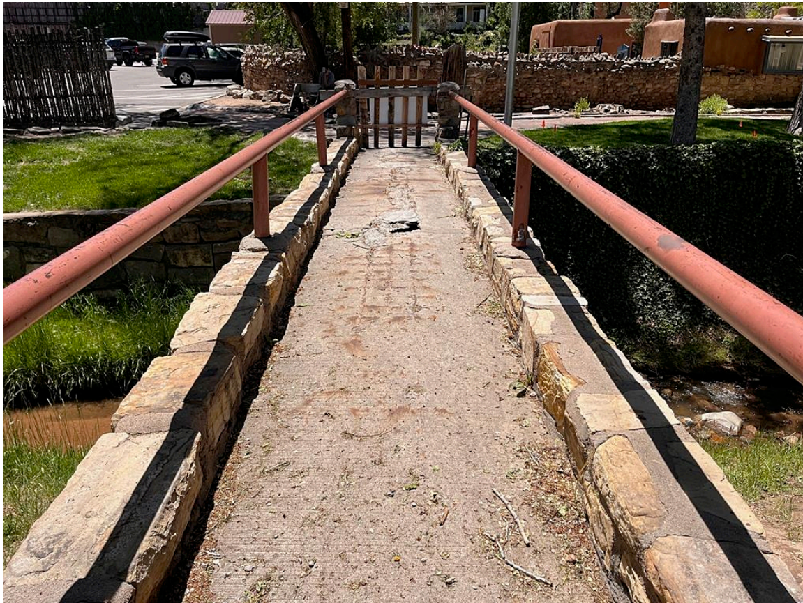
Photo 9: Deck and railing. Camera facing south.
