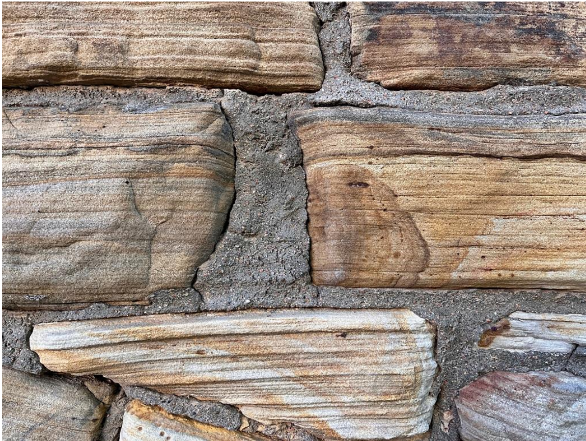
Photo 6: Exterior stonework of false spandrel wall.
