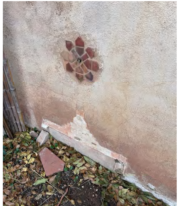
North Elevation - northeast corner of house - thickened wall at exterior with decorative tile and broken spigot (remnants of a fountain)
