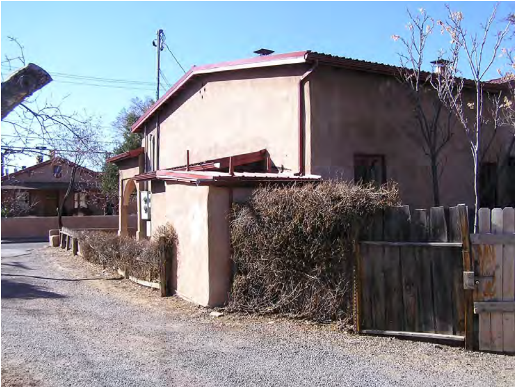
7 - North Façade (northeast corner)
