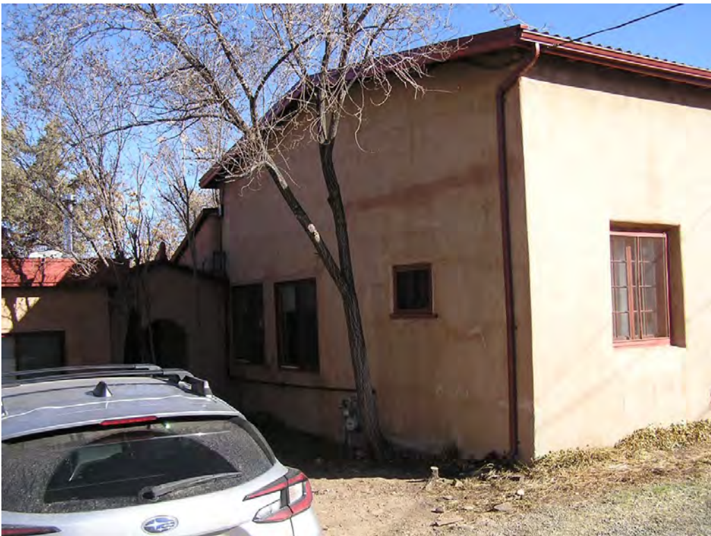
2 - South Façade showing west face of structure
