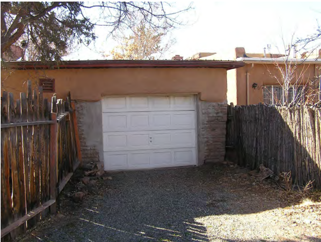
12 - North Façade (northwest corner)
