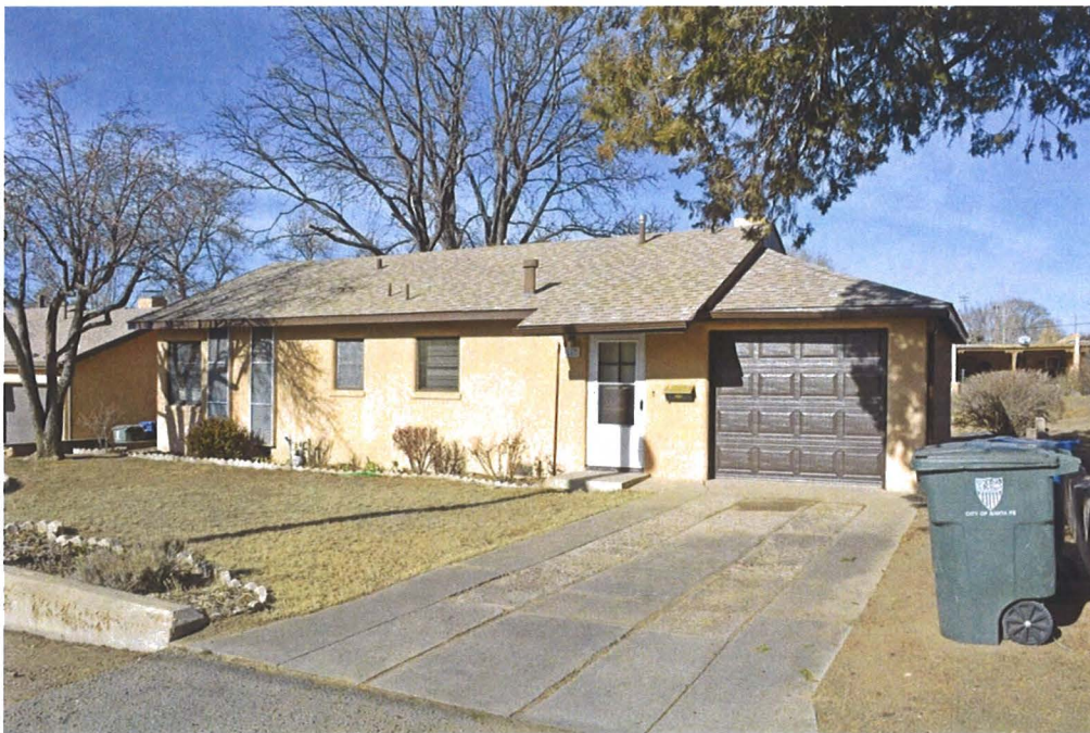
Photo 2: Street and east elevations, facing northeast.
