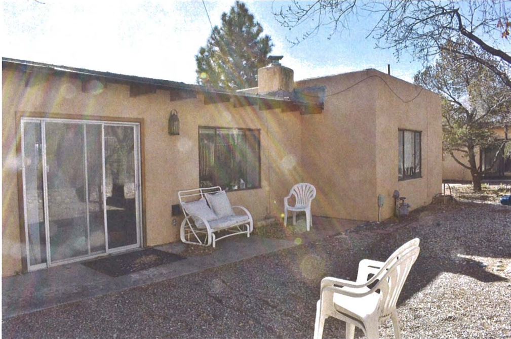
Photo 3: North elevation, facing southwest (Sharon Joyce, February 23, 2018).
