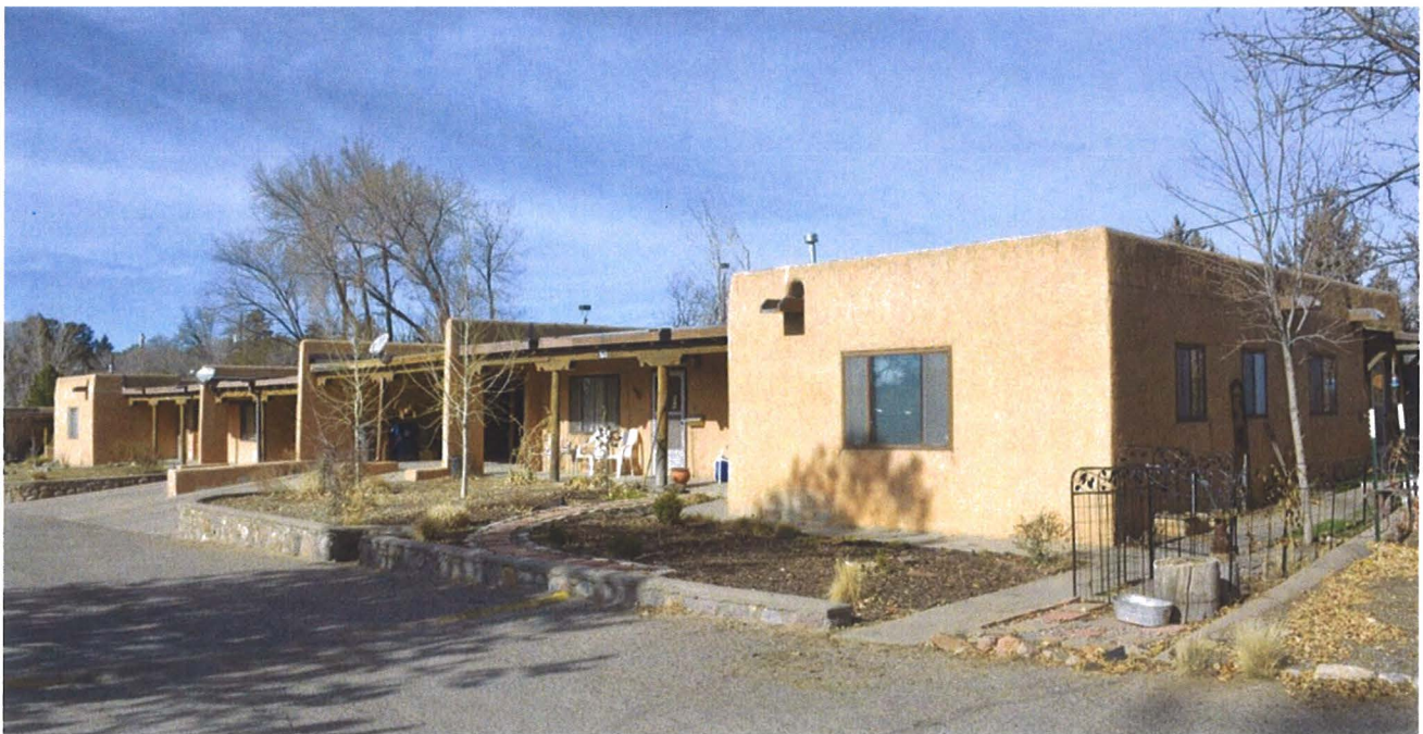
Photo 1: Street elevation and east elevations, facing northwest.
