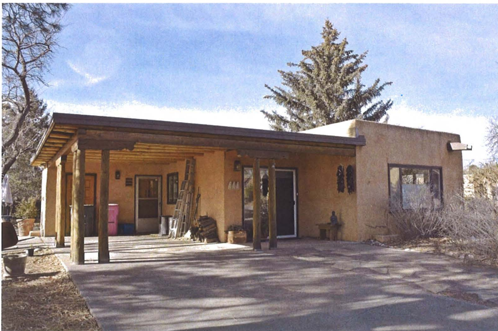
Photo 1: East and south elevations, facing northeast.
