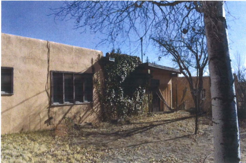
Photo 2: West elevation, facing southwest (Sharon Joyce, February 23, 2018).
