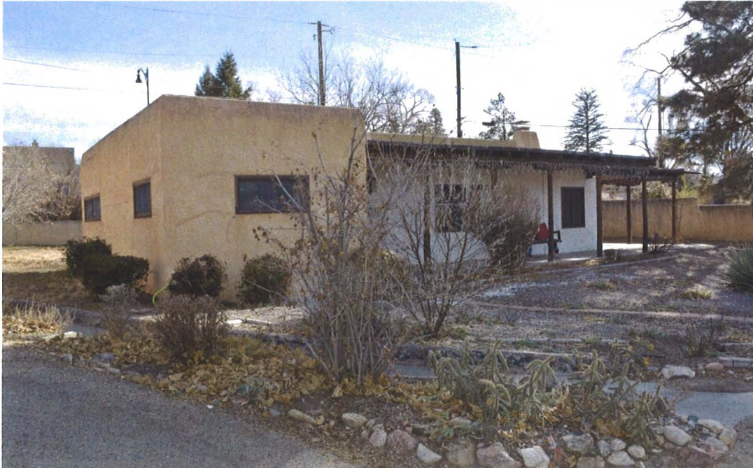
Photo 2: Street and north elevations, facing southeast.
