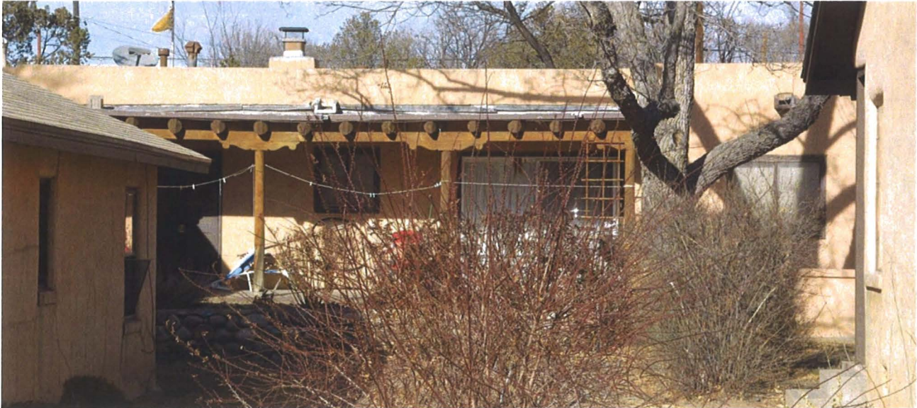
Photo 4: South elevation, facing north.
