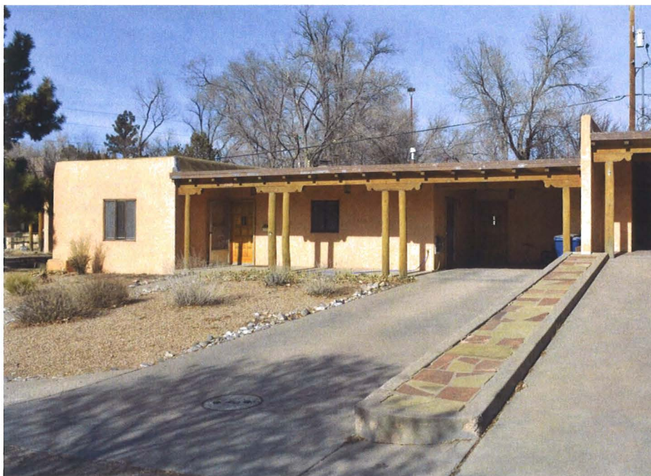
Photo 1: Street and east elevations, facing northwest.
