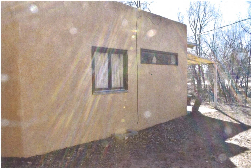
Photo 3: North elevation, facing southwest (Sharon Joyce, February 23, 2018).
