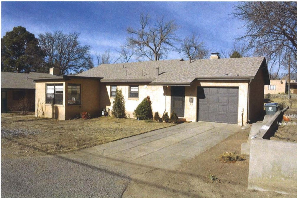
Photo 1: Street and east elevations, facing northwest.
