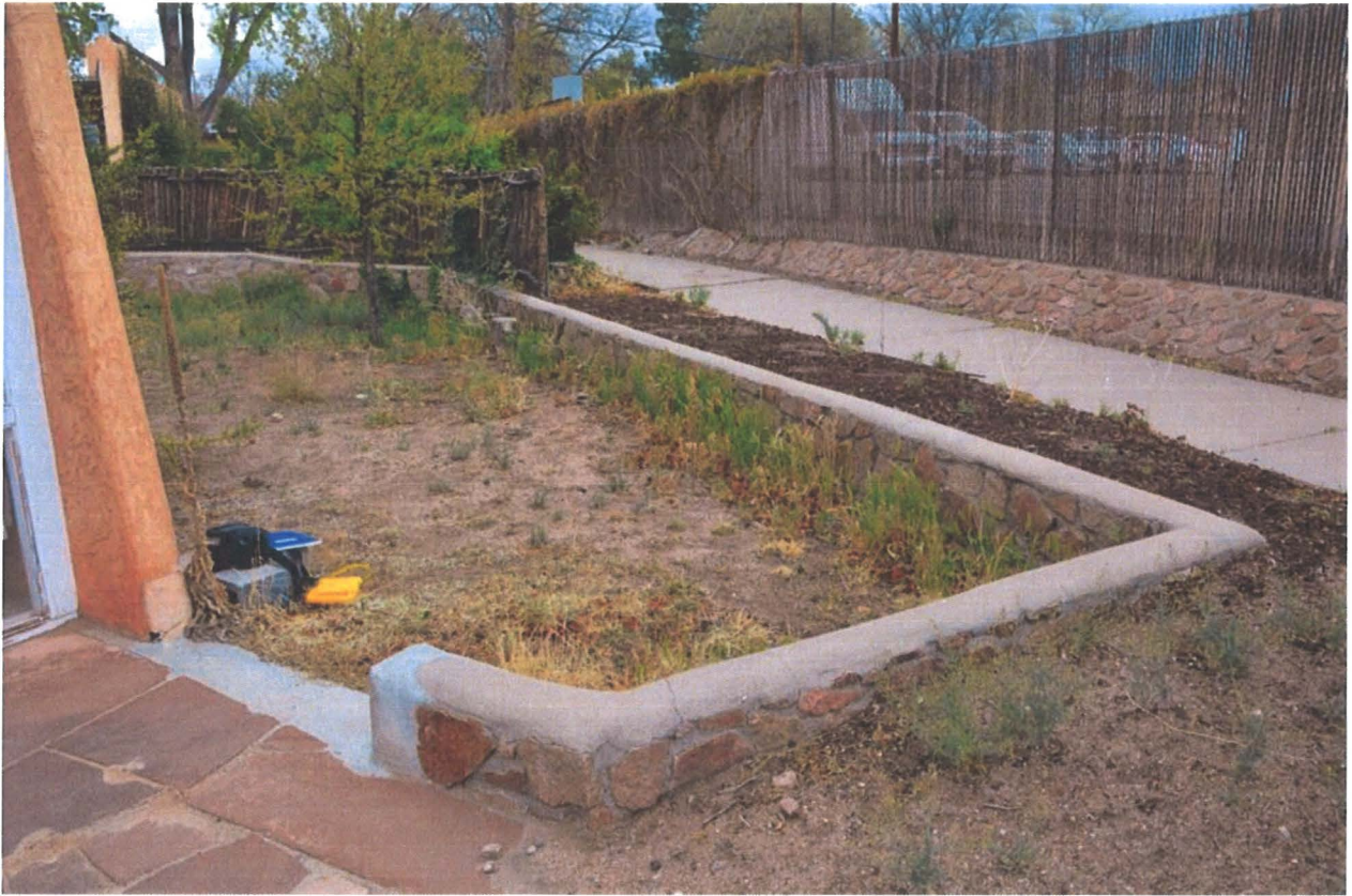
Figure 2: 124 Camino Santiago, rear retaining wall, May 3, 2018.
