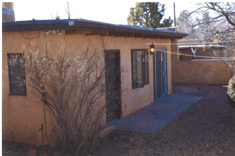
Photo 2: North elevation, facing southeast and southwest (Sharon Joyce, February 23, 2018).
