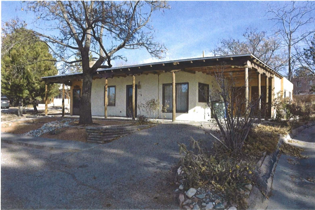
Photo 1: Street elevation and south elevations, facing northeast.
