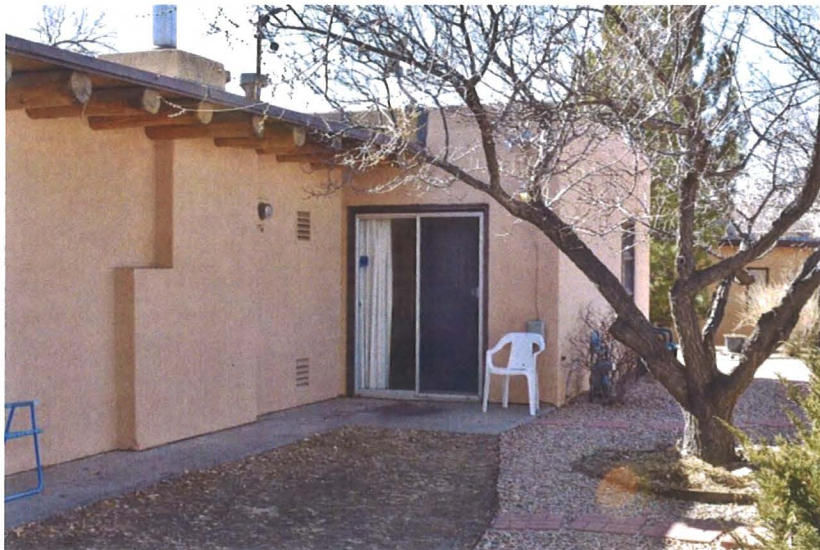
Photo 3: North elevation, facing southwest (Sharon Joyce, February 23, 2018).
