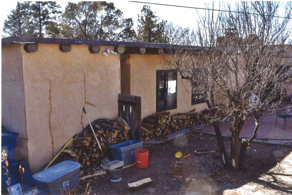
Photo 3: North elevation, facing southwest (Sharon Joyce, February 23, 2018).
