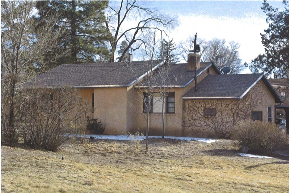
Photo 3: North elevation, facing southeast.
