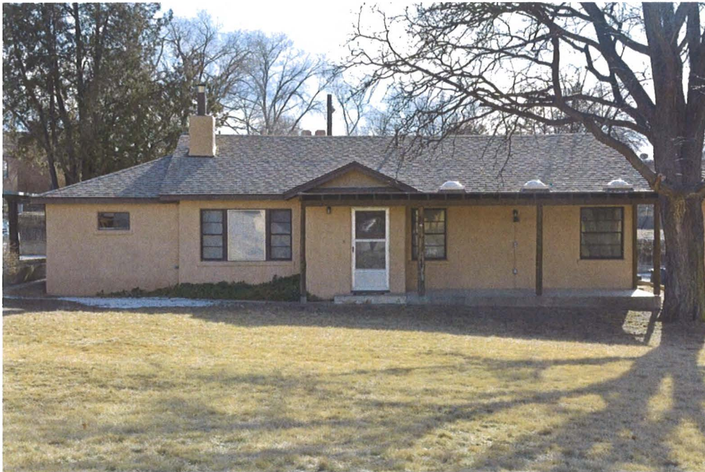
Photo 2: North elevation, facing south.
