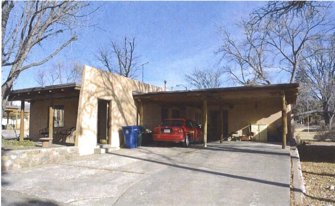
Photo 3: South and west elevations of addition and expanded carport, facing east.
