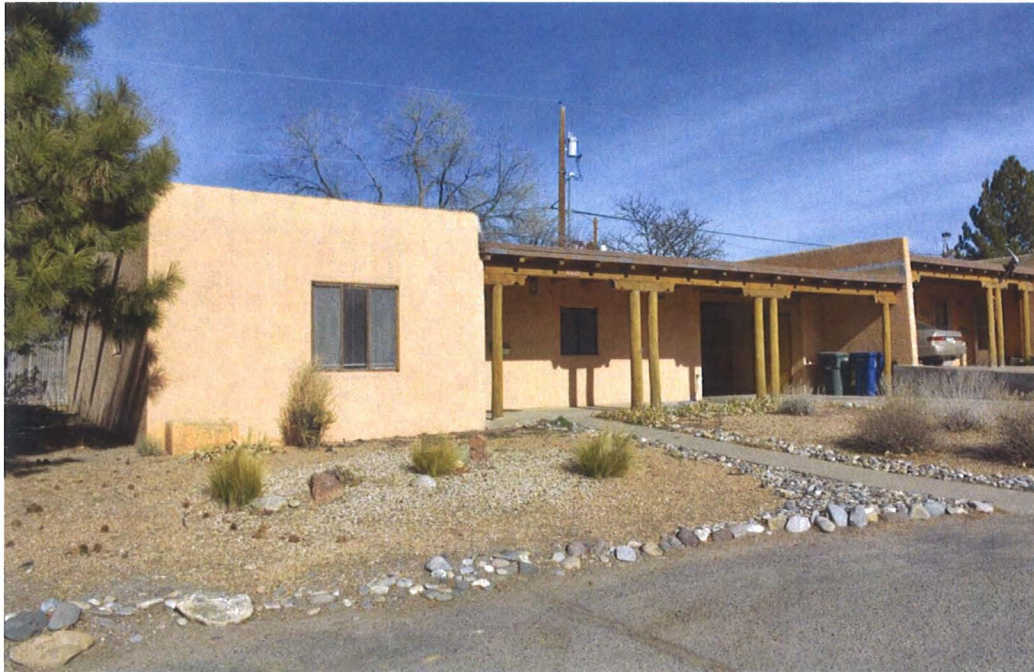
Photo 2: Street and west elevations, facing northeast.
