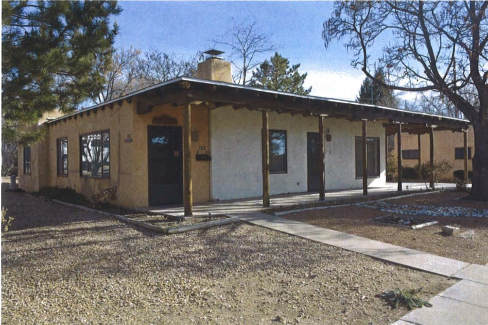
Photo 2: North and street elevations, facing southeast.
