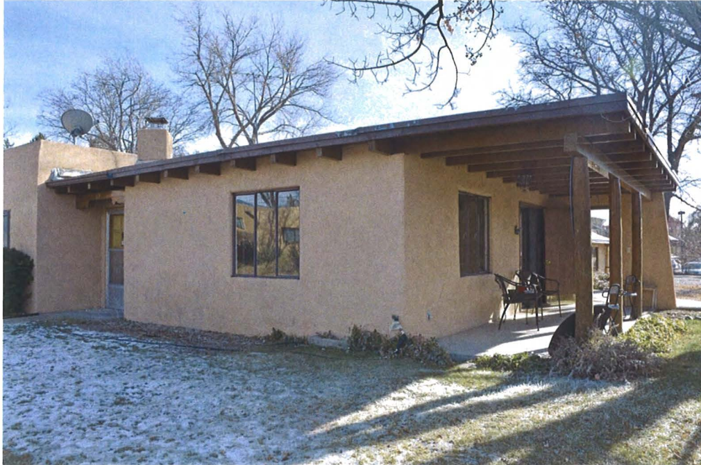
Photo 2: Street and west elevations of addition, facing northeast.
