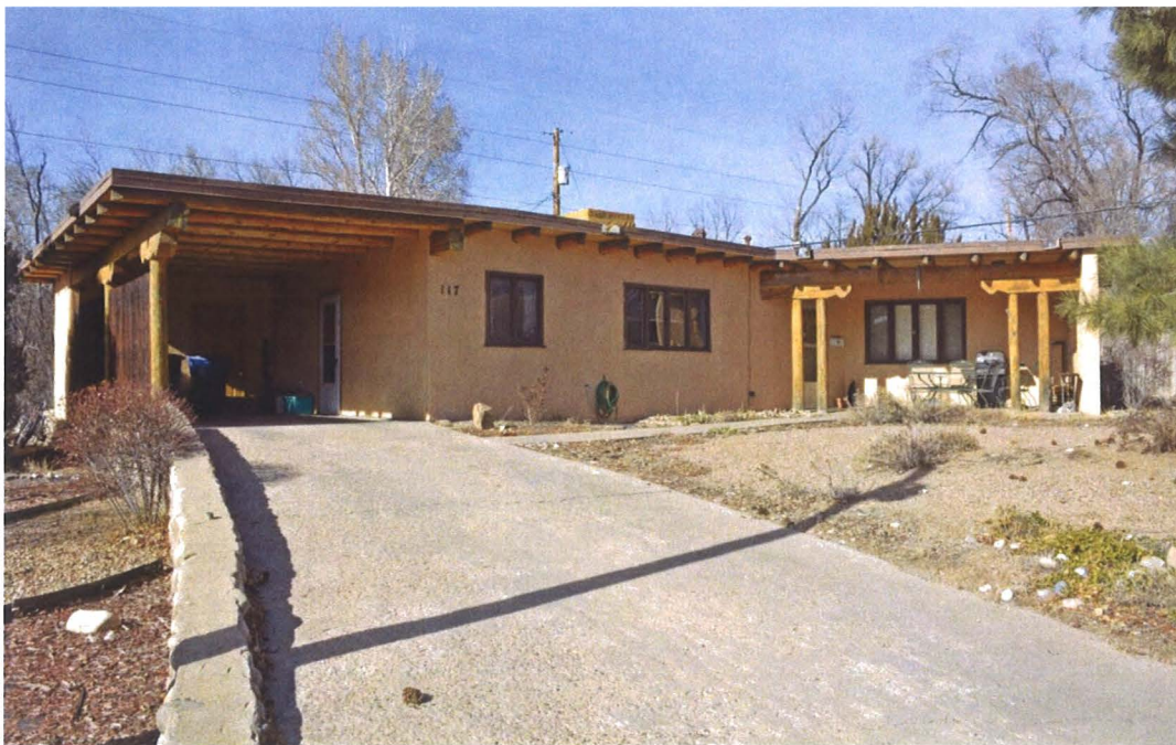
Photo 1: Street, west and south elevations, facing northeast.
