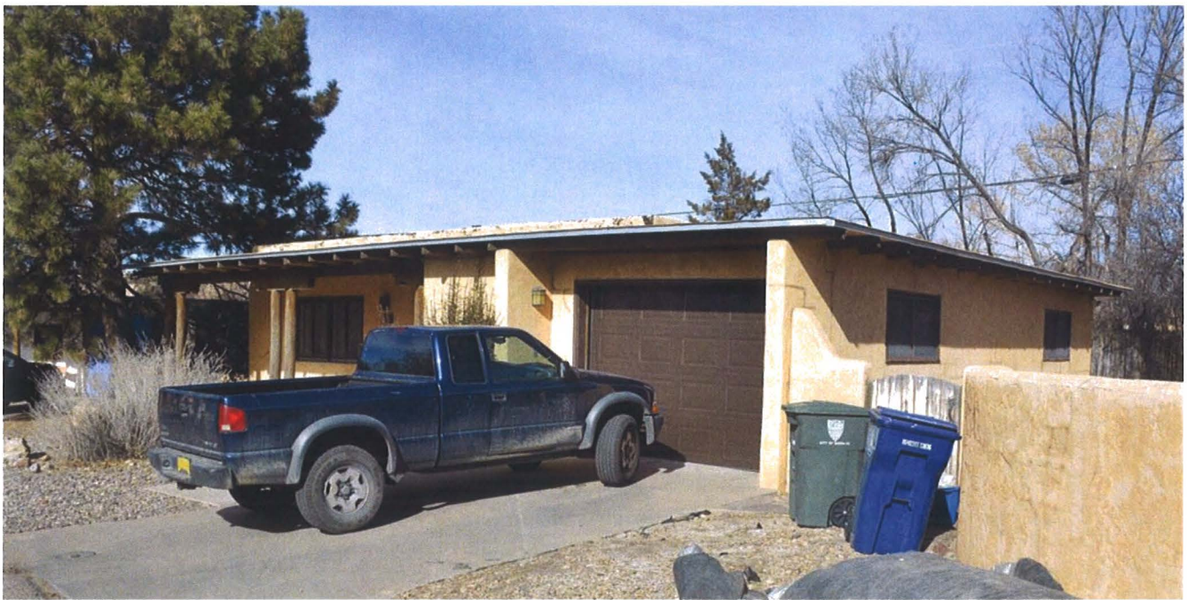
Photo 1: Street elevation and north elevations, facing northwest.
