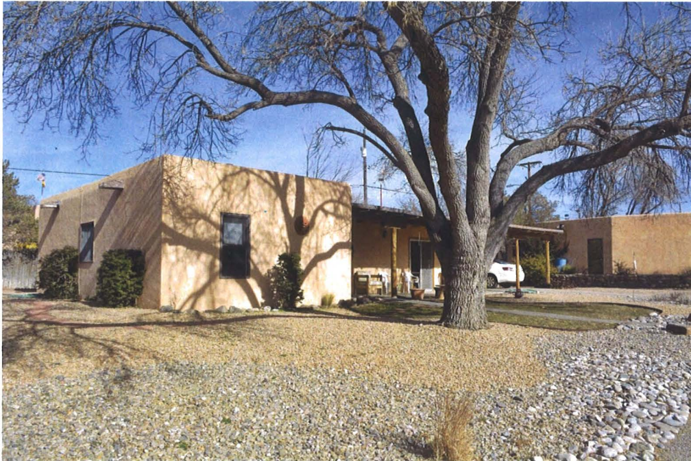
Photo 2: Street and west elevations, facing northeast.
