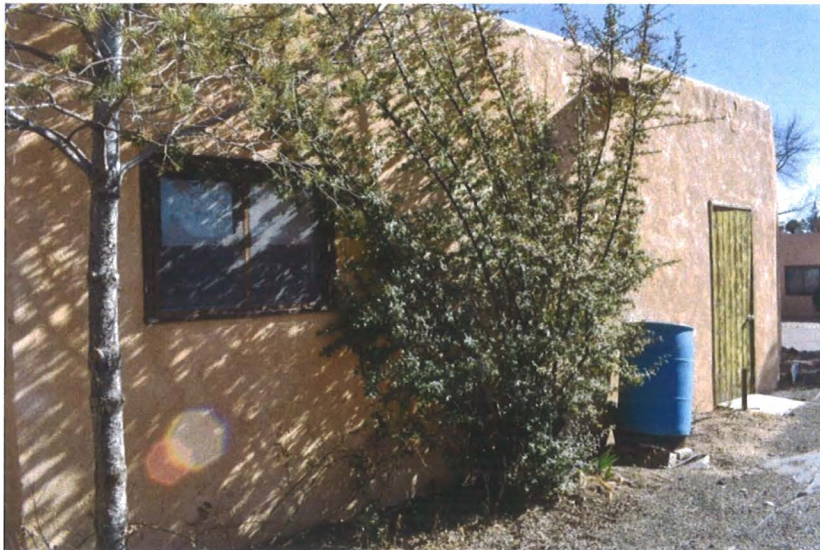
Photo 2: Street and west elevations (top), facing northeast. West elevation (bottom), facing southeast (Sharon Joyce, February 23, 2018).
