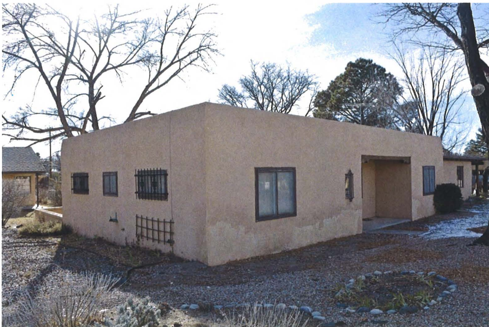
Photo 1: Street and north elevations, facing southeast.
