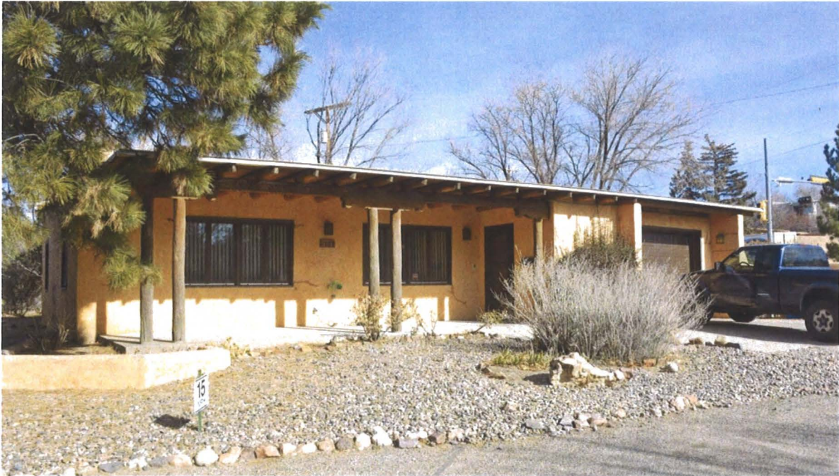
Photo 2: Street and west elevations, facing northeast.
