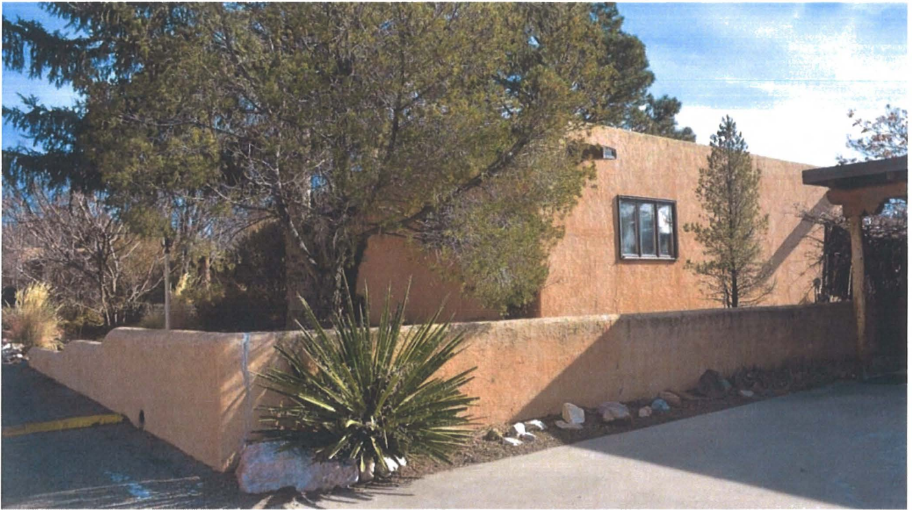
Figure 4: Stucco-on-block property wall between 114 and 118 Camino Santiago, January 18, 2018.
