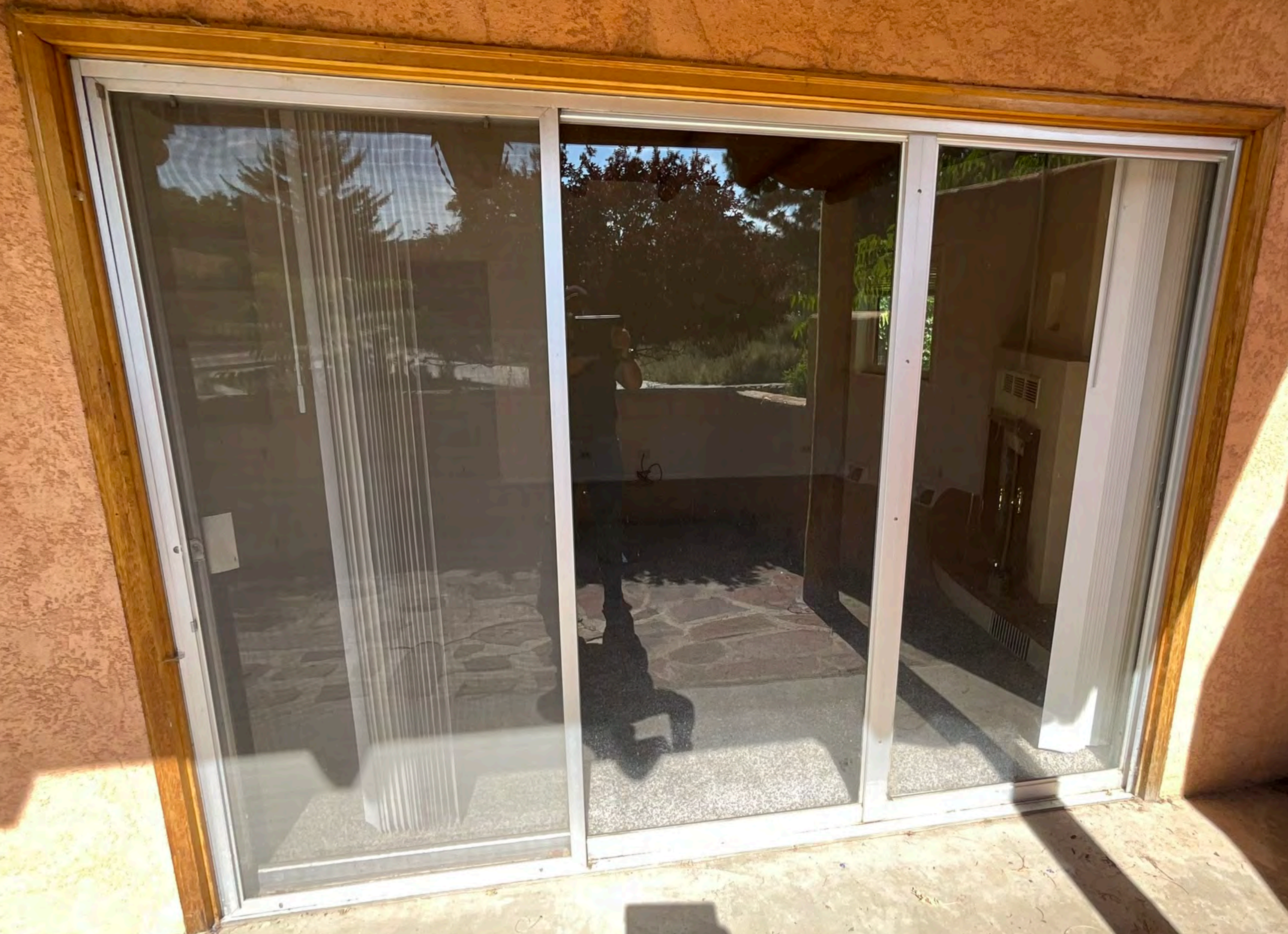
East Elevation Door #4
