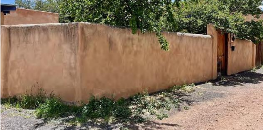
Figure 7: West Yard Wall
