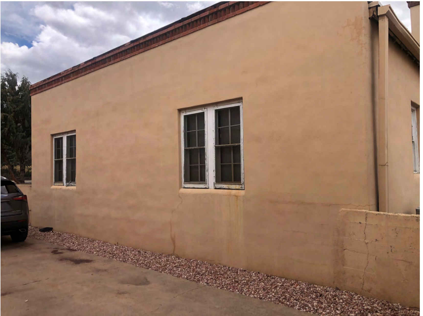
414 Don Gaspar Ave – North Façade
