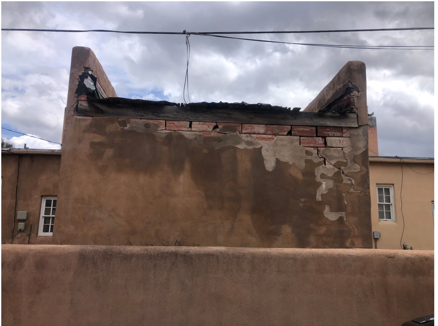
410 Don Gaspar Ave – Garage West Façade
