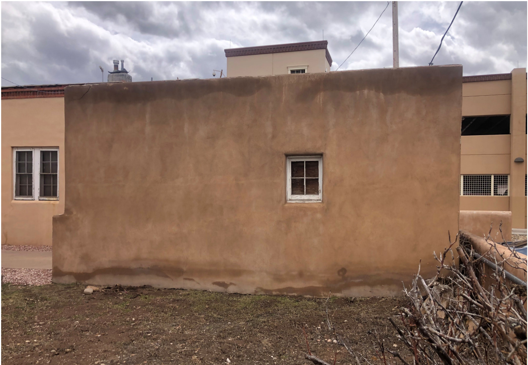
410 Don Gaspar Ave – Garage North Façade
