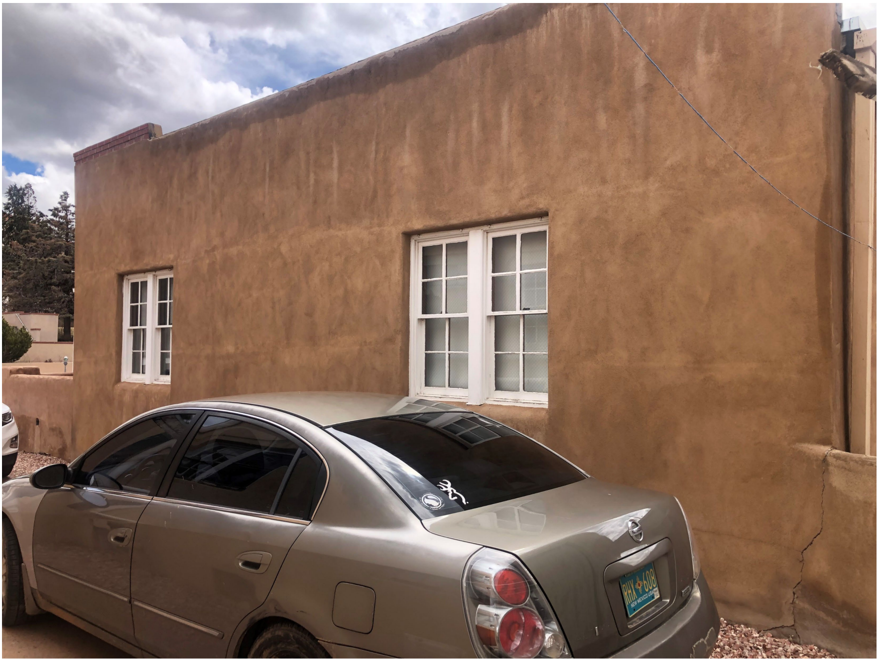
410 Don Gaspar Ave – North Façade
