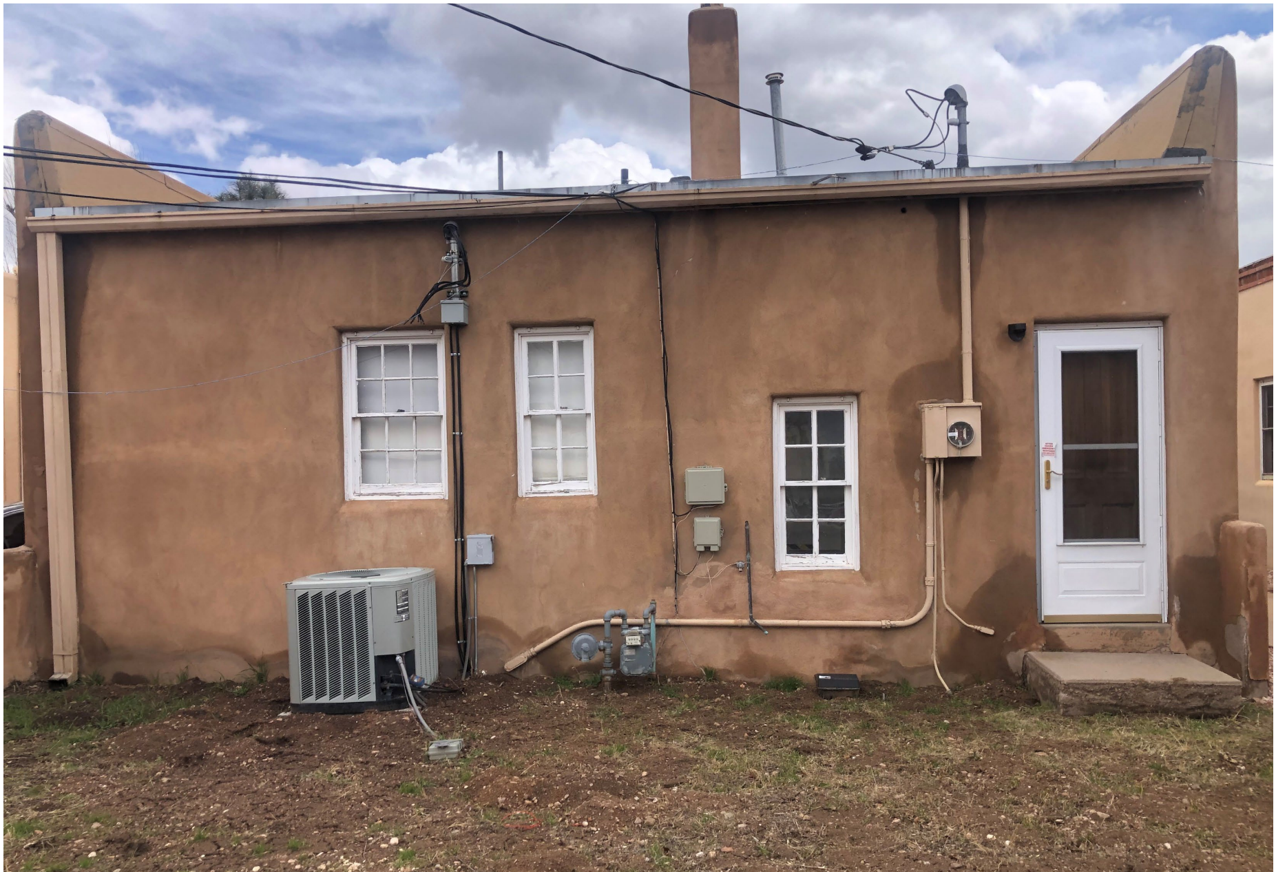
410 Don Gaspar Ave – West Facade
