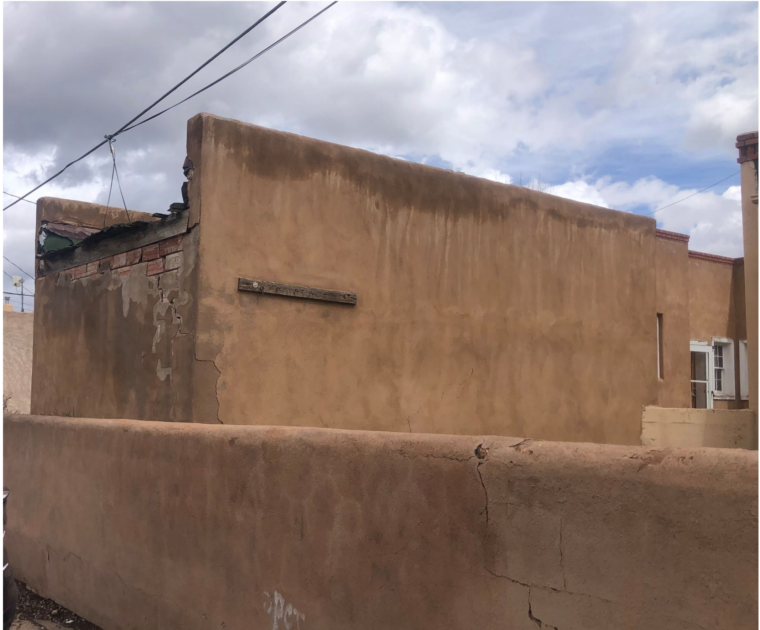
410 Don Gaspar Ave – Garage South Façade
