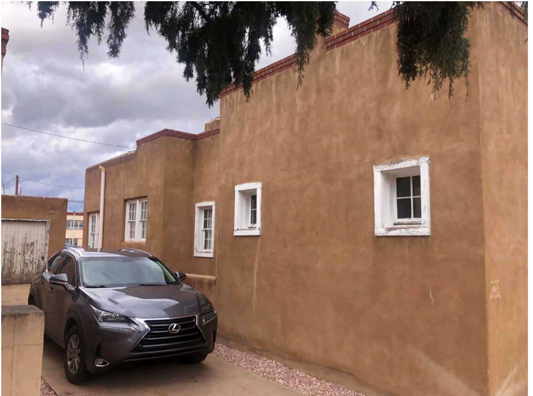
410 Don Gaspar Ave – South Facade
