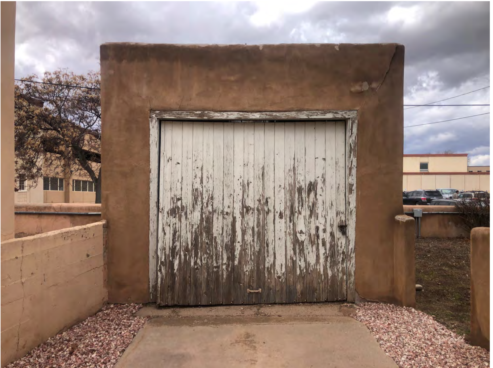
410 Don Gaspar Ave – Garage East Façade
