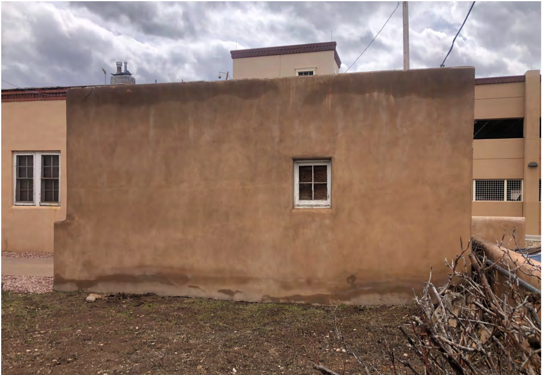
410 Don Gaspar Ave – Garage North Façade
