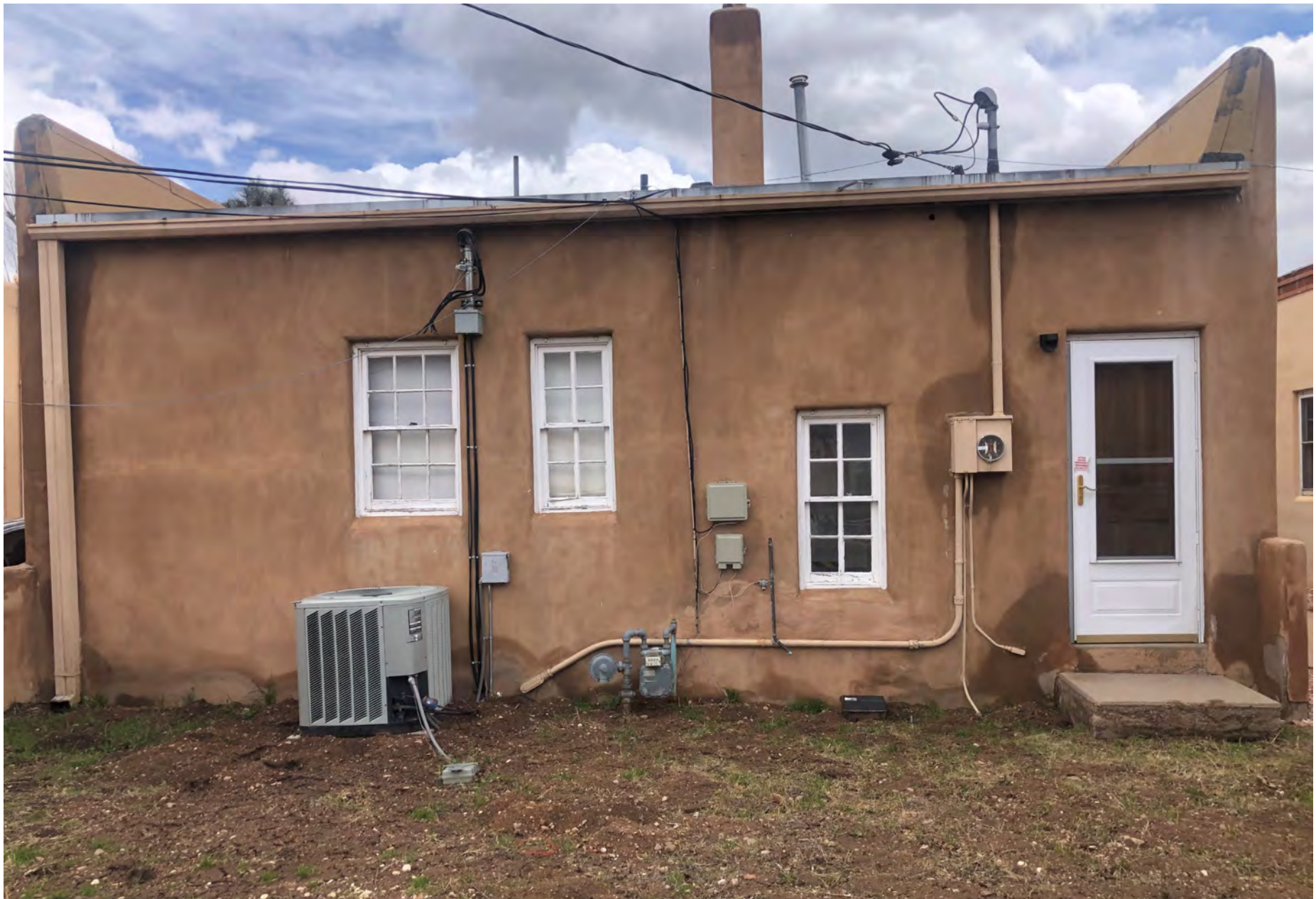
410 Don Gaspar Ave – West Facade
