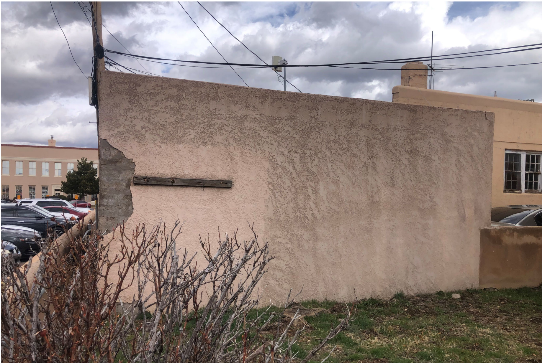
406 Don Gaspar Ave – Garage South Façade
