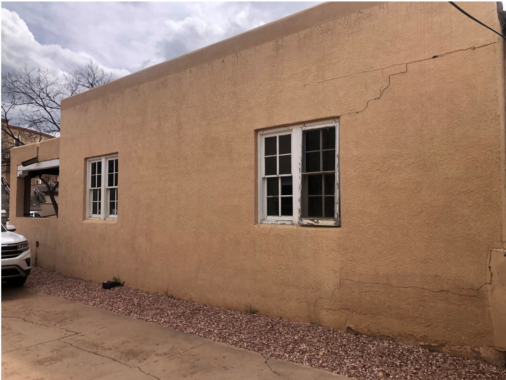
406 Don Gaspar Ave – North Façade
