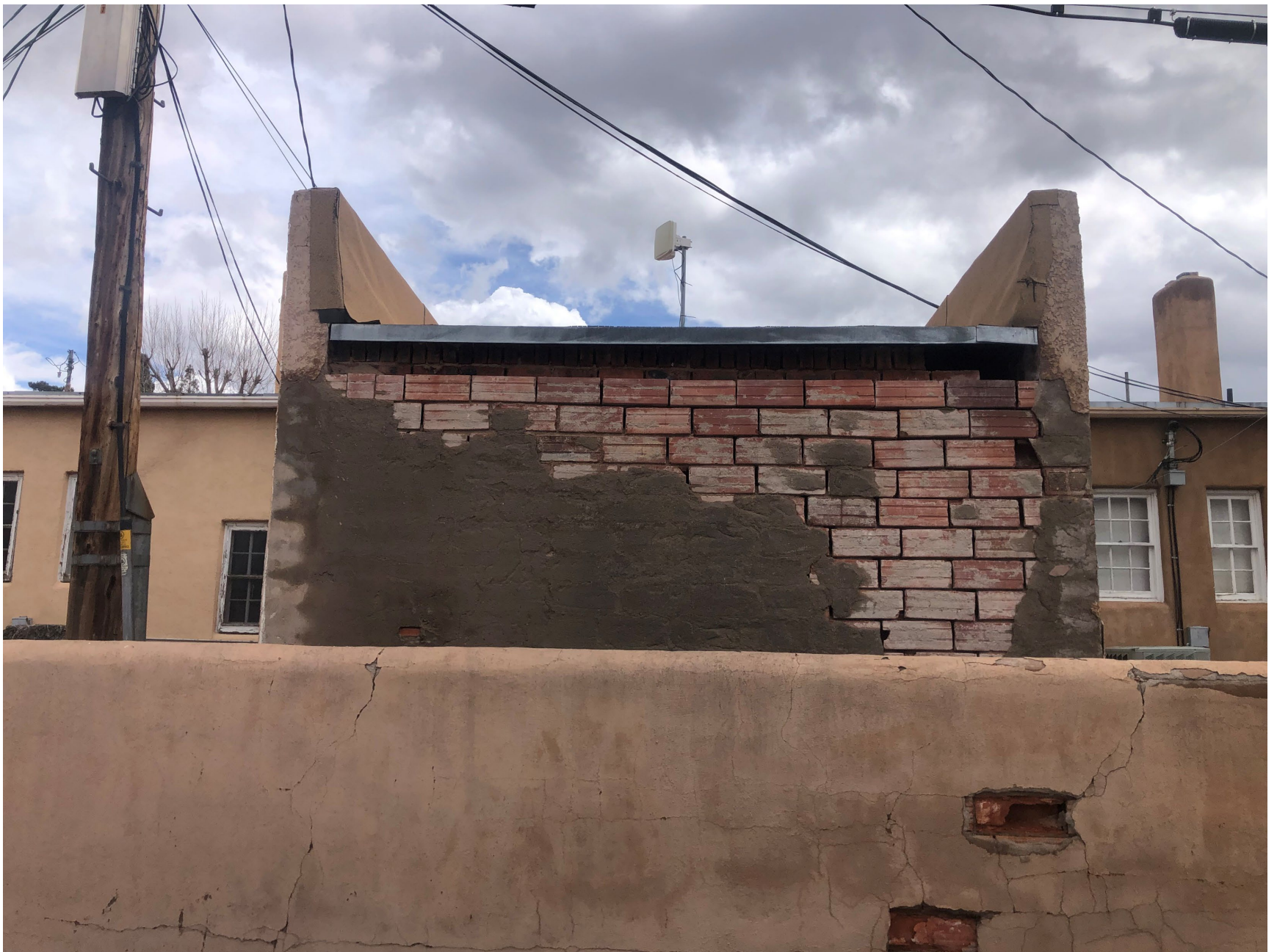
406 Don Gaspar Ave – Garage West Façade
