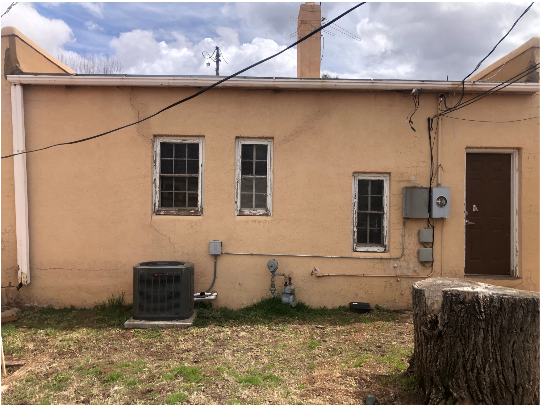
406 Don Gaspar Ave – West Facade
