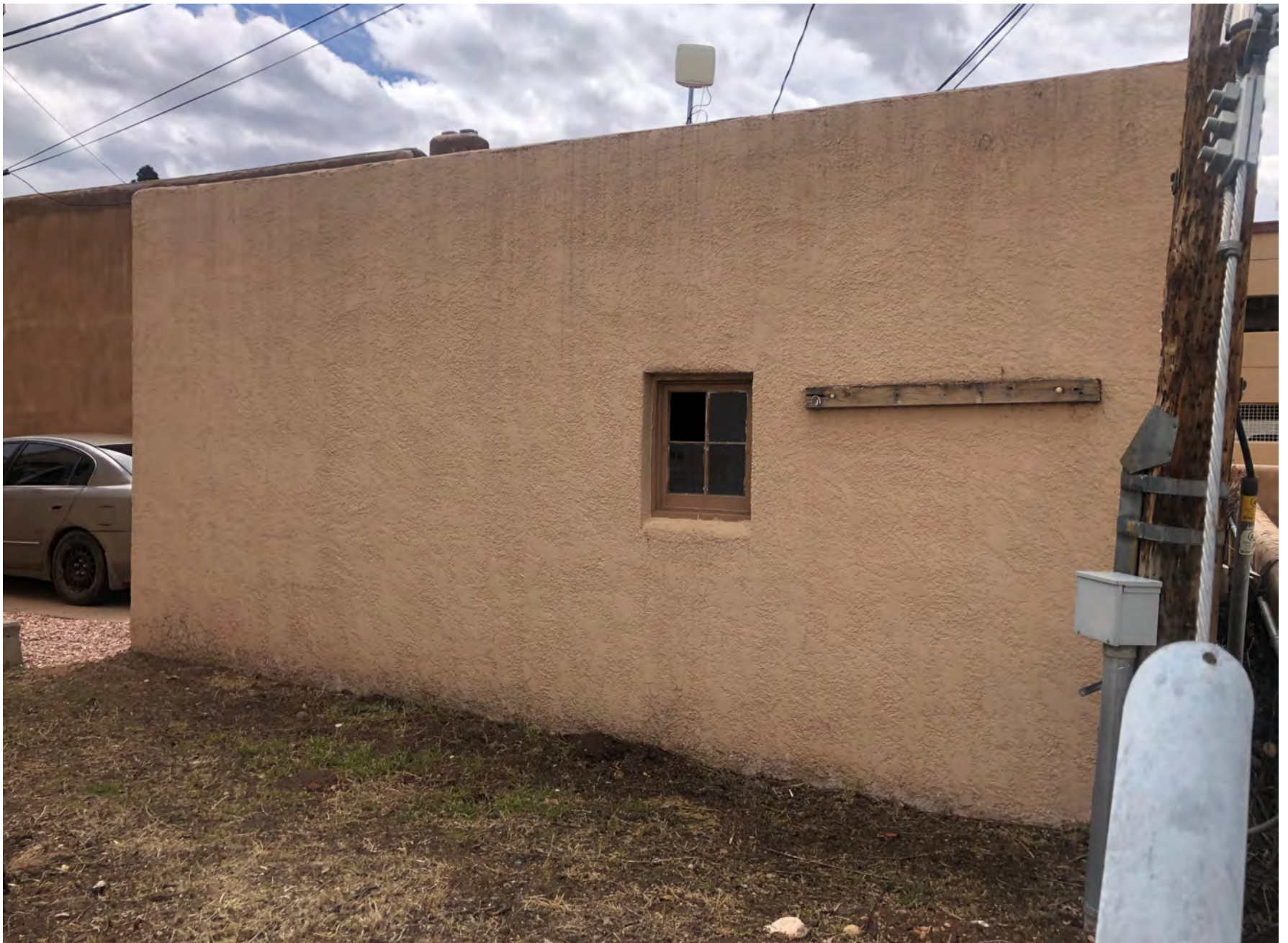
406 Don Gaspar Ave – Garage North Facade
