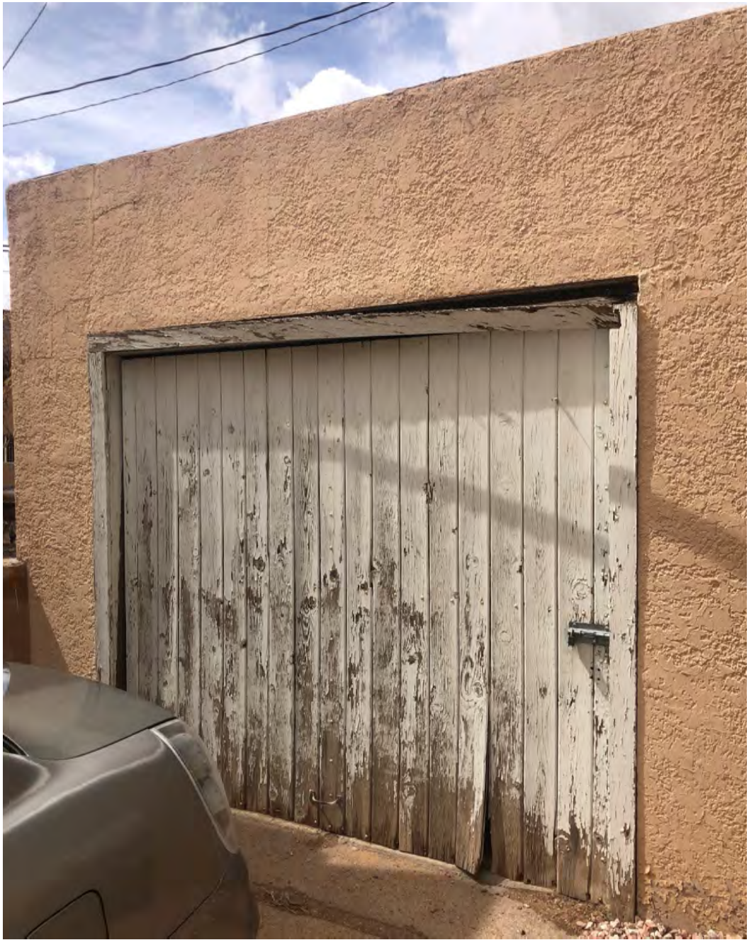
406 Don Gaspar Ave – Garage East Façade
