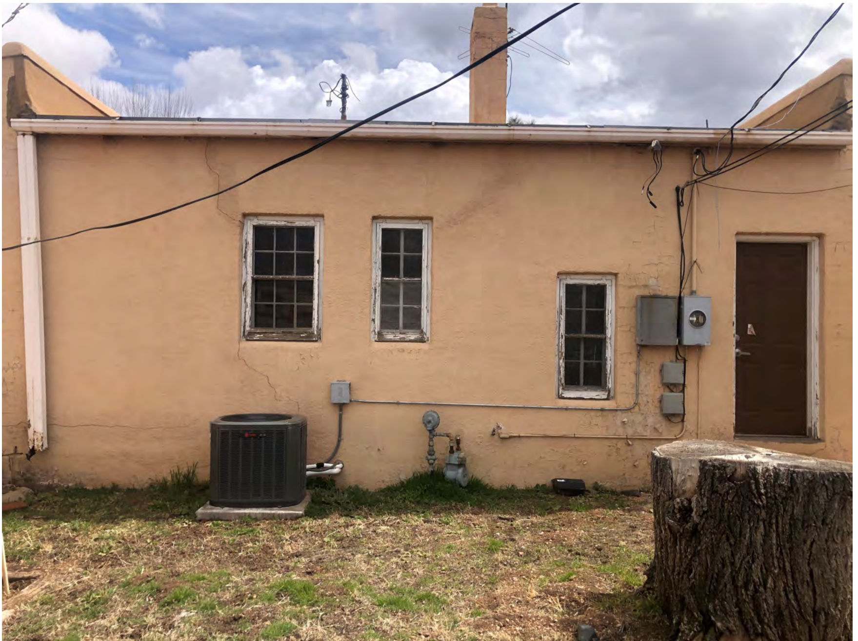
406 Don Gaspar Ave – West Facade
