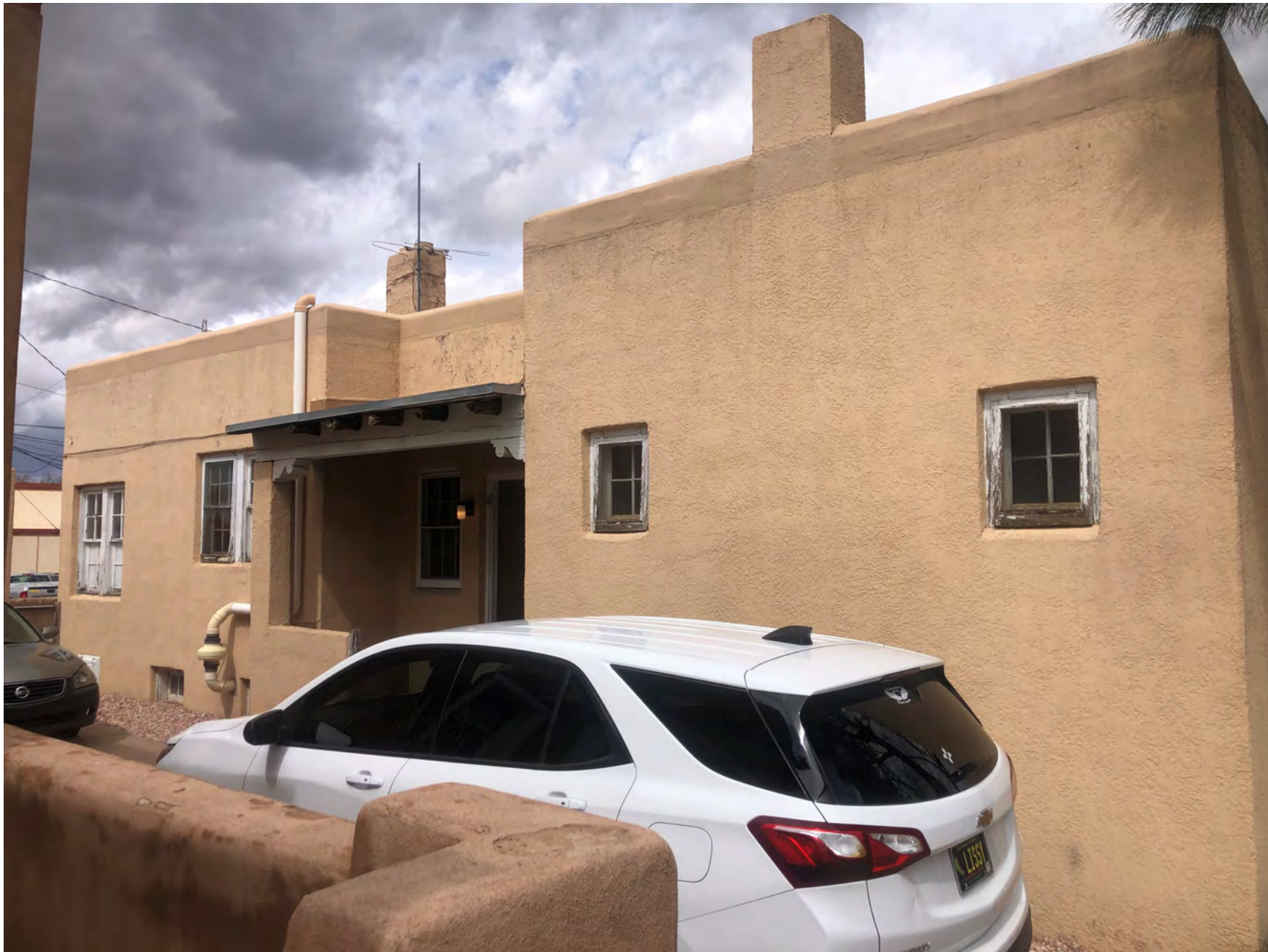
406 Don Gaspar Ave – South Facade
