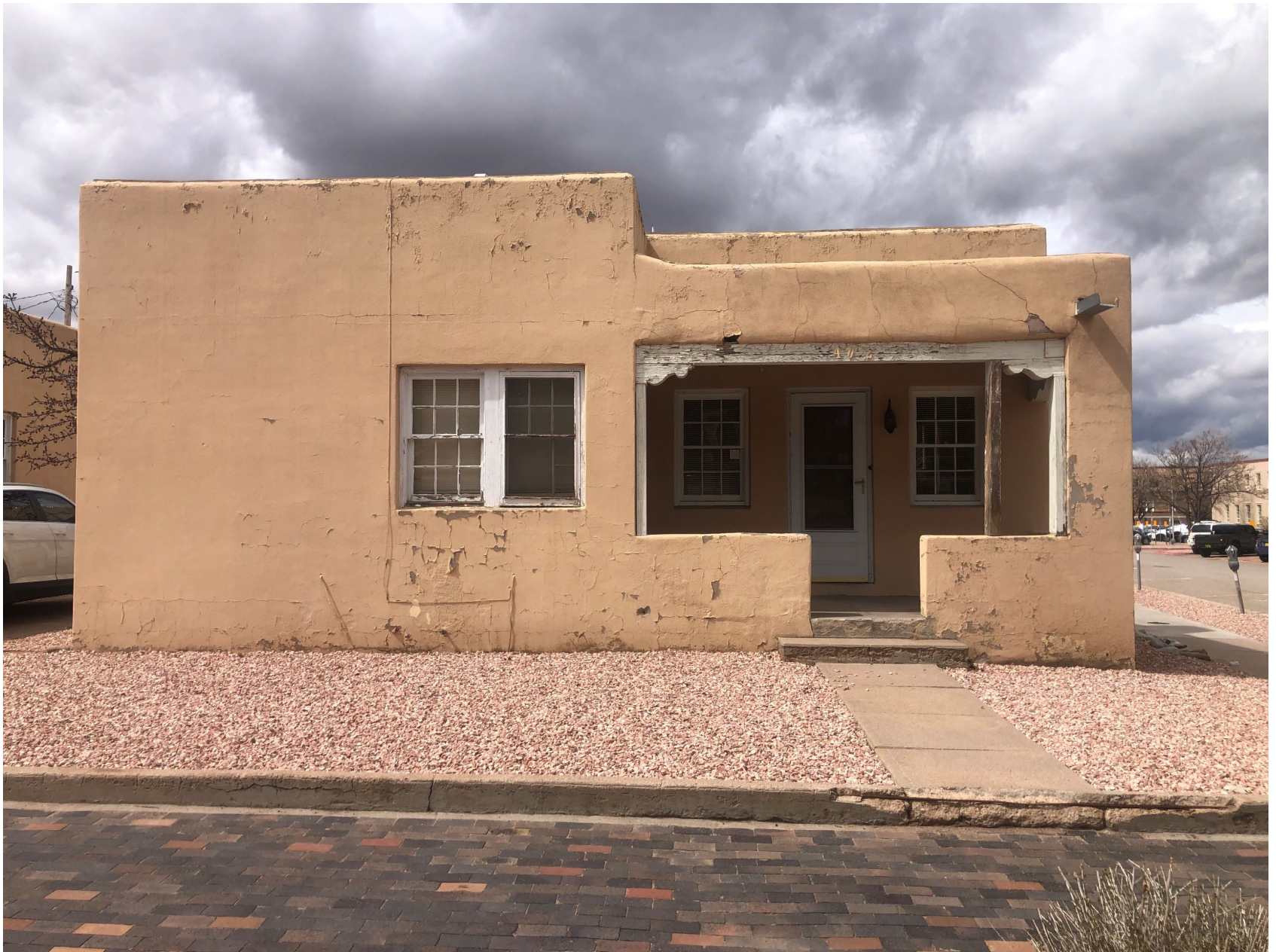
402 Don Gaspar Ave – East (Front) Façade
