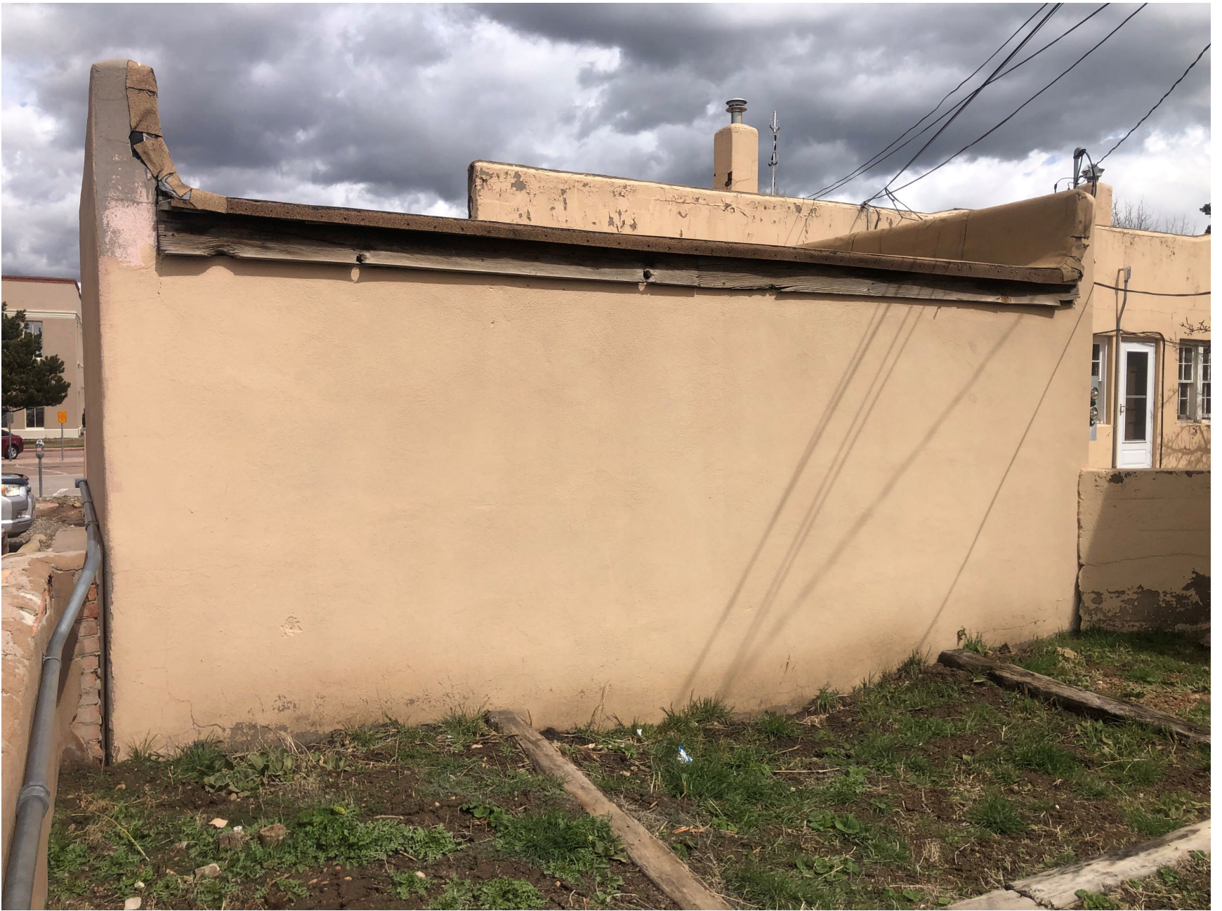
402 Don Gaspar Ave – Garage South Façade
