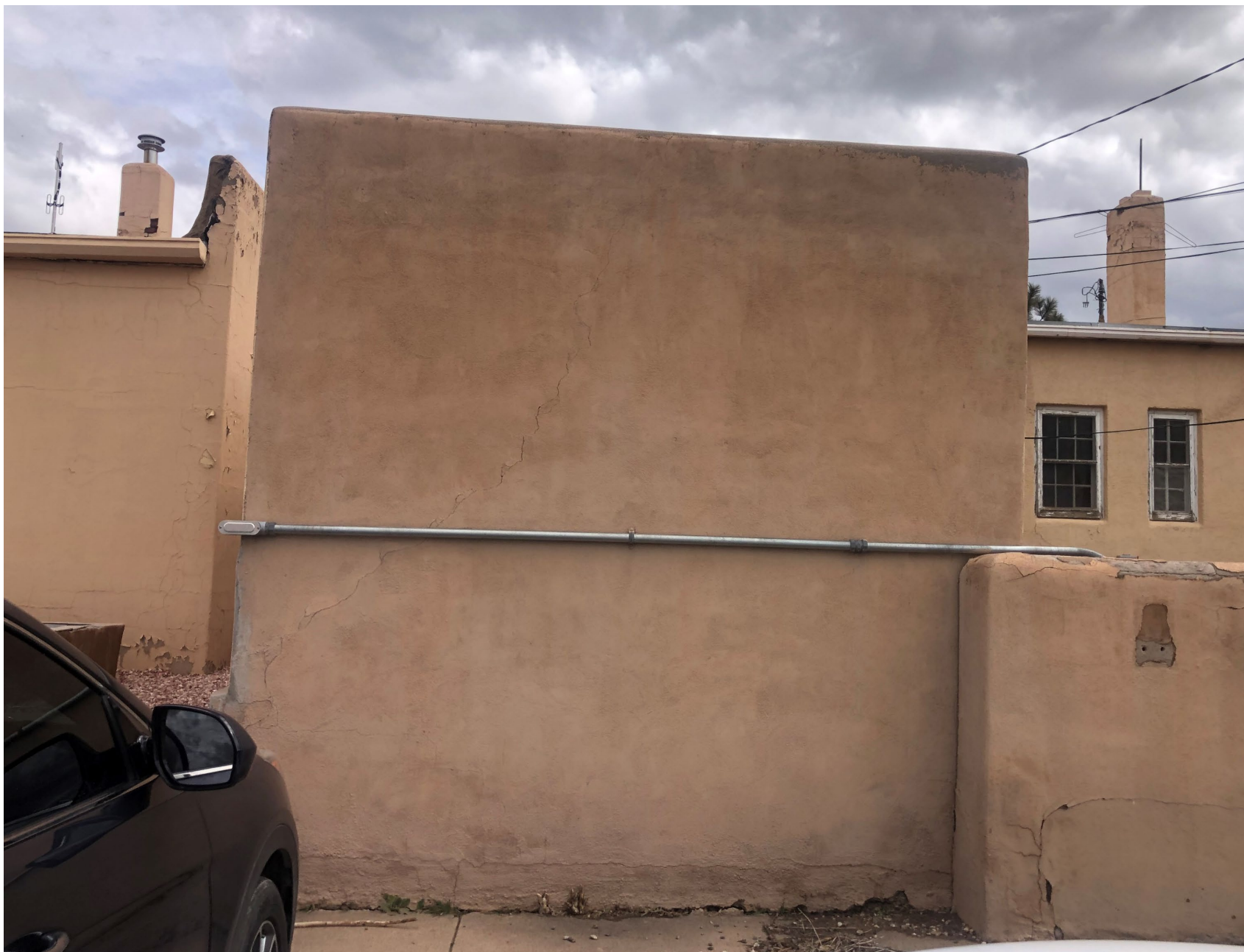
402 Don Gaspar Ave – Garage West Façade
