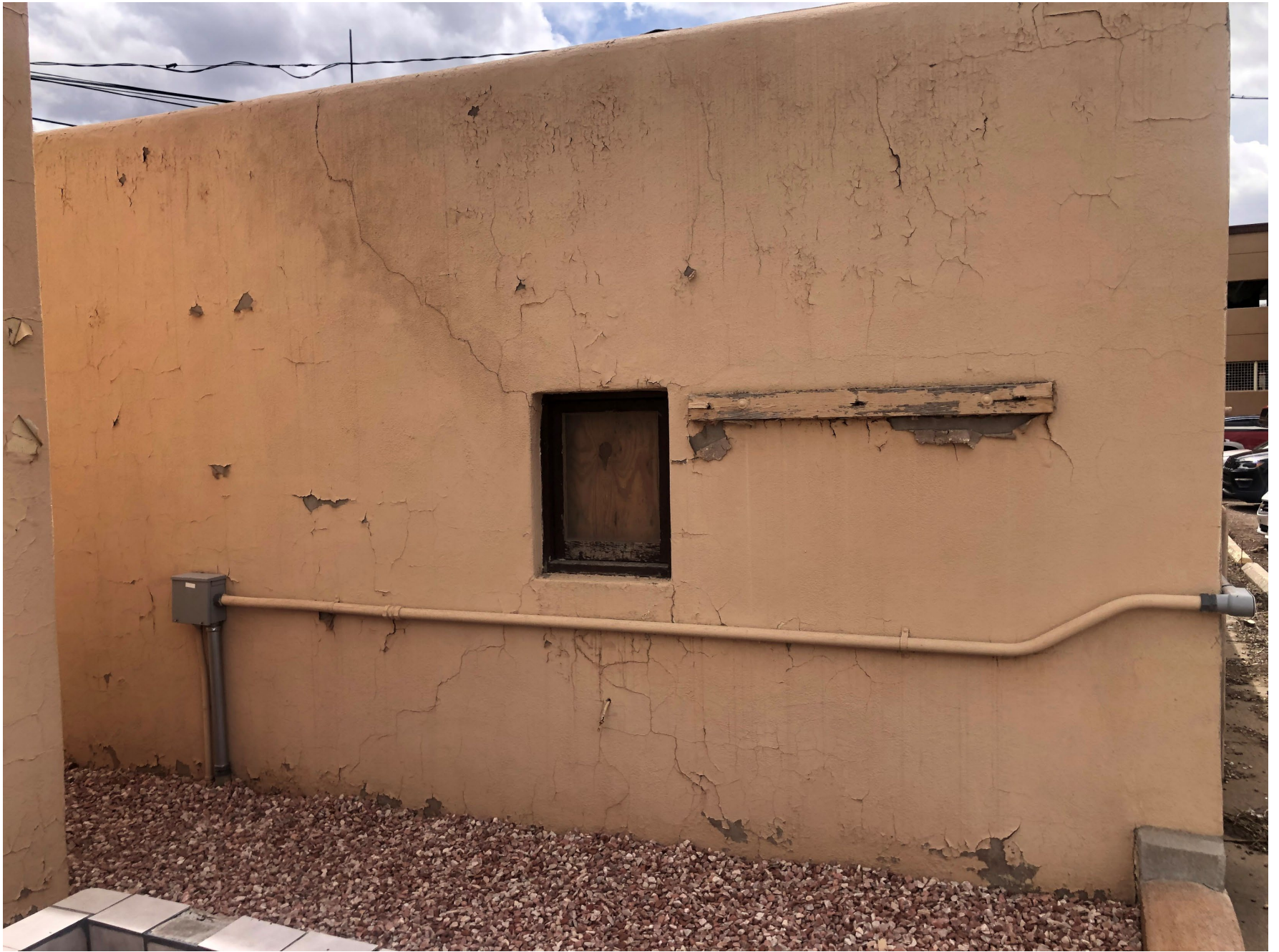
402 Don Gaspar Ave – Garage North Façade
