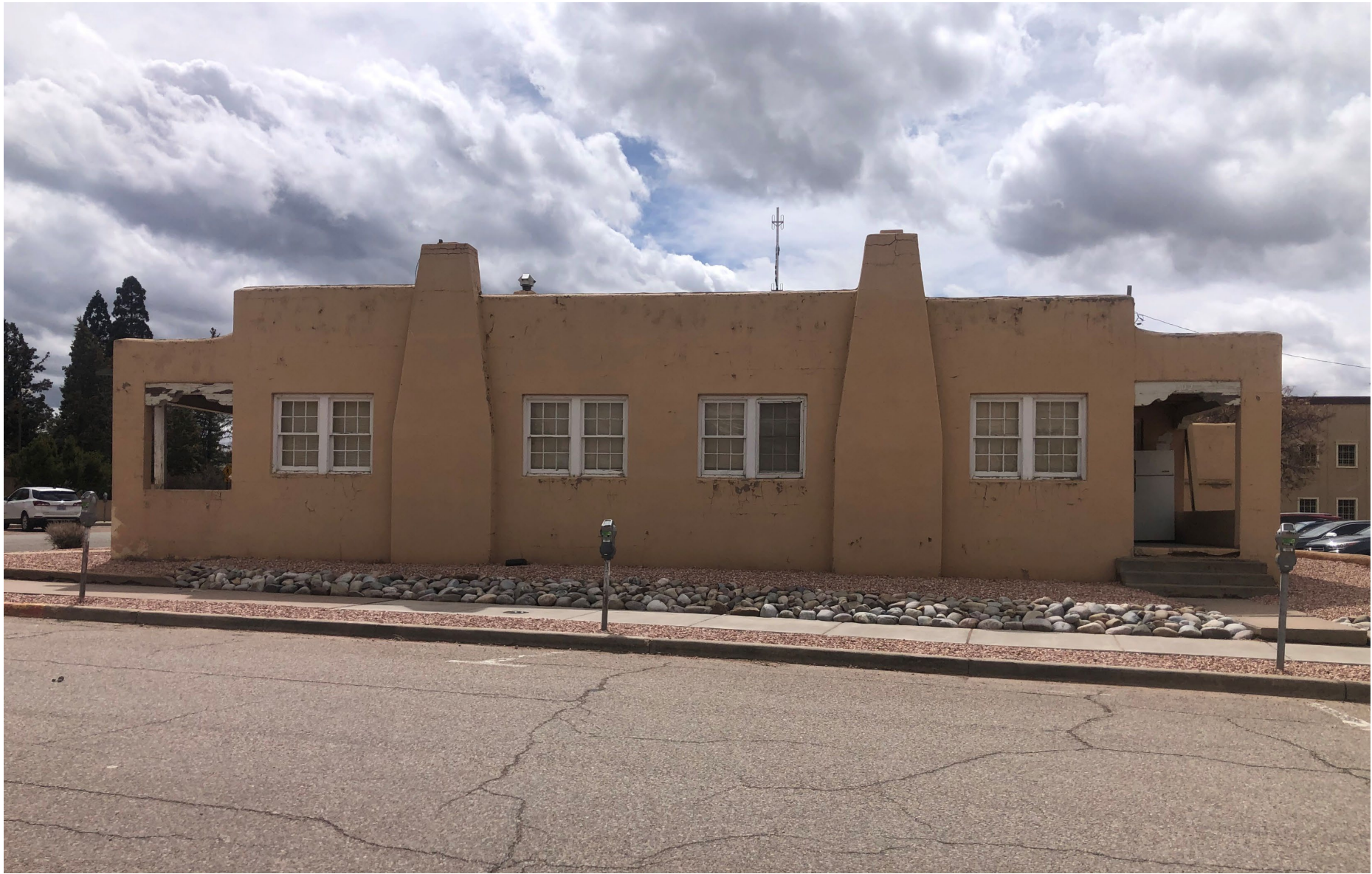
402 Don Gaspar Ave –North Façade
