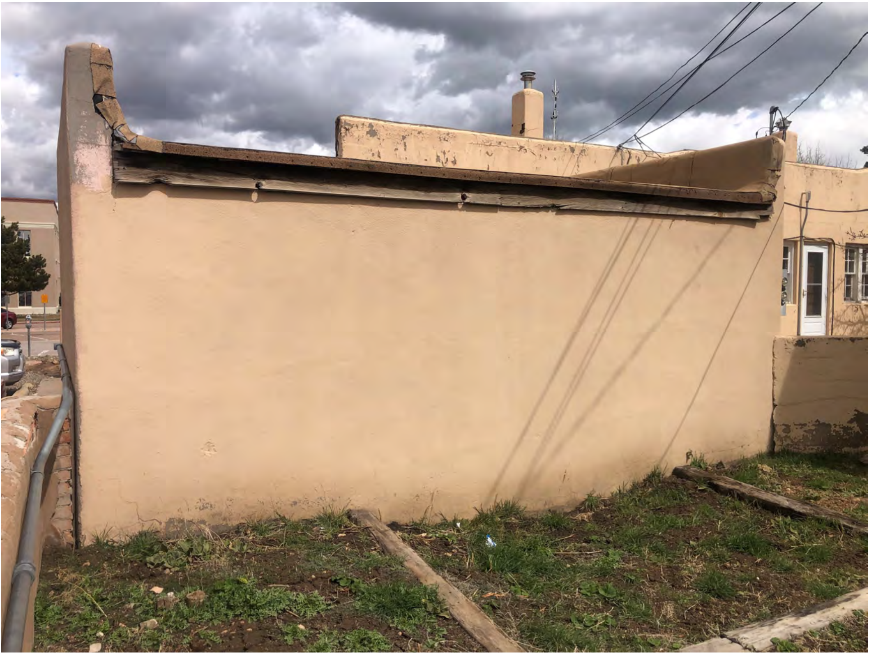
402 Don Gaspar Ave – Garage South Façade
