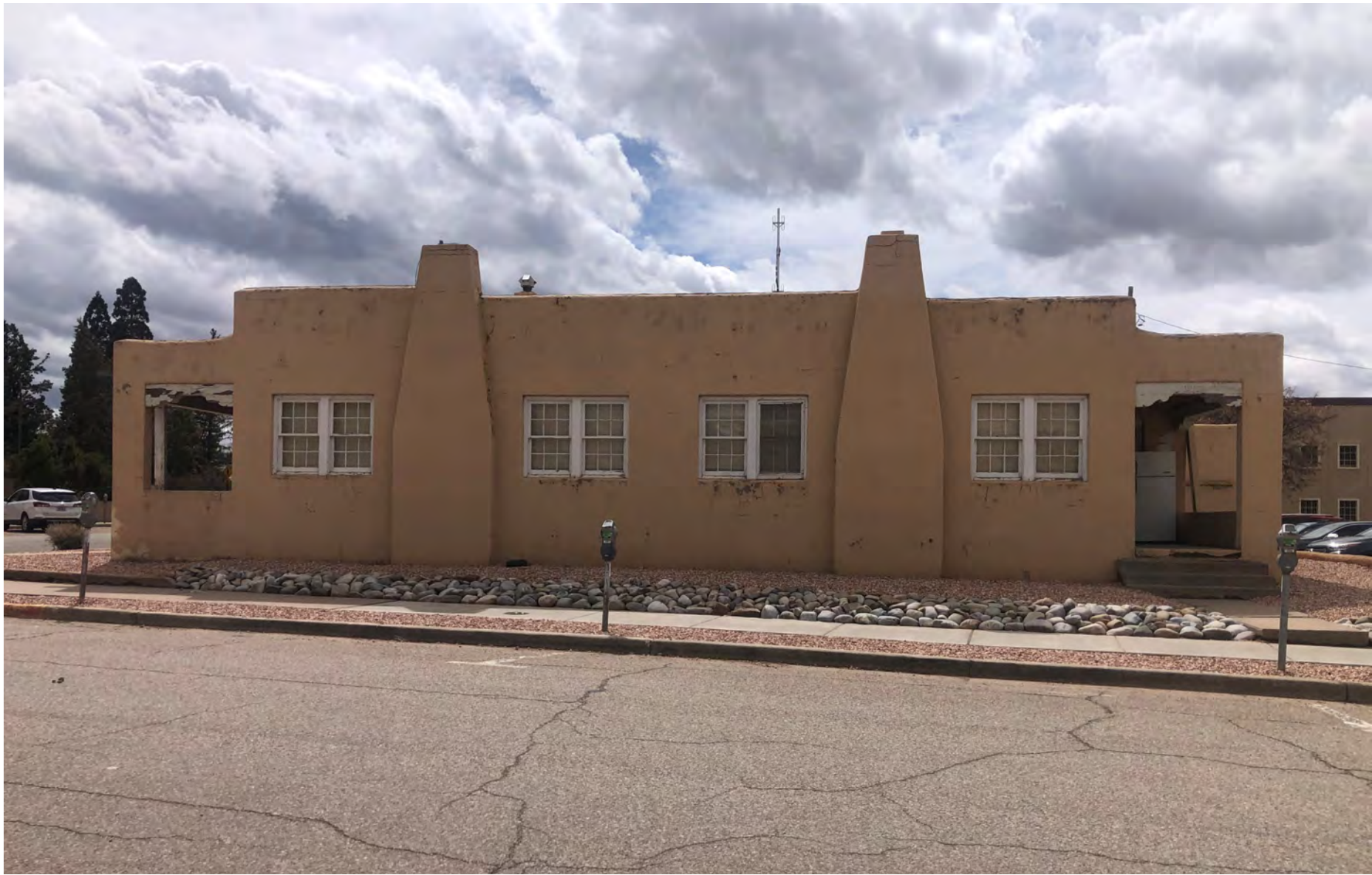
402 Don Gaspar Ave –North Façade
