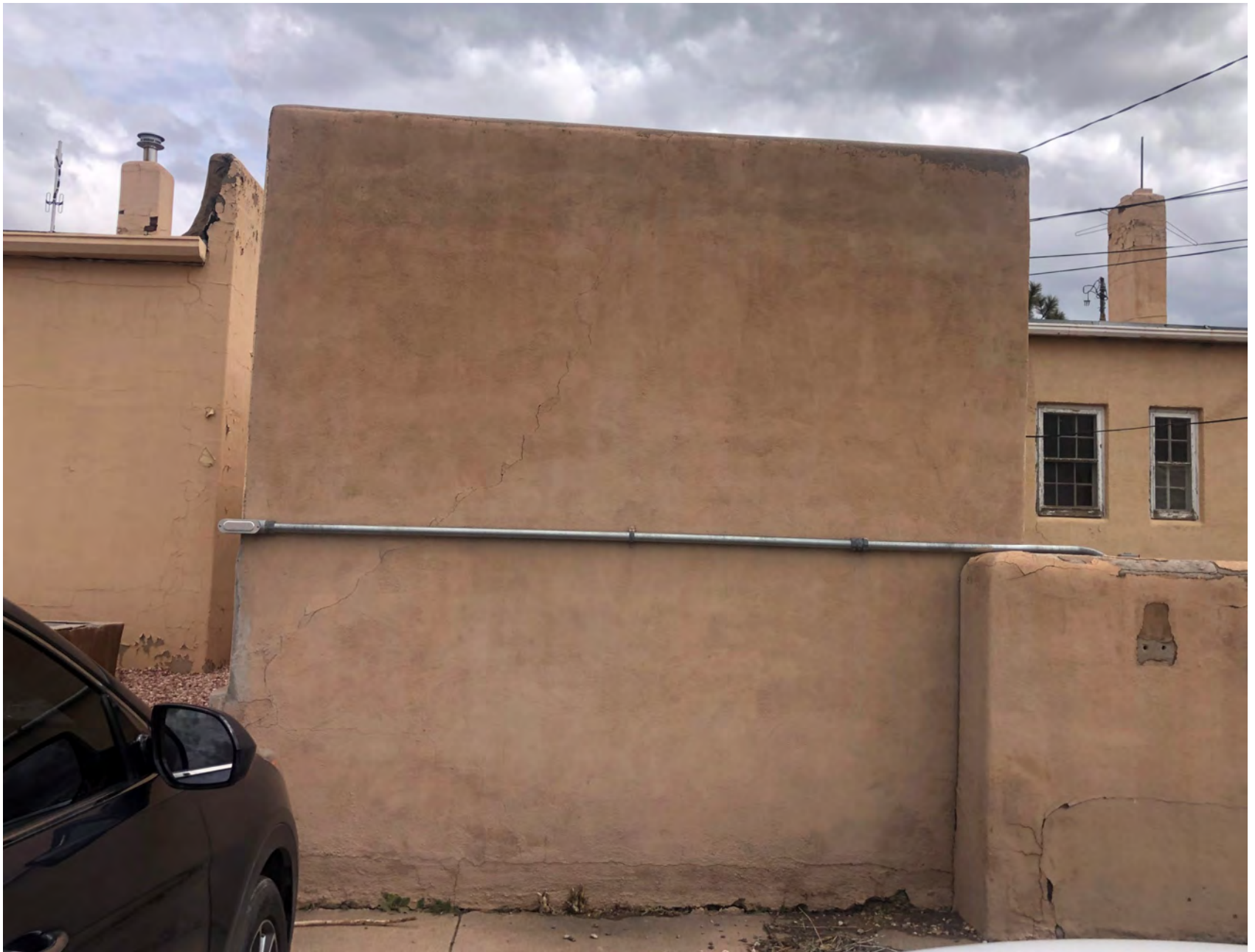
402 Don Gaspar Ave – Garage West Façade
