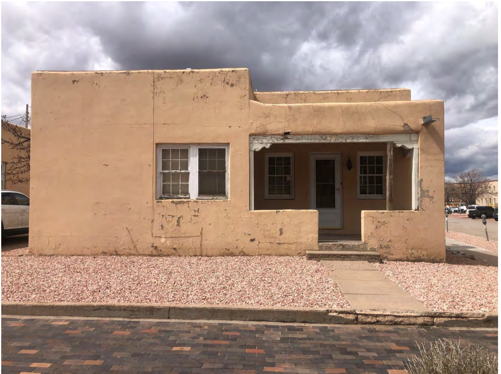
402 Don Gaspar Ave – East (Front) Façade
