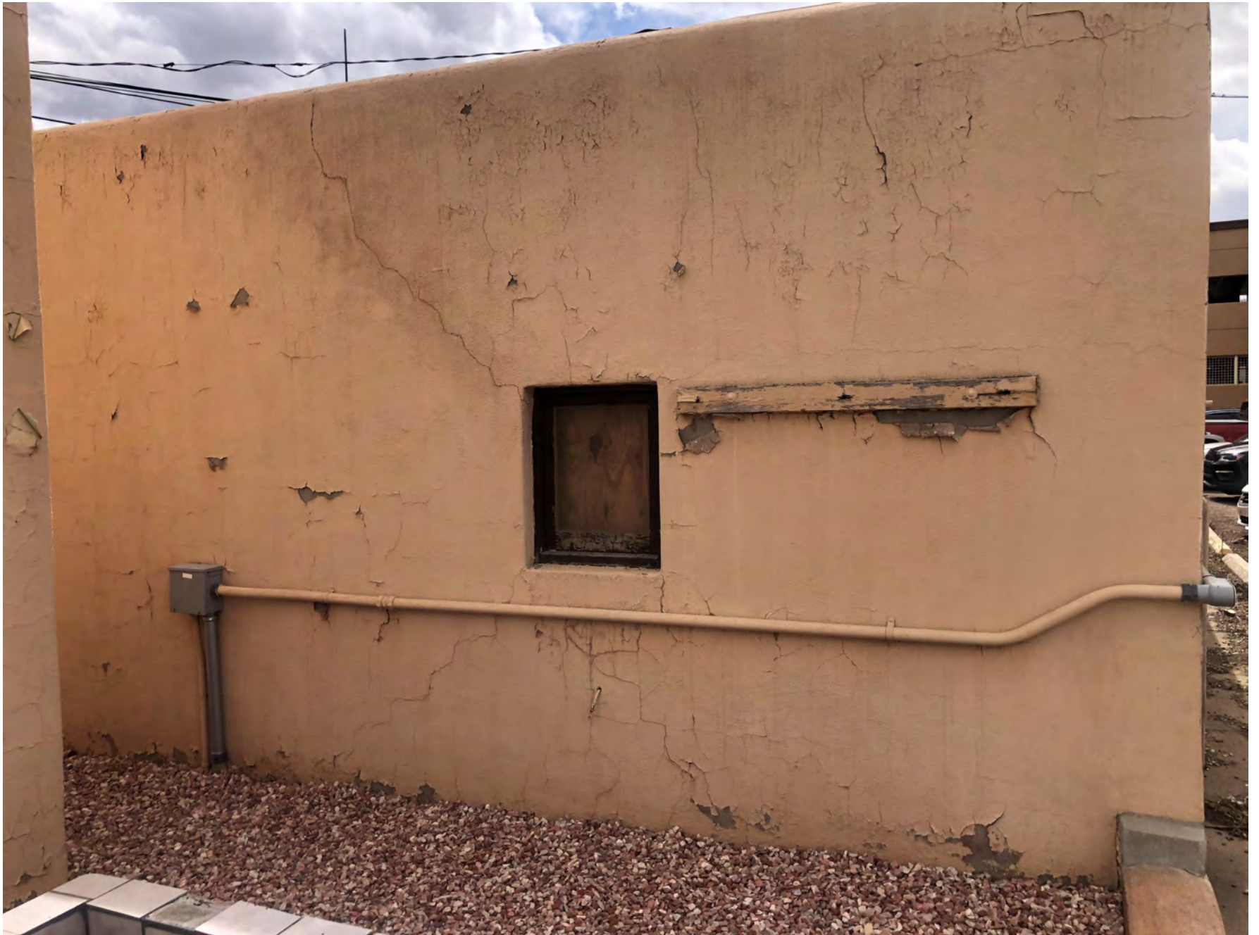
402 Don Gaspar Ave – Garage North Façade
