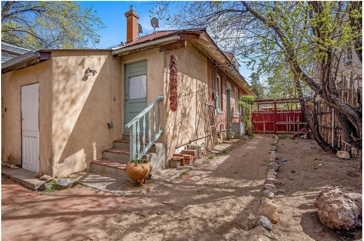
Figure 2: Addition in 2023, prior to demolition. Note attachment to original building's eaves. Addition was removed, roof repaired, and construction of a new addition that is 42 square feet larger (through the squaring off of the addition at the original entryway) than the historic addition.
