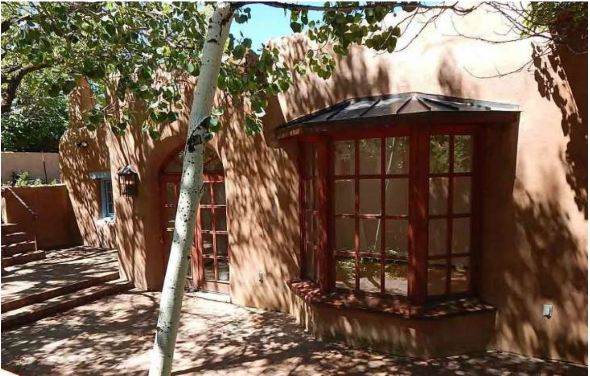
Figure 3. East Facade III.
