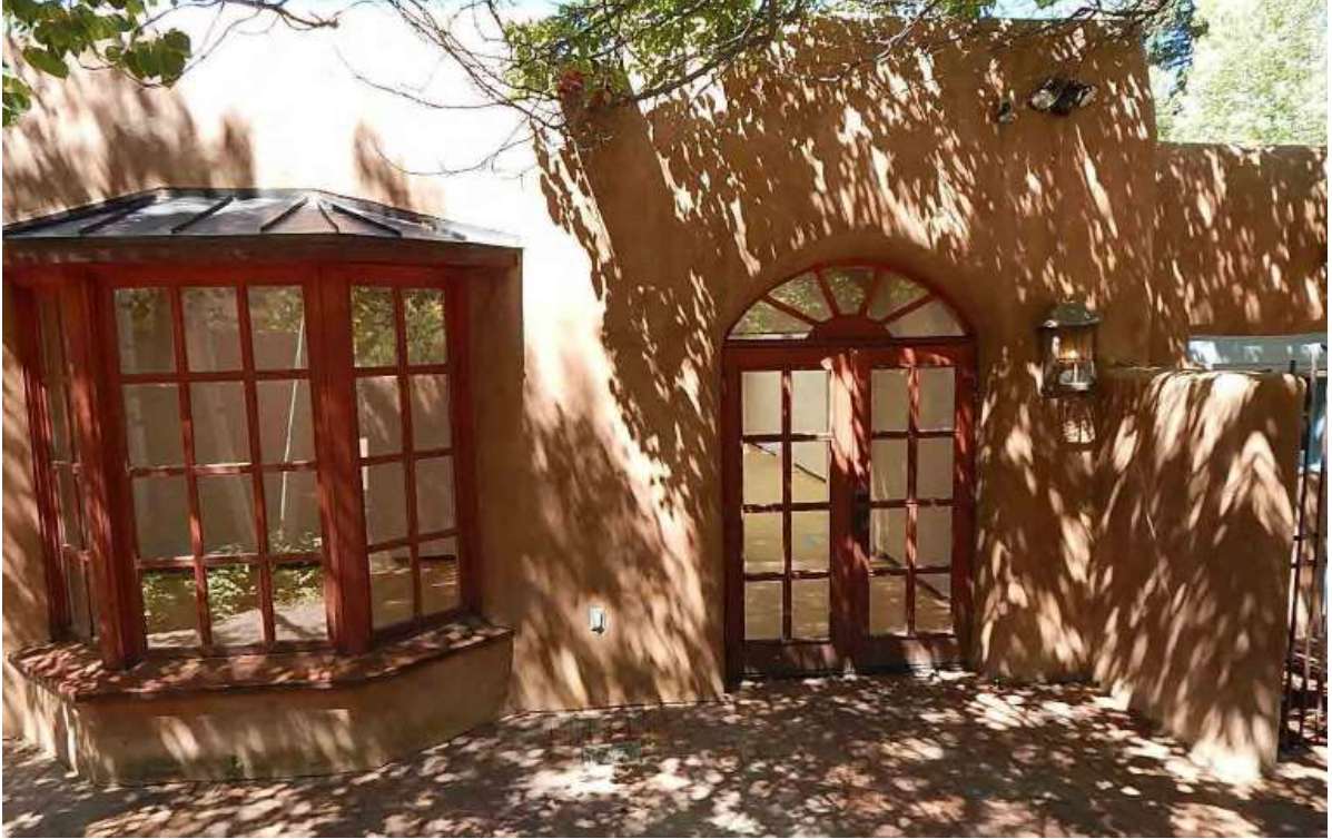
Figure 2. East Facade II.
