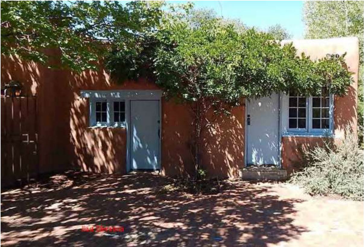
Figure 1. East Facade I.
