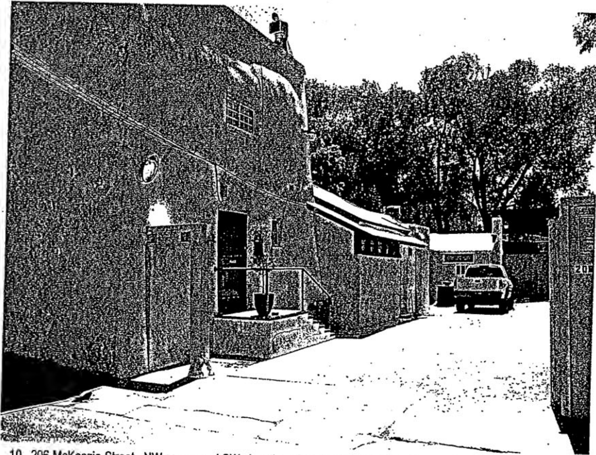
10. 206 McKenzie Street. NW corner and SW elevation of building indicates similar massing as seen in a 1995 photograph. View SE. (ArcCom September 2, 2005).
