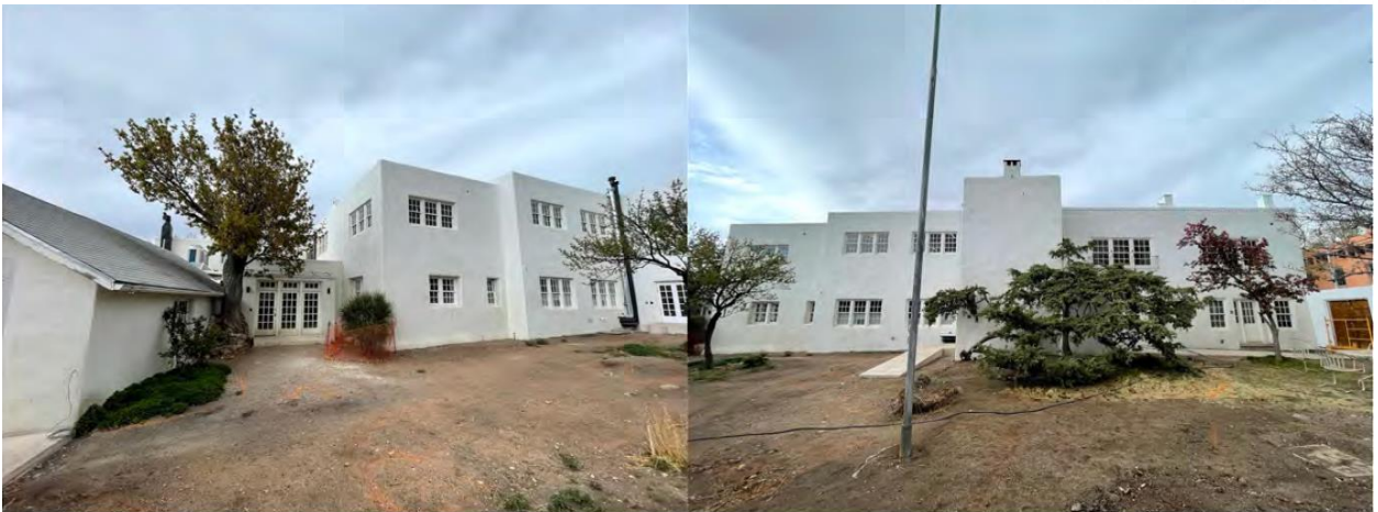
(Left side of South Elevation)
