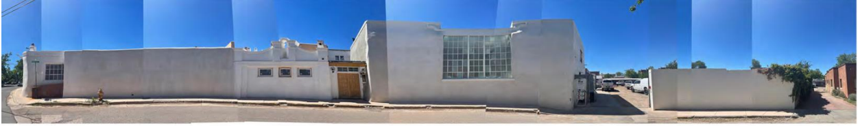
206 McKenzie Street McKenzie Street / North Elevation
