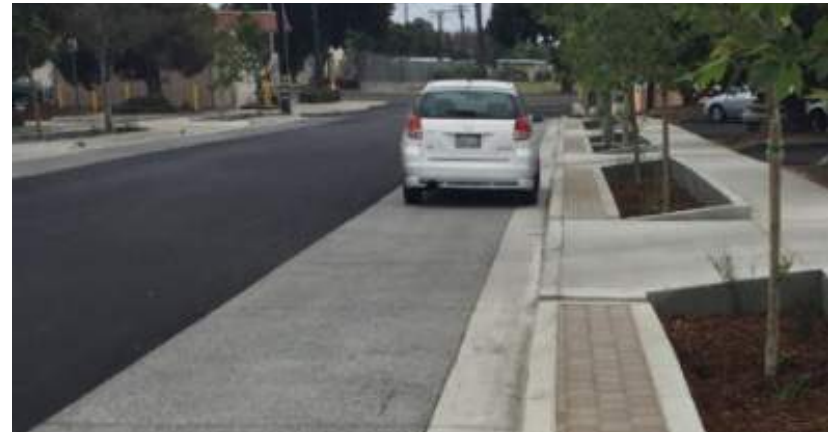
Permeable parking aisles reduce runoff, enhance infiltration
