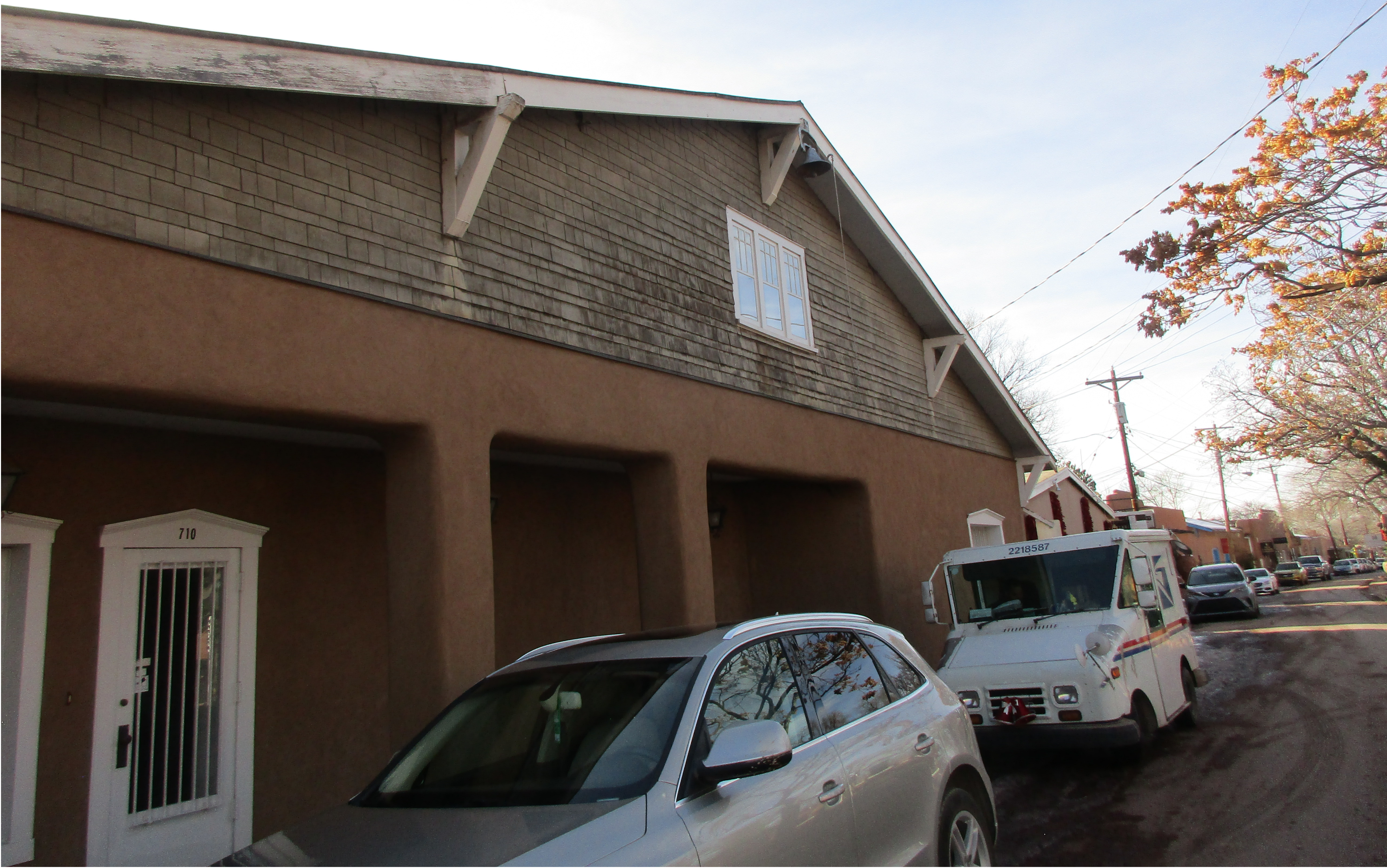
710 Canyon Rd - Street View North Elevation
