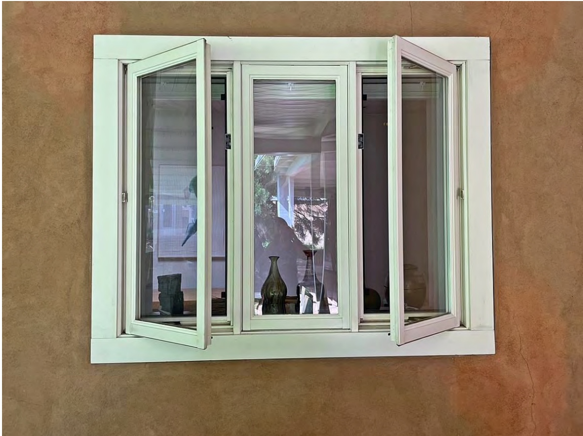
Photo 12: Wing. East elevation. Fenestration. Camera facing west.
