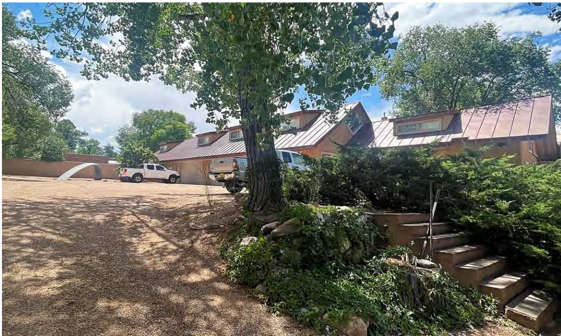
Photo 2: 1980s Back Building. Camera facing southwest.
