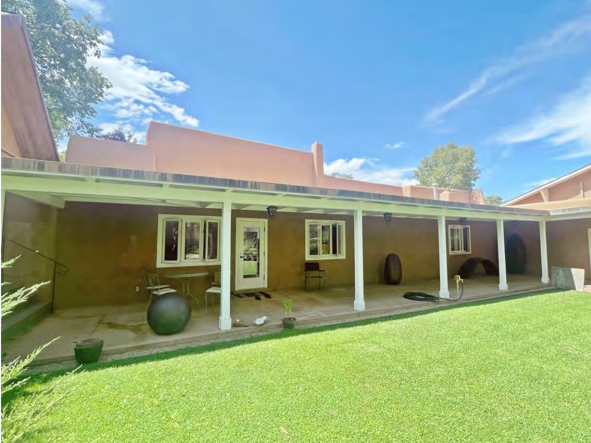
Photo 11: Wing. East elevation. Camera facing northwest.
