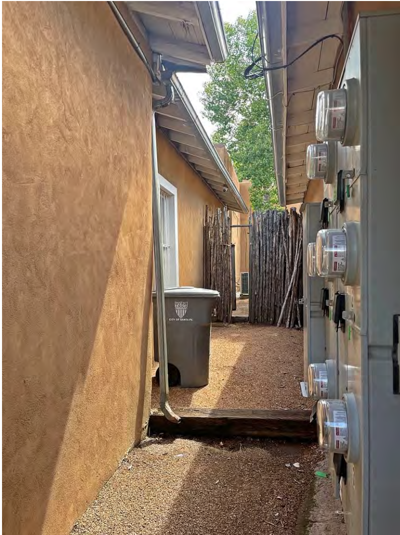
Photo 9: West elevation. Camera facing south.
