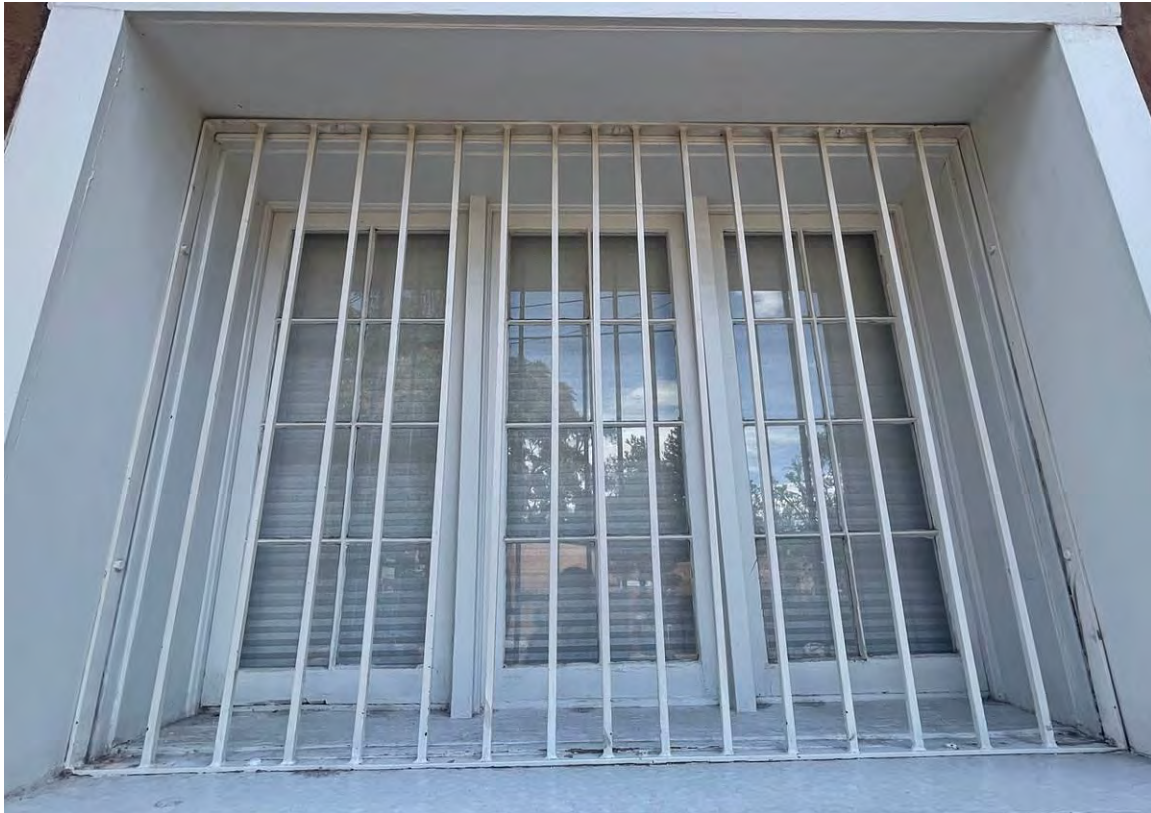
Photo 4: North elevation. West window. Camera facing up.
