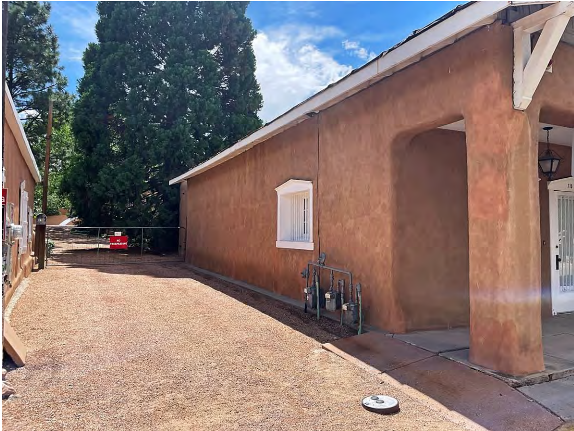
Photo 6: East elevation. Camera facing southwest.
