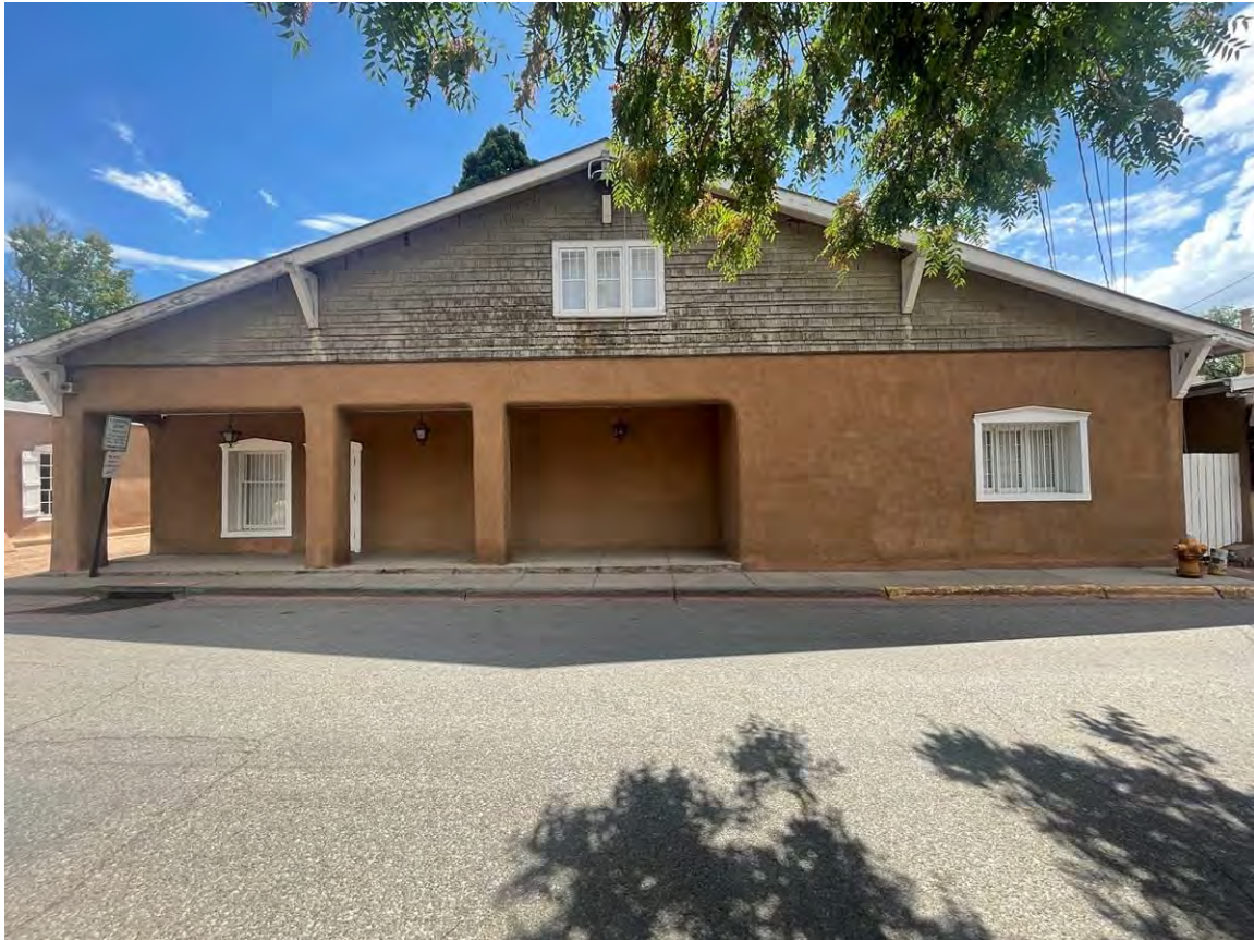
Photo 3: Front Building. North façade. Camera facing south.
