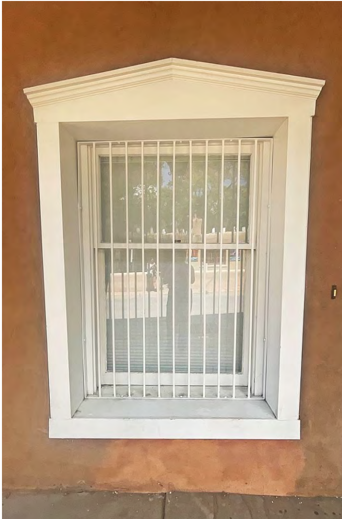
Photo 5: North elevation. East window. Camera facing south.
