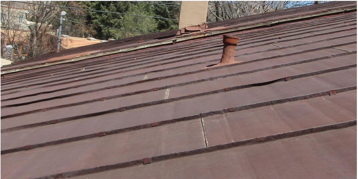
Existing Roof Material
