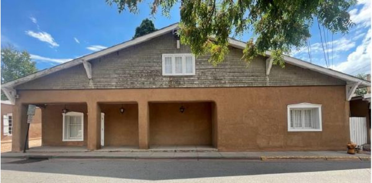
Figure 1: North Street Facing Elevation: Primary Facade
