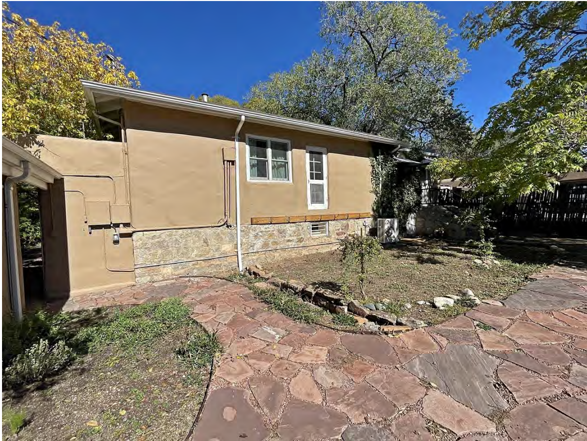
Photo 9: South elevation. Camera facing northeast.
