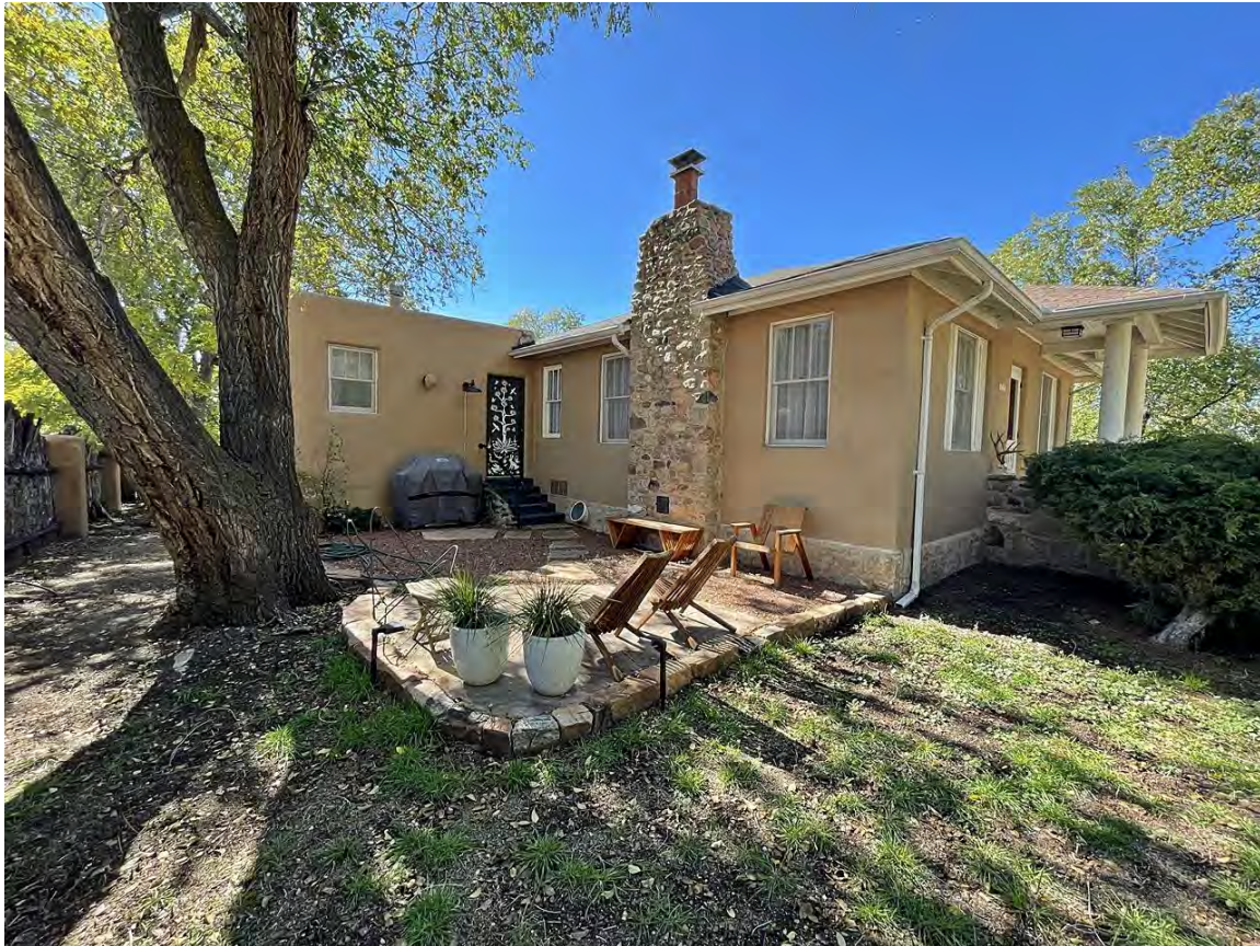
Photo 13: East elevation. Camera facing southwest.
