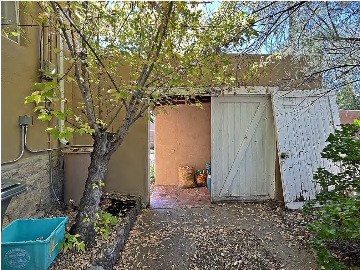
Photo 14: Former garage, north elevation. Camera facing south.
