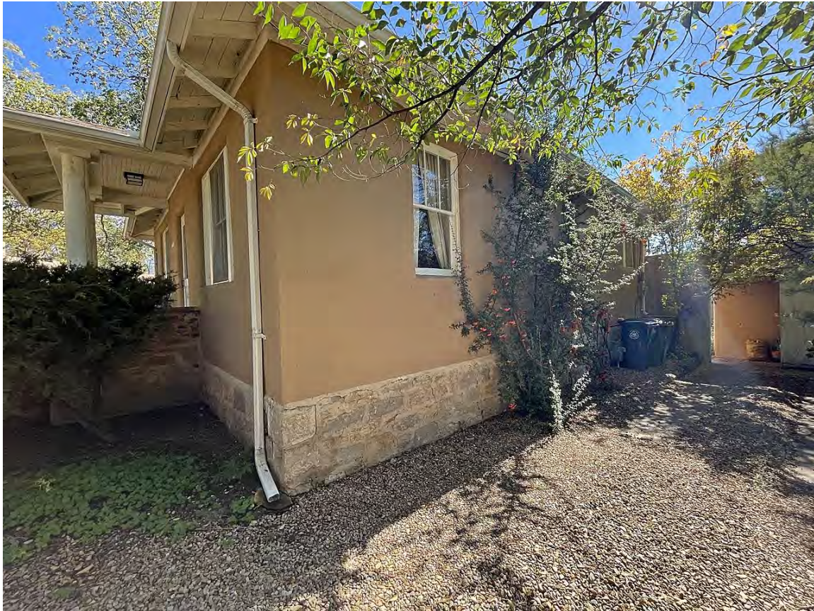
Photo 7: Northwest corner. Camera facing southeast.
