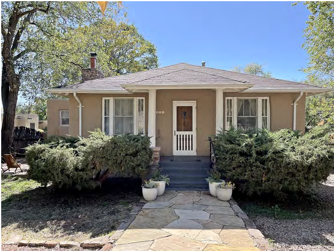
Photo 1: Front (north) façade. Camera facing south.
