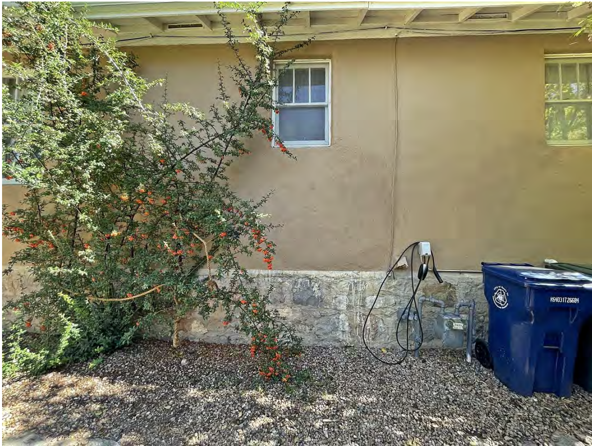
Photo 8: Partial west elevation. Camera facing east.
