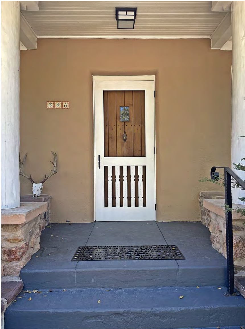
Photo 4: North façade, detail of front door. Camera facing south.
