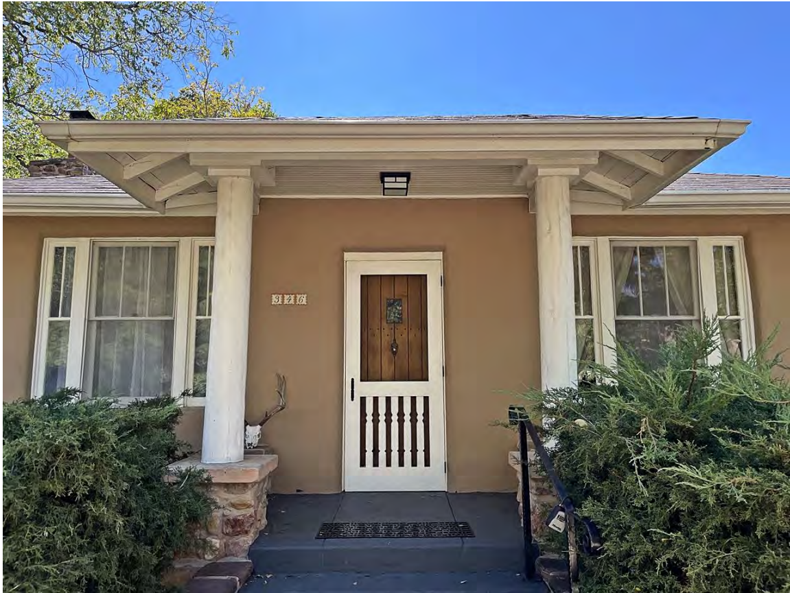
Photo 3: North façade entry. Camera facing south.
