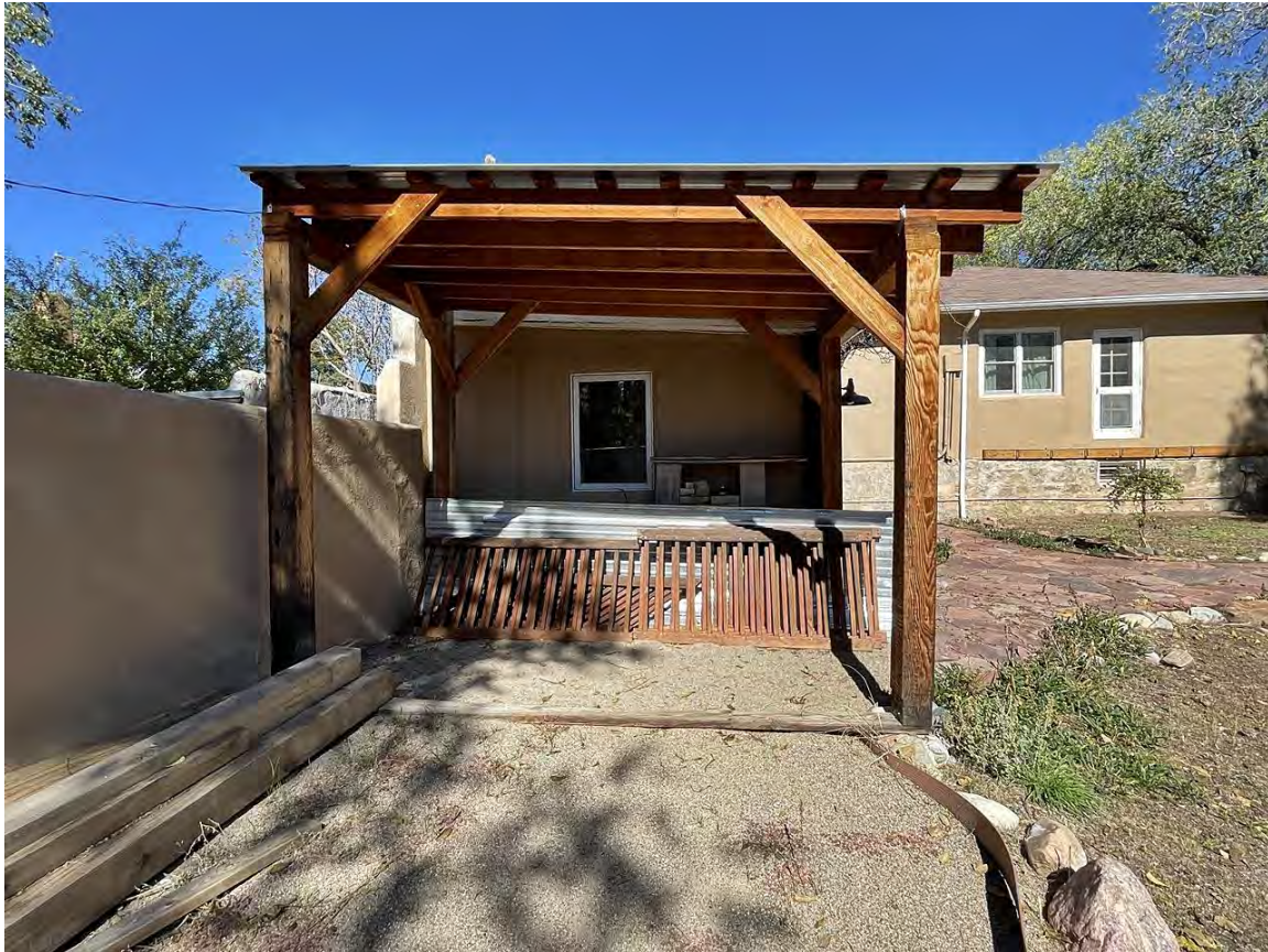
Photo 17: Studio, south elevation. Camera facing north.
