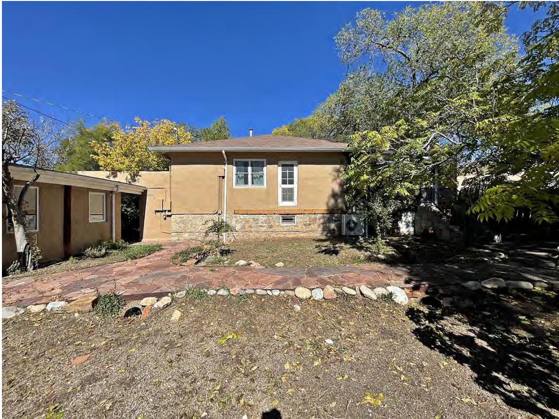
Photo 15: House and Studio. Camera facing north.
