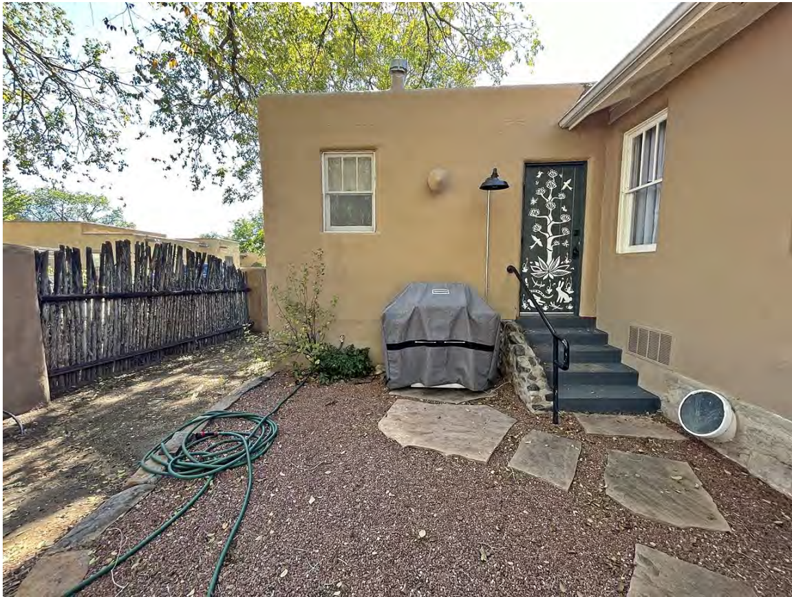
Photo 12: Addition, north elevation. Camera facing south.
