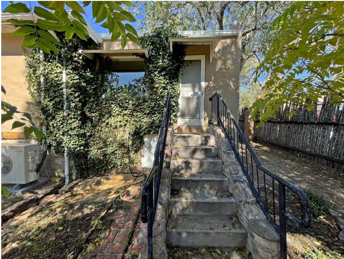
Photo 10: Addition, south elevation. Camera facing north.
