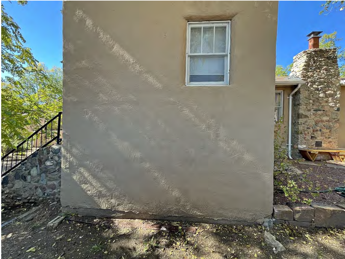
Photo 11: Addition, east elevation. Camera facing west.
