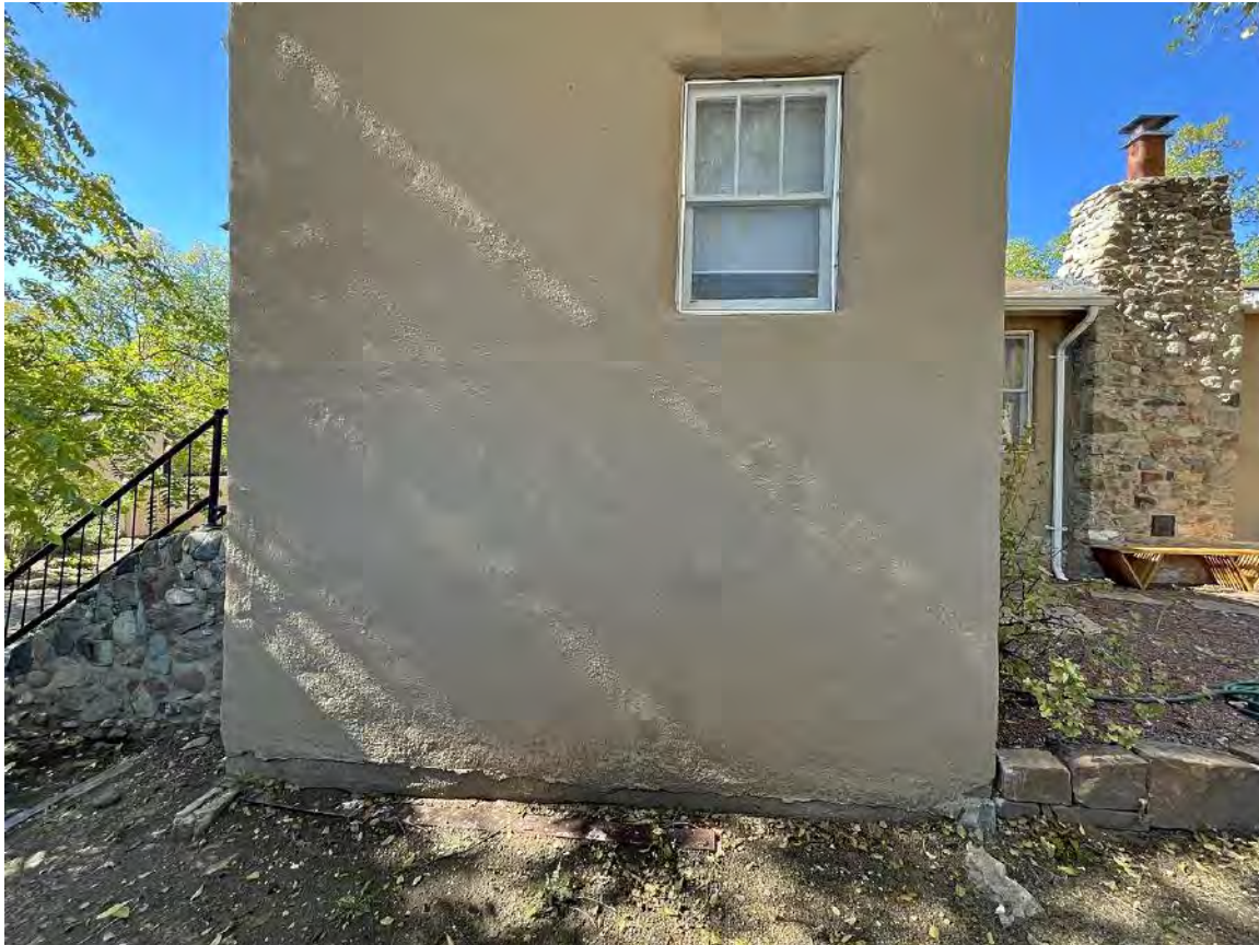
Photo 11: Addition, east elevation. Camera facing west.
