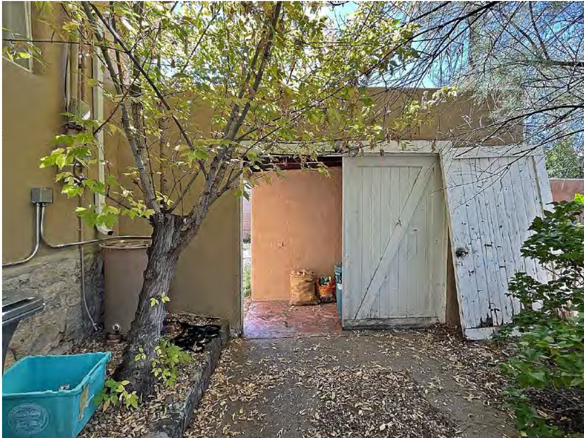
Photo 14: Former garage, north elevation. Camera facing south.
