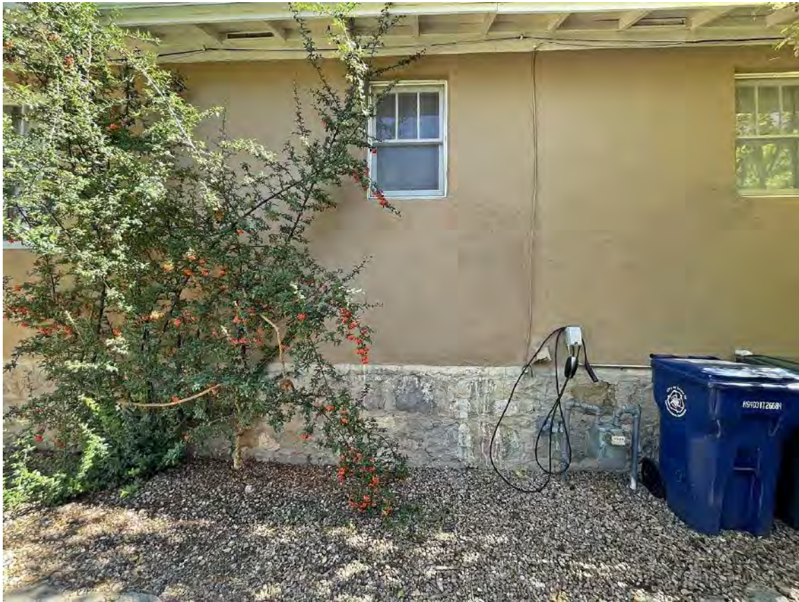
Photo 8: Partial west elevation. Camera facing east.
