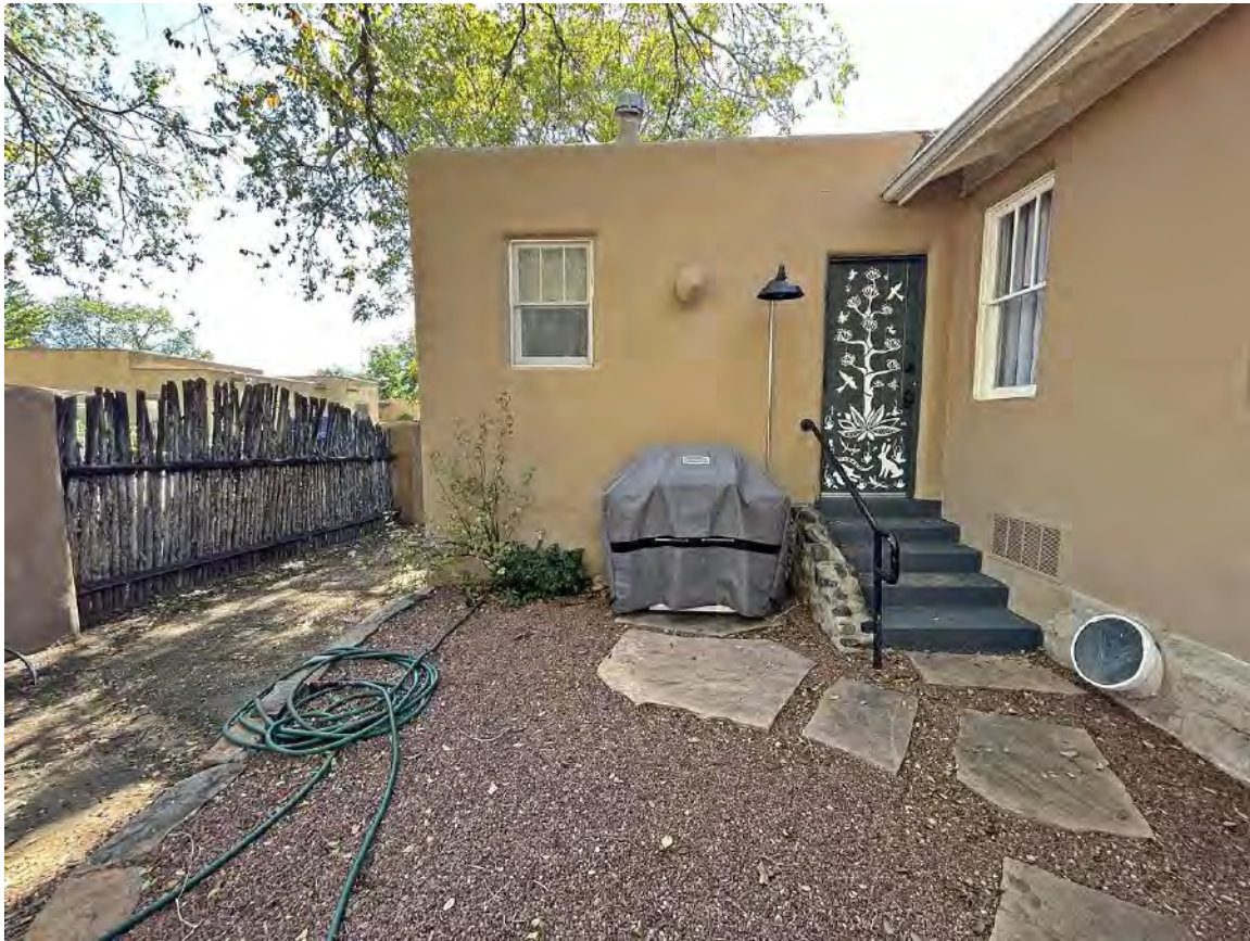
Photo 12: Addition, north elevation. Camera facing south.
