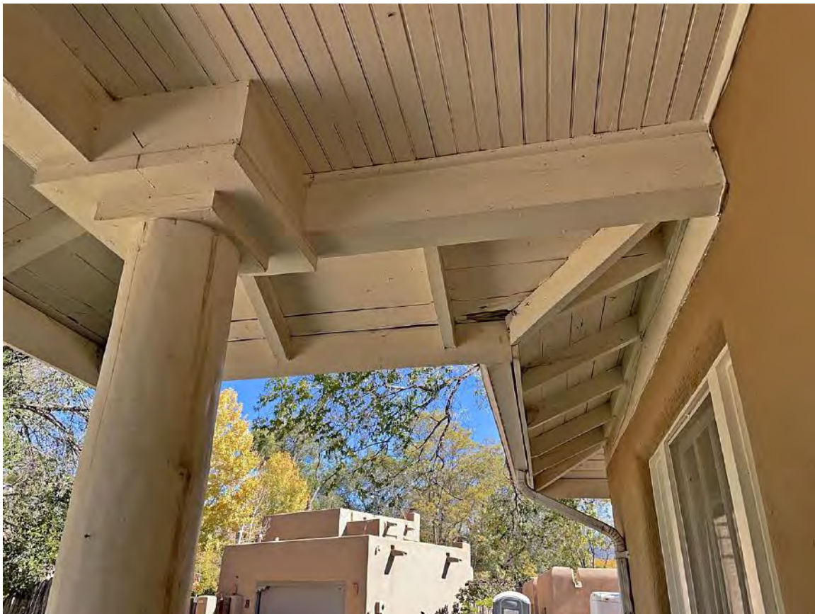
Photo 6: North façade, detail of porch decking. Camera facing east.
