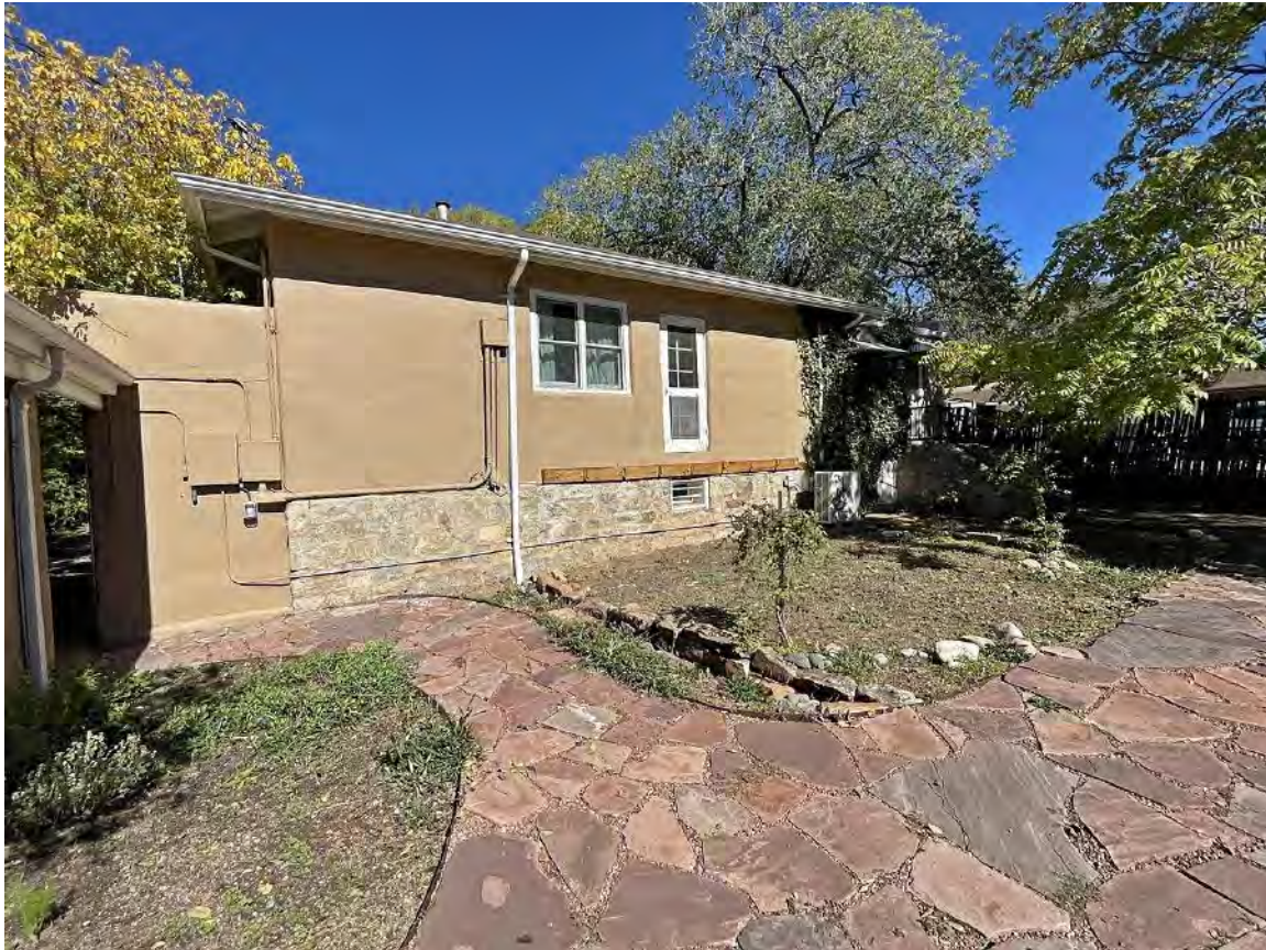
Photo 9: South elevation. Camera facing northeast.
