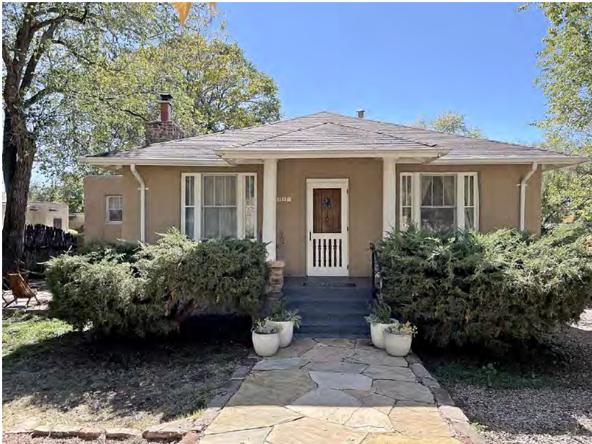
Photo 1: Front (north) façade. Camera facing south.
