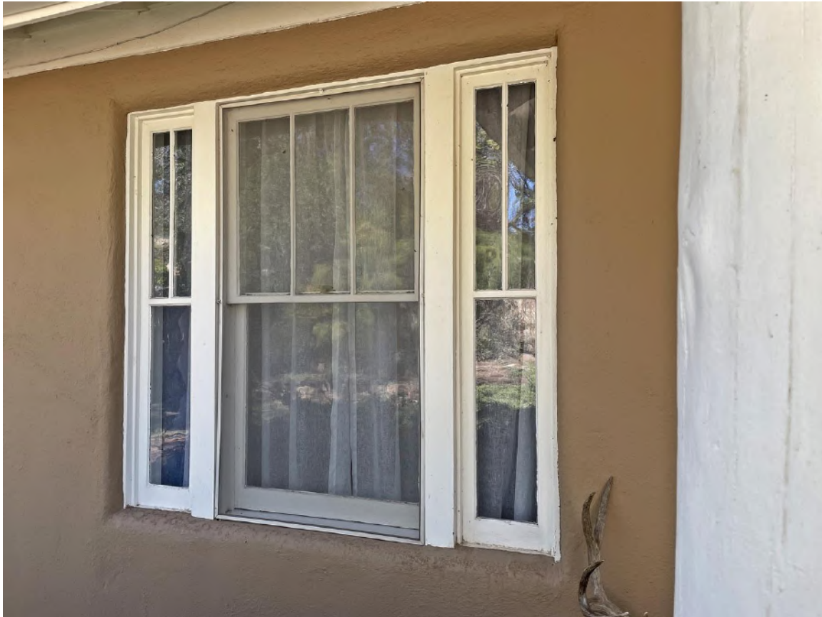
Photo 5: North façade, detail of combination window. Camera facing southeast.
