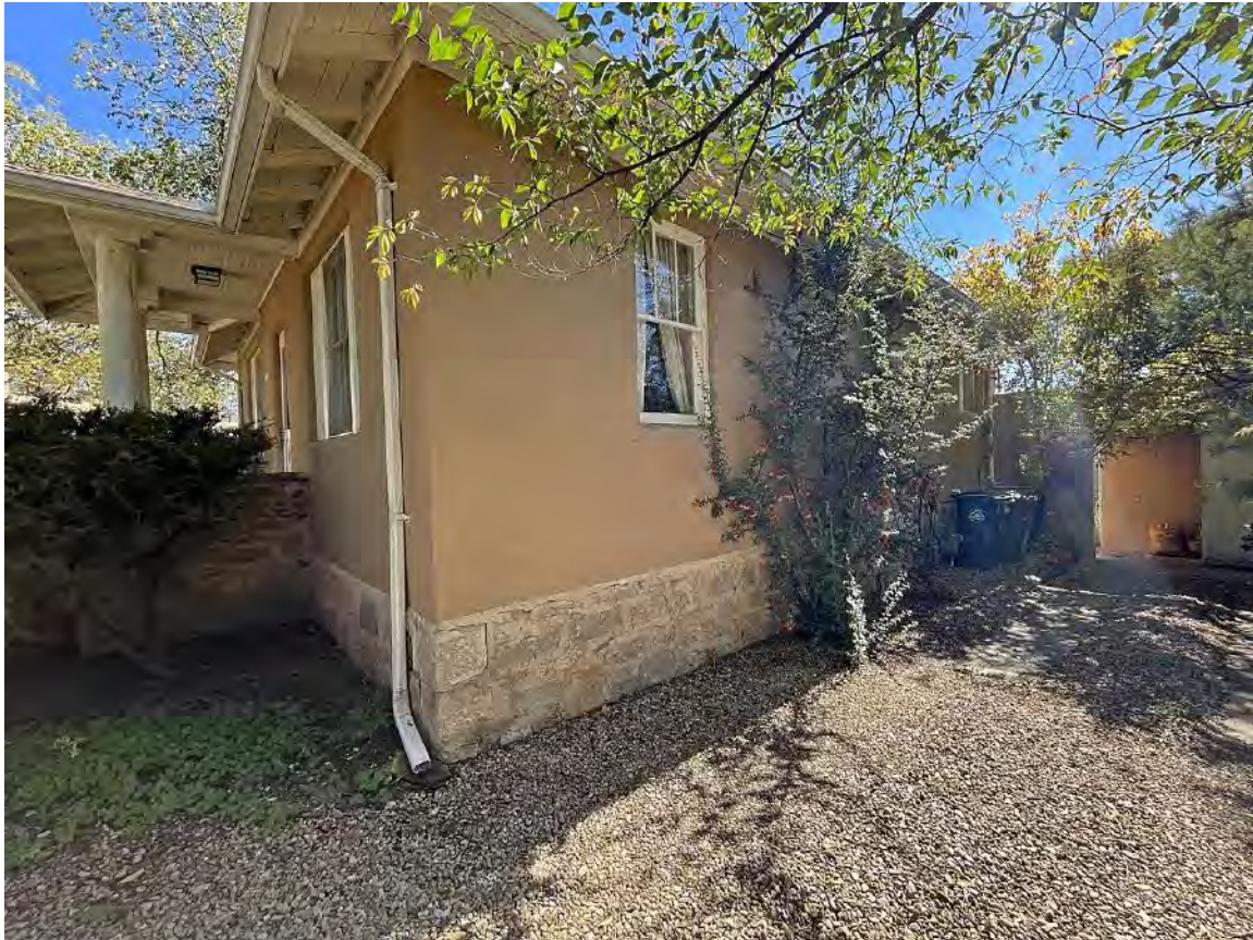
Photo 7: Northwest corner. Camera facing southeast.
