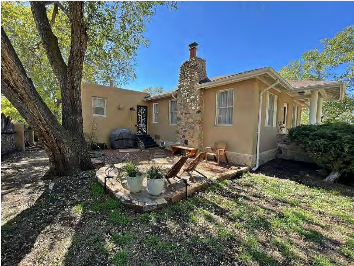
Photo 13: East elevation. Camera facing southwest.
