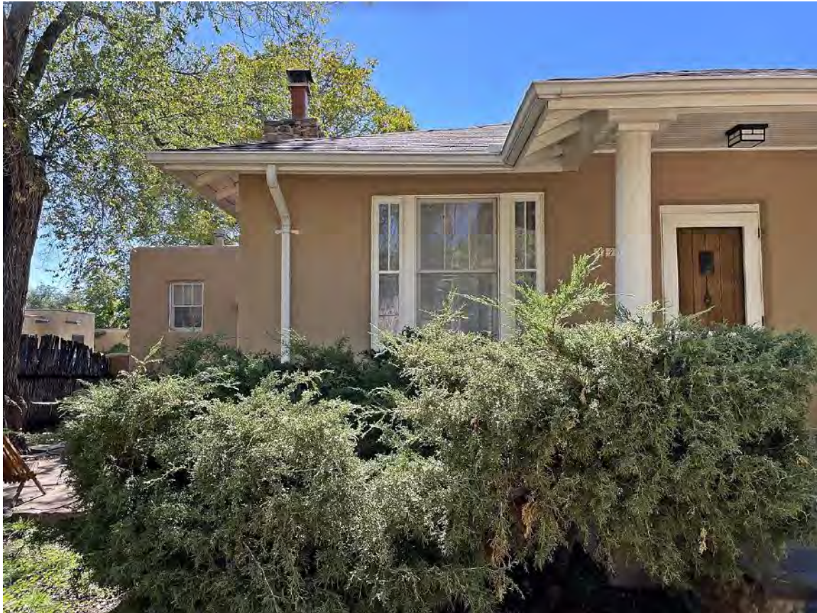
Photo 2: Partial north façade with addition at rear. Camera facing south.
