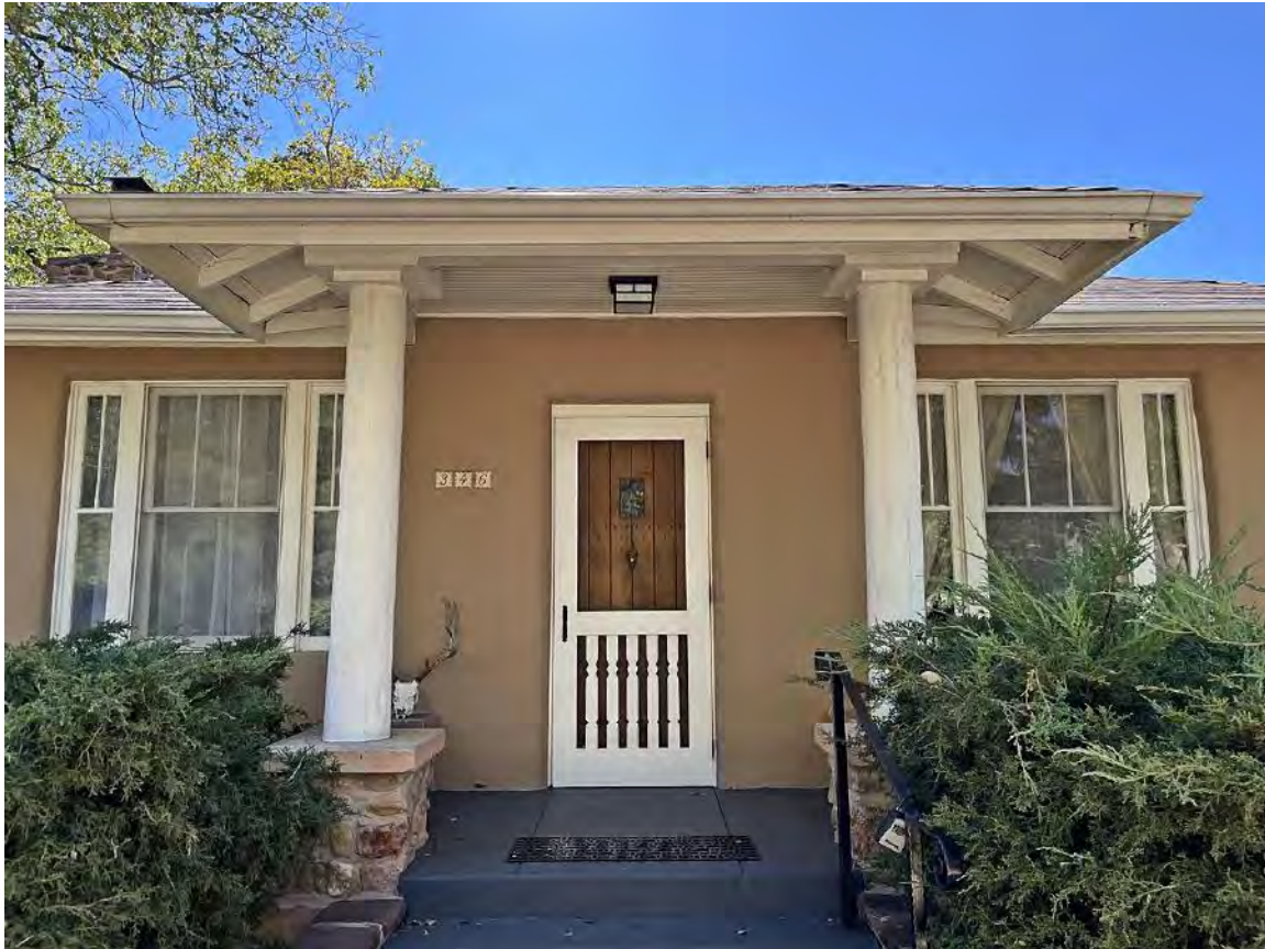
Photo 3: North façade entry. Camera facing south.
