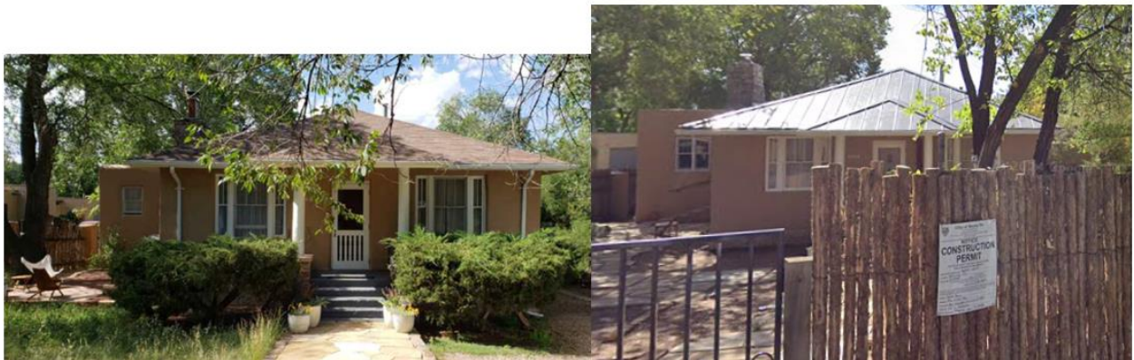
Figure 2: Pre (2022) and Post (2024) construction
