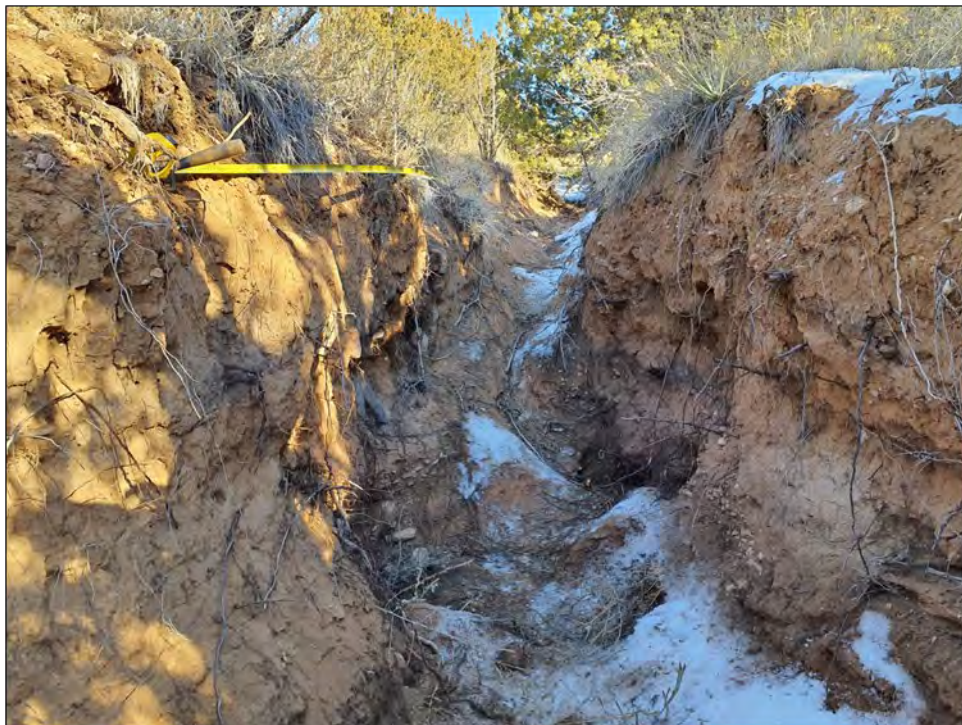
Figure 4-70. LA 202471, site overview of drainage, facing east (Frame T10-3770).
