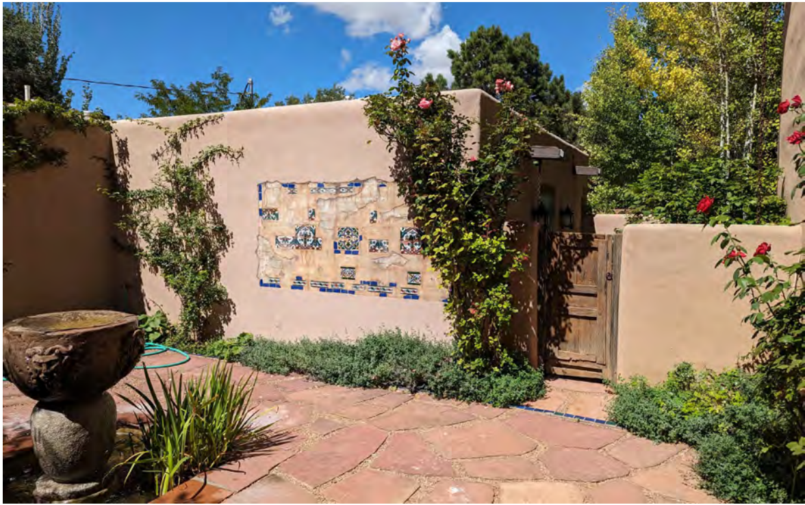
CENTER SOUTH GARAGE ELEVATION LOOKING NORTH
