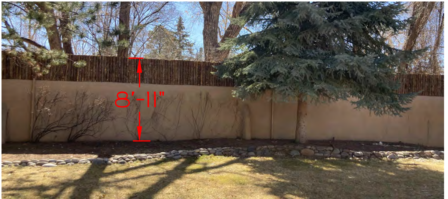
SOUTH FENCE FROM OUR PROPERTY
