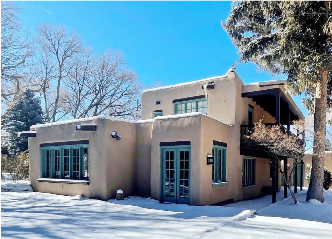
Photo 8: East elevation, dining room addition. Camera facing southwest.
