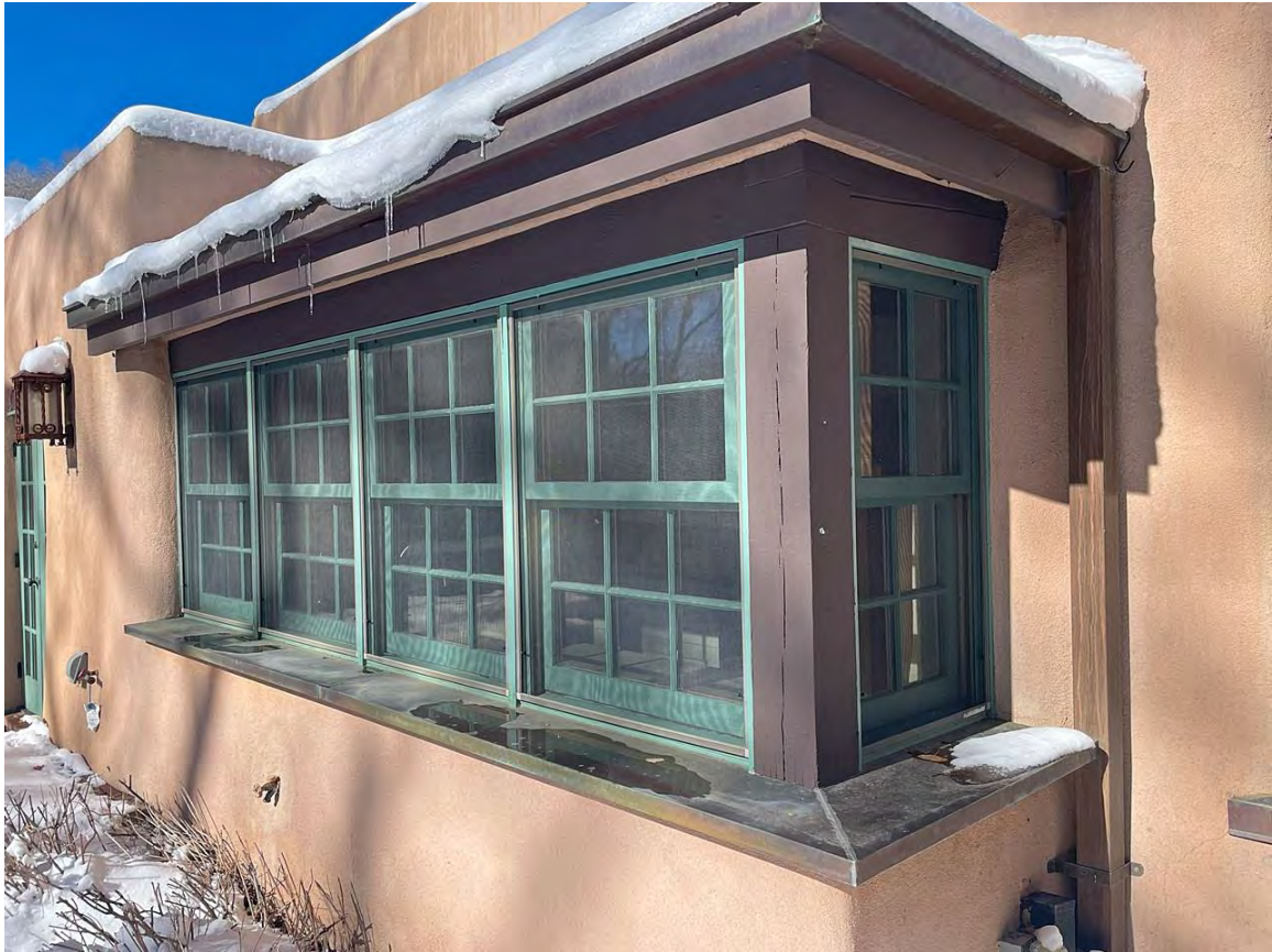
Photo 12: South elevation, kitchen extension. Camera facing northwest.
