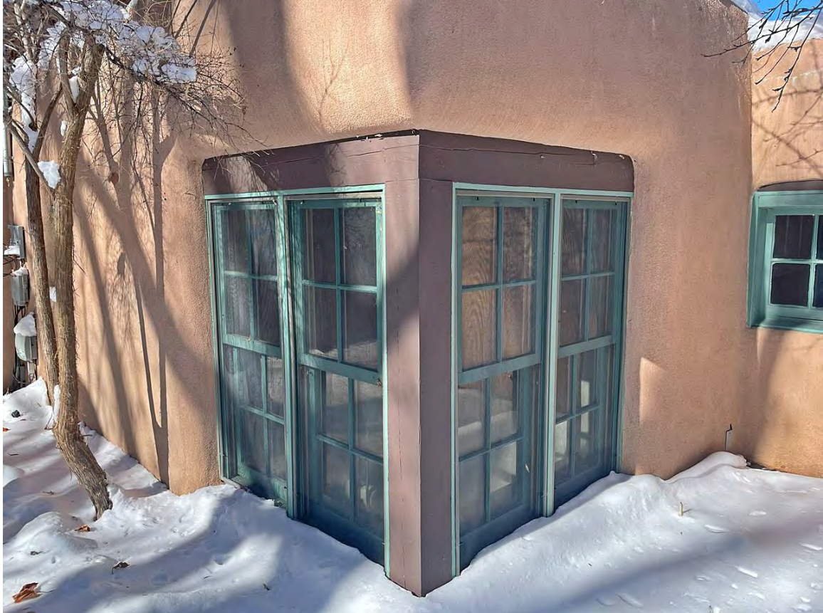
Photo 14: Non-historic bump-put bathroom addition. Note wall juncture, right. Camera facing northwest.
