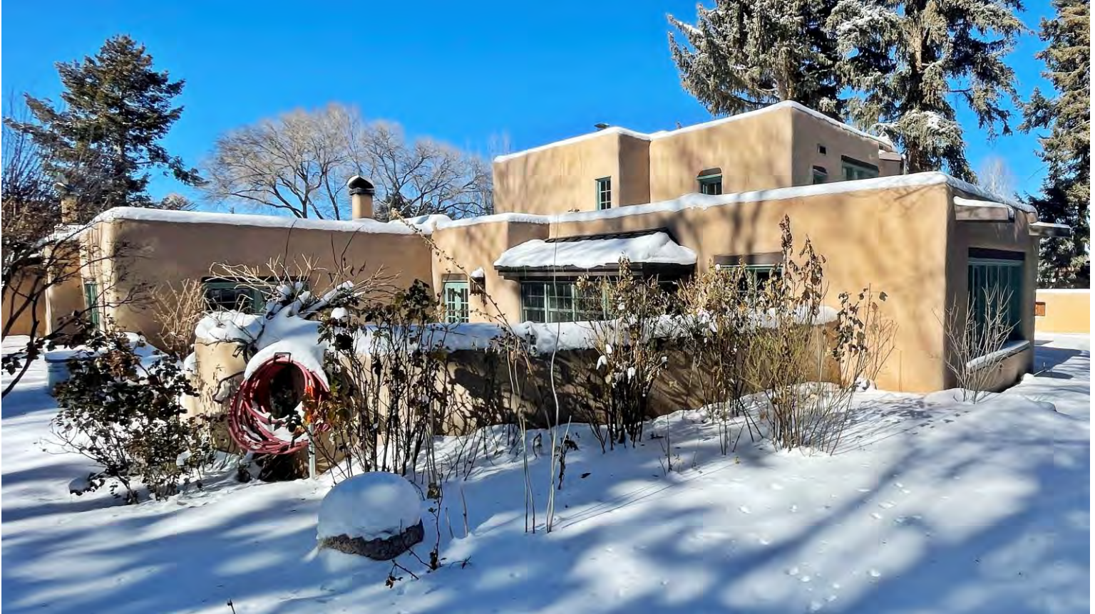
Photo 10: Full south elevation. Primary bedroom wing (former apartment), left; infilled portal and kitchen extension, center; dining room addition, right; historic two-story core block, background. Camera facing northwest.
