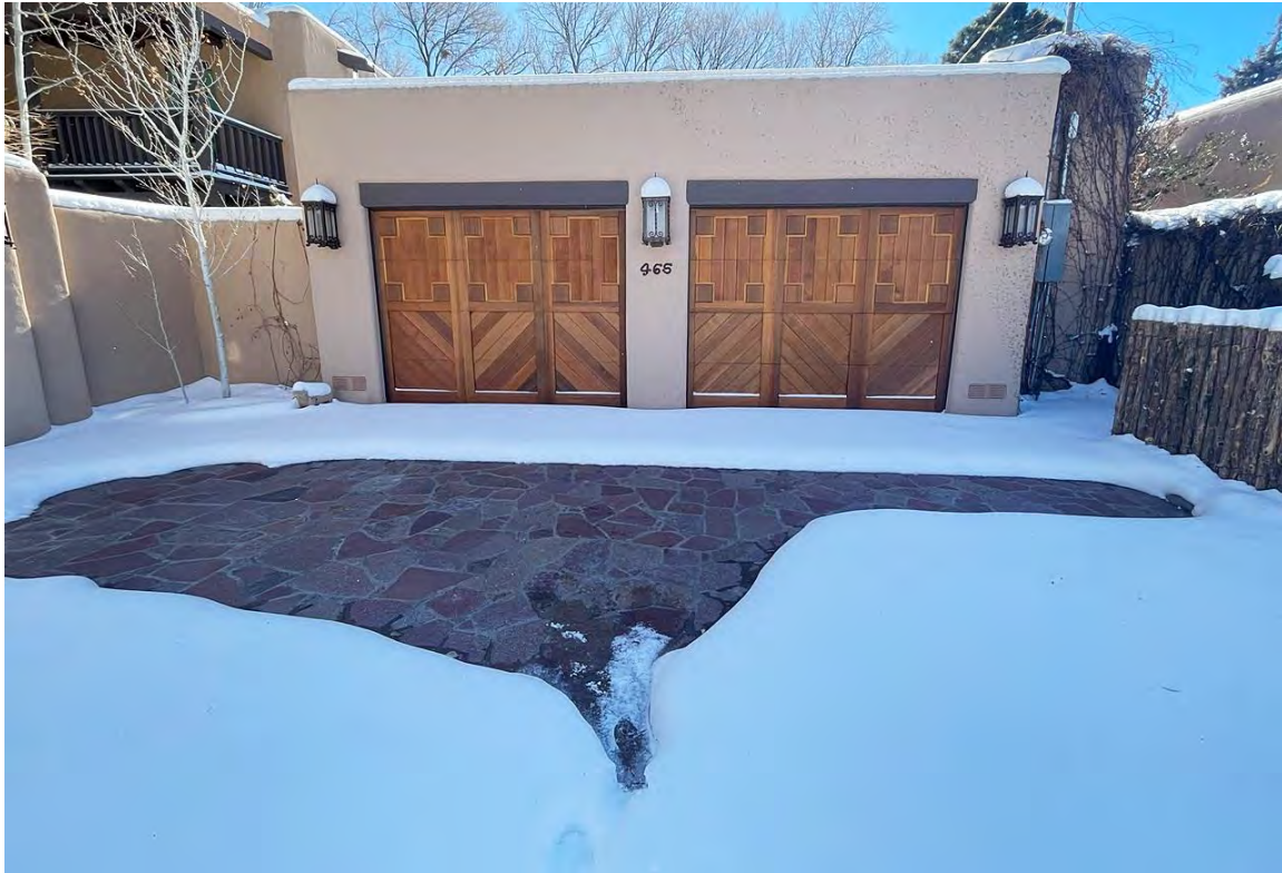
Photo 18: Non-historic two-car garage, north elevation. Camera facing south.
