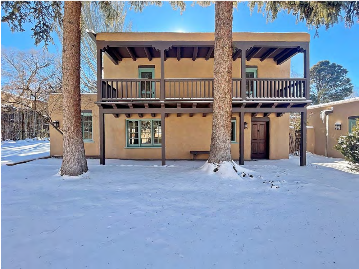
Photo 4: North façade of historic two-story core block. Camera facing south.
