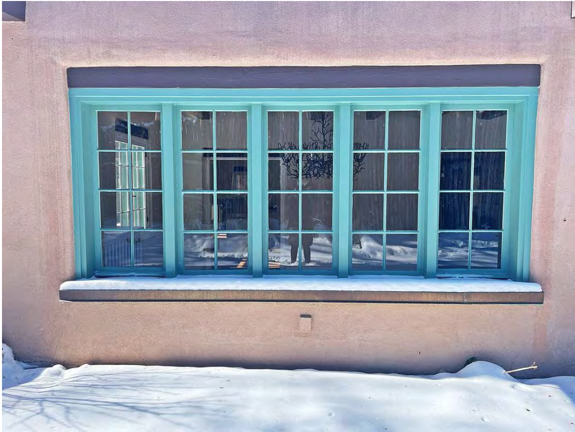
Photo 9: Closeup of dining room window. Camera facing west.
