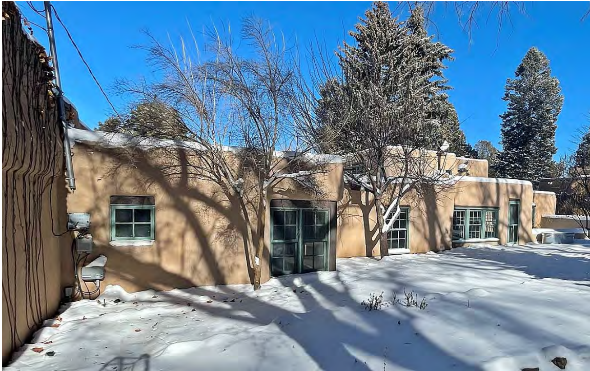
Photo 13: Full South elevation. Non-historic bump-put bathroom addition, left; primary bedroom wing, center; infilled portal and kitchen extension, right; dining room addition, extreme right. Camera facing northeast.
