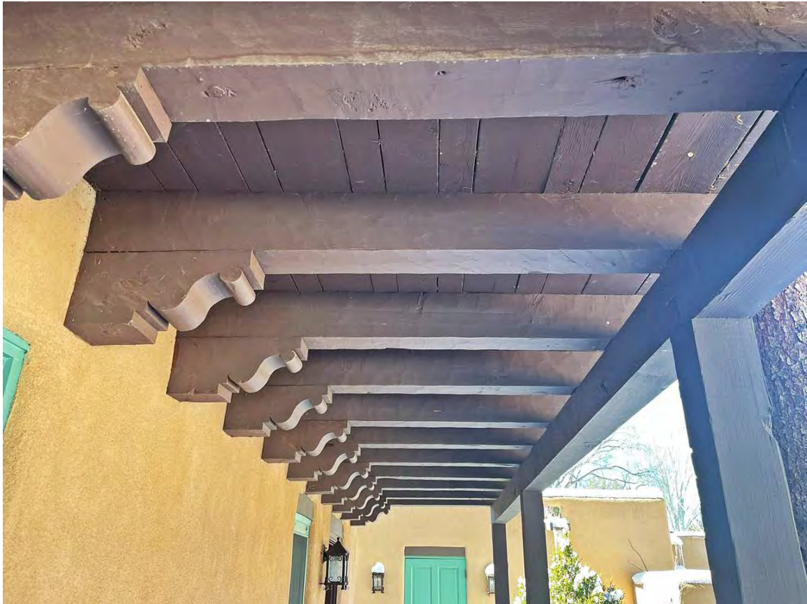
Photo 6: Beams and decking of second-story porch. Camera facing up.
