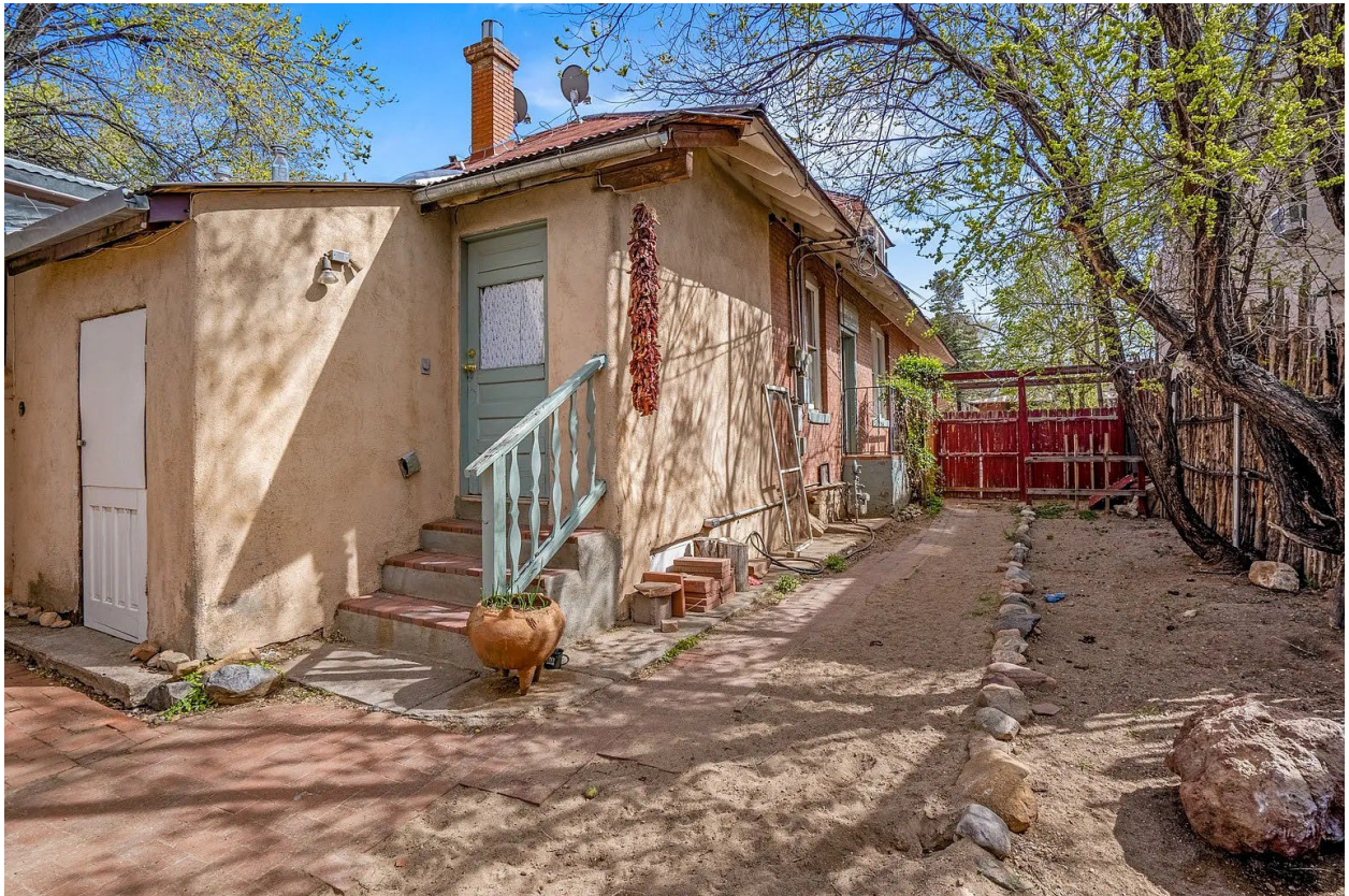
Figure 2: Addition in 2023, prior to demolition. Note attachment to original building's eaves. Addition was removed, roof repaired, and construction of a new addition that is 42 square feet larger (through the squaring off of the addition at the original entryway) than the historic addition.
