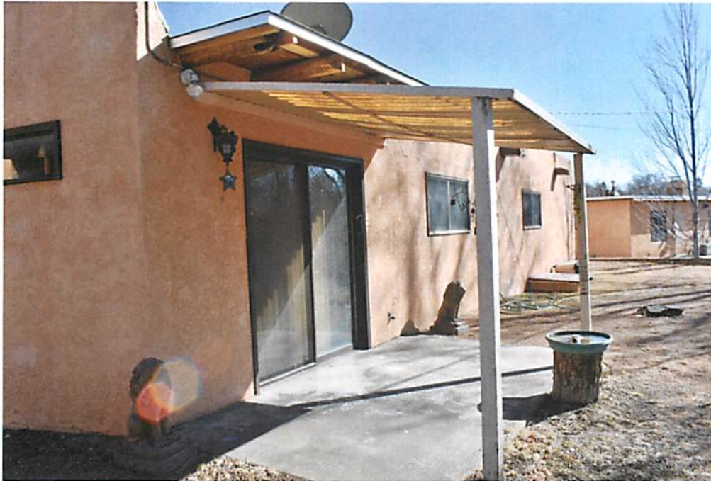
Photo 2: West elevation, facing south (Sharon Joyce, February 23, 2018).
