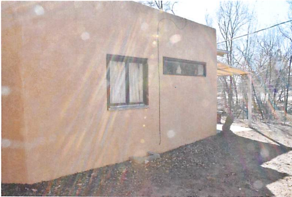
Photo 3: North elevation, facing southwest (Sharon Joyce, February 23, 2018).
