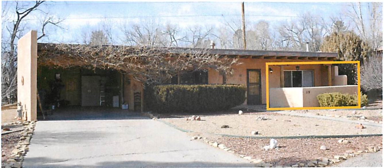
Photo 1: Street and south elevations, facing northwest. Box indicates removed portion of angled patio wall.
