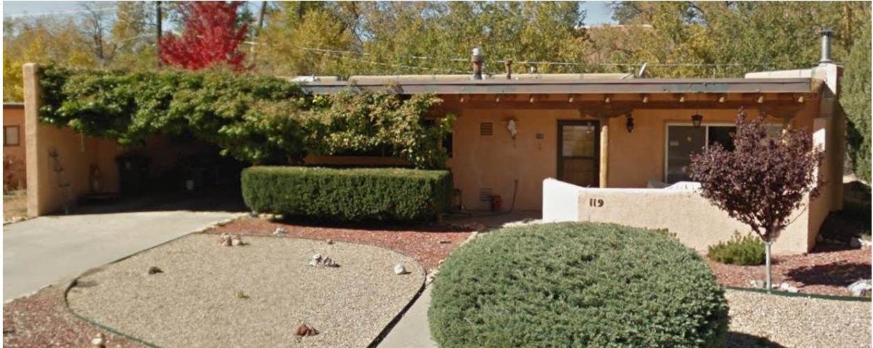
Figure 2: East Street Facing Elevation of 119 Camino Santiago
