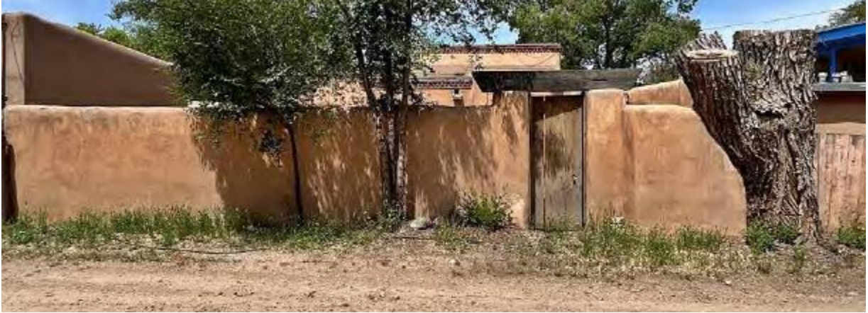
Figure 5: East Yard Wall
