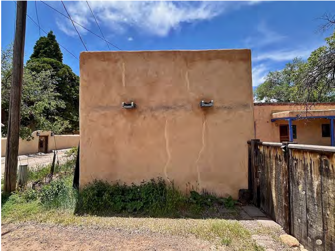
Photo 28: Guesthouse, south elevation. Camera facing south.
