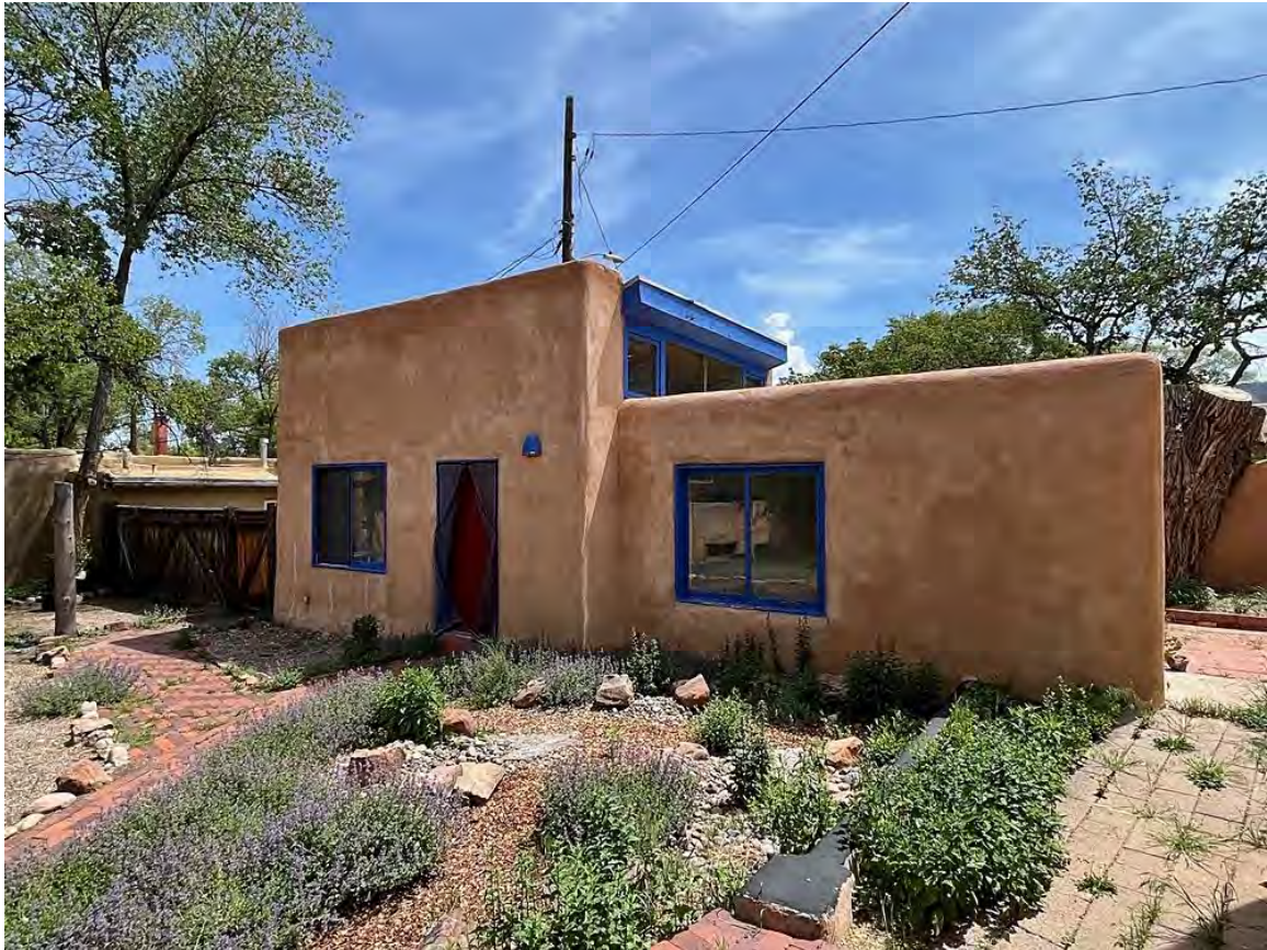
Photo 25: Guesthouse, west elevation. Camera facing northeast.
