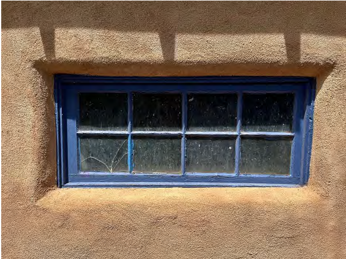
Photo 32: Garage, east elevation. Window detail. Camera facing west.
