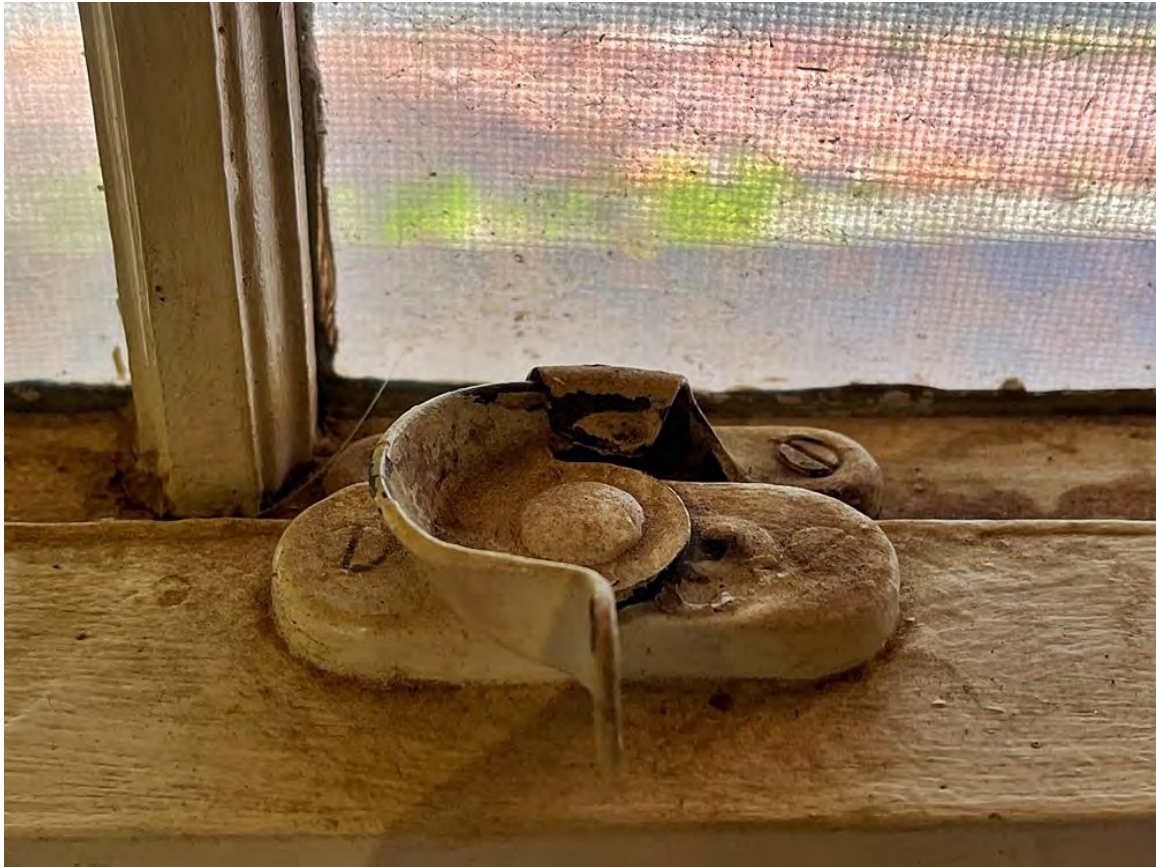
Photo 8: Primary House, north elevation. West window detail. Camera facing down.
