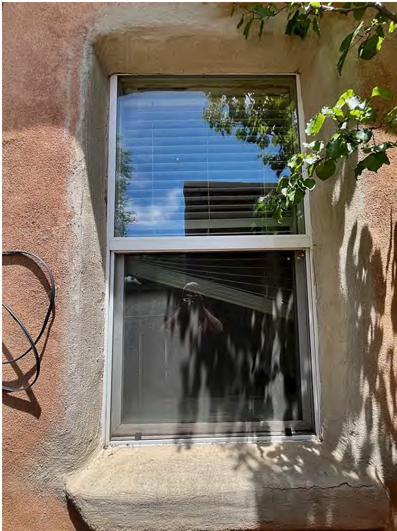
Photo 14: Primary House, south elevation. West window. Camera facing north.
