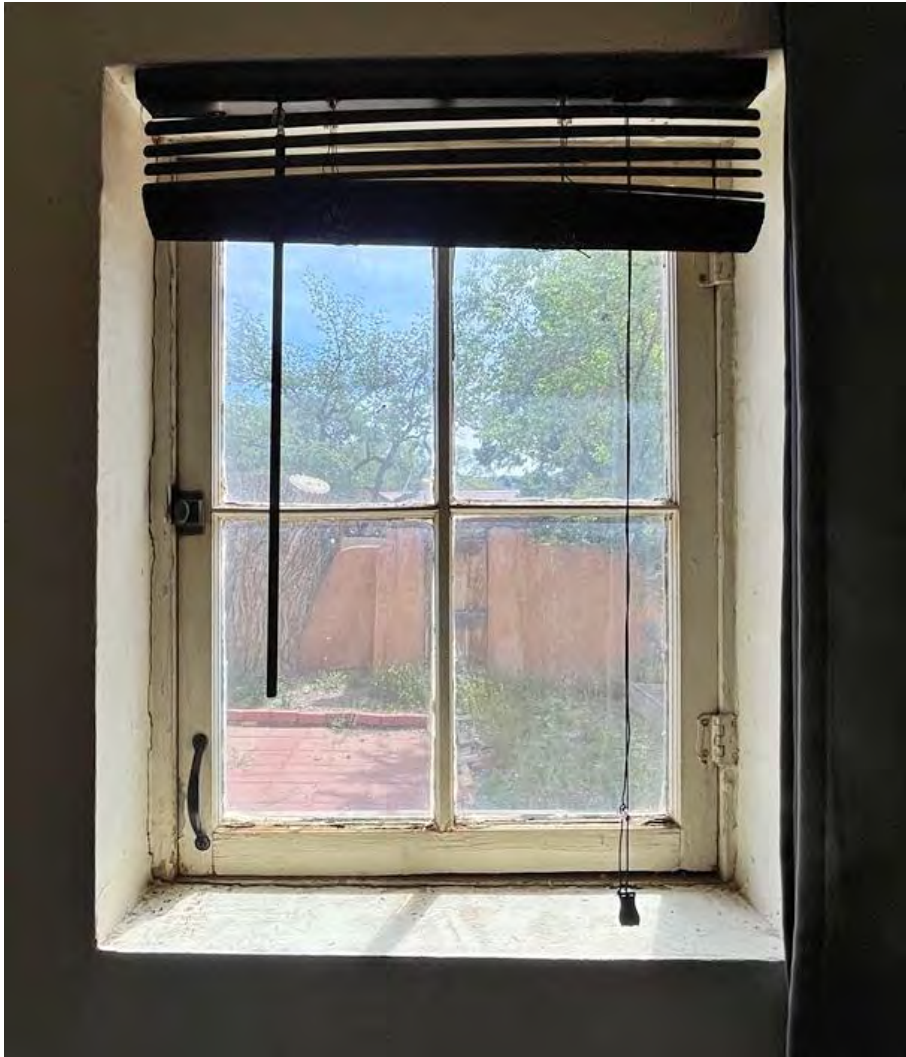
Photo 18: Primary House, east elevation. Window at closet. Camera facing east.
