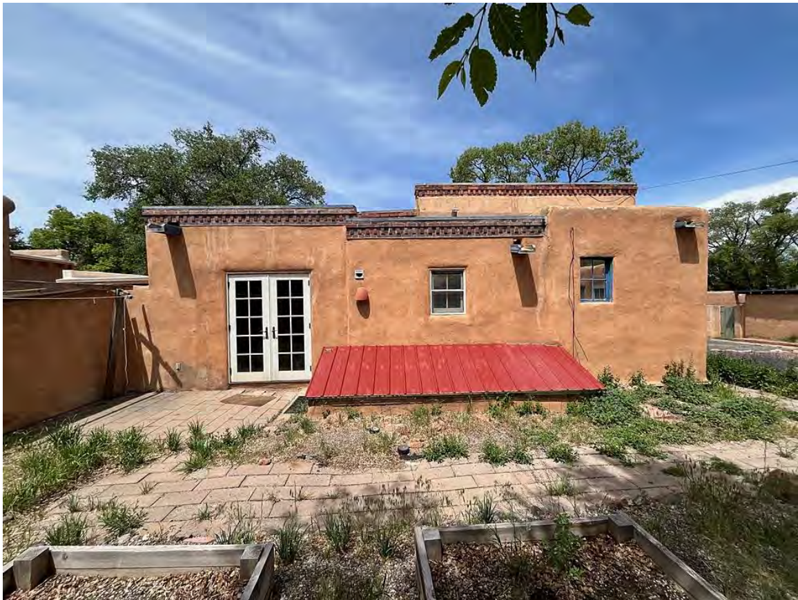
Photo 16: Primary House, east elevation. Camera facing west.
