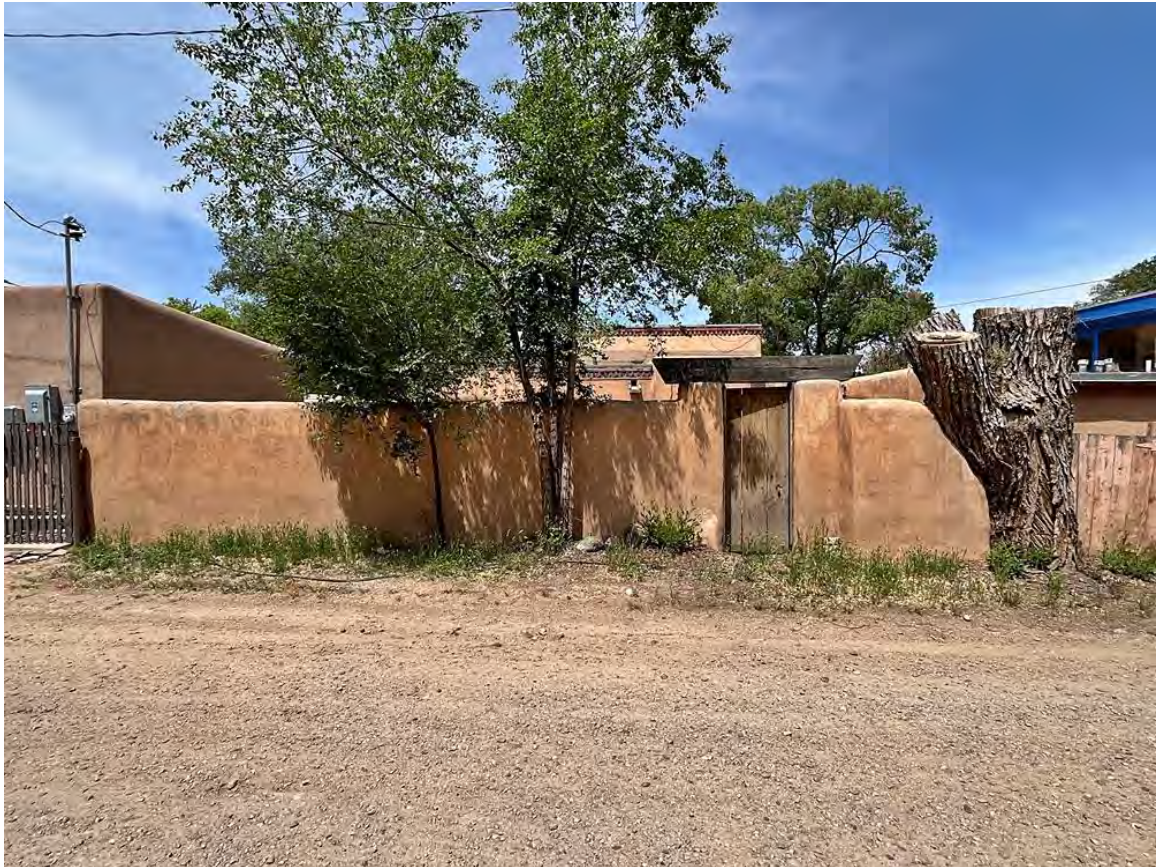
Photo 34: East yard/privacy wall along Camino Manzano. Camera facing southeast.
