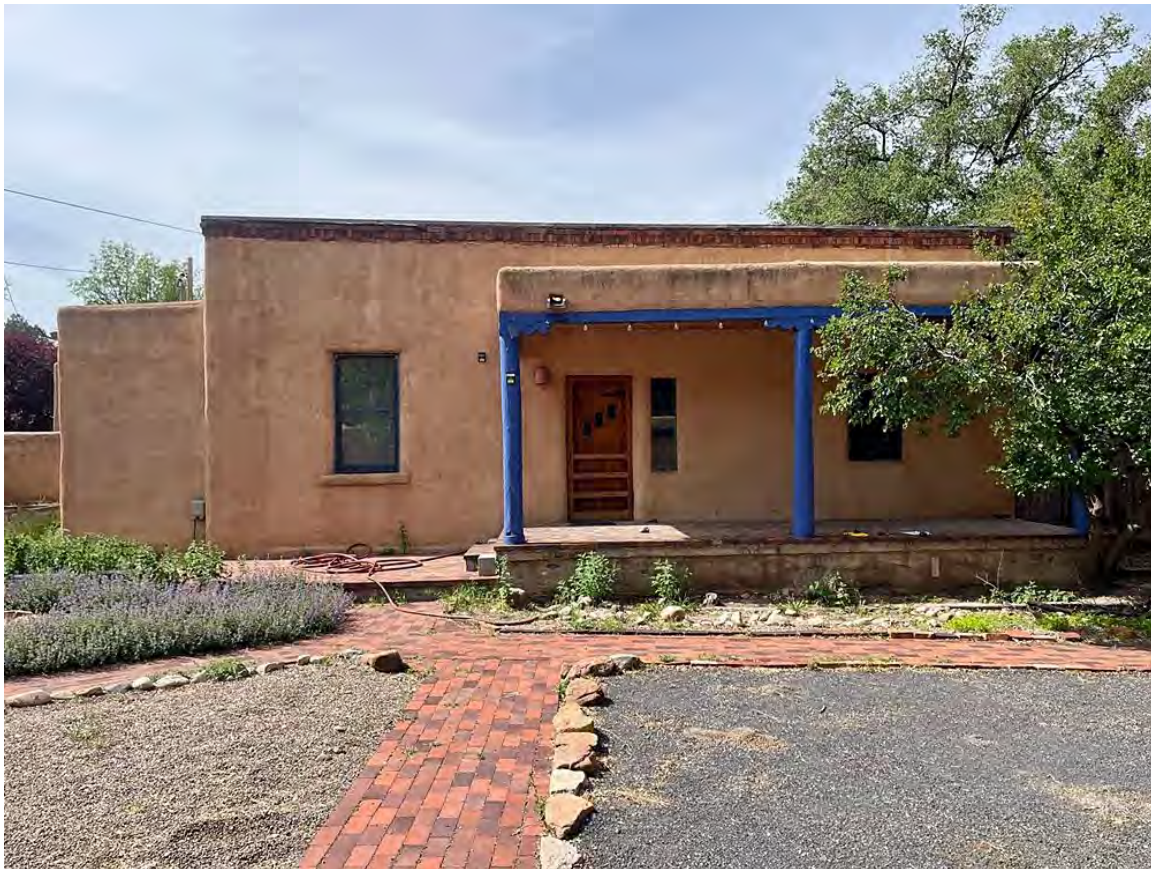
Photo 3: Primary House, north elevation. Camera facing south.
