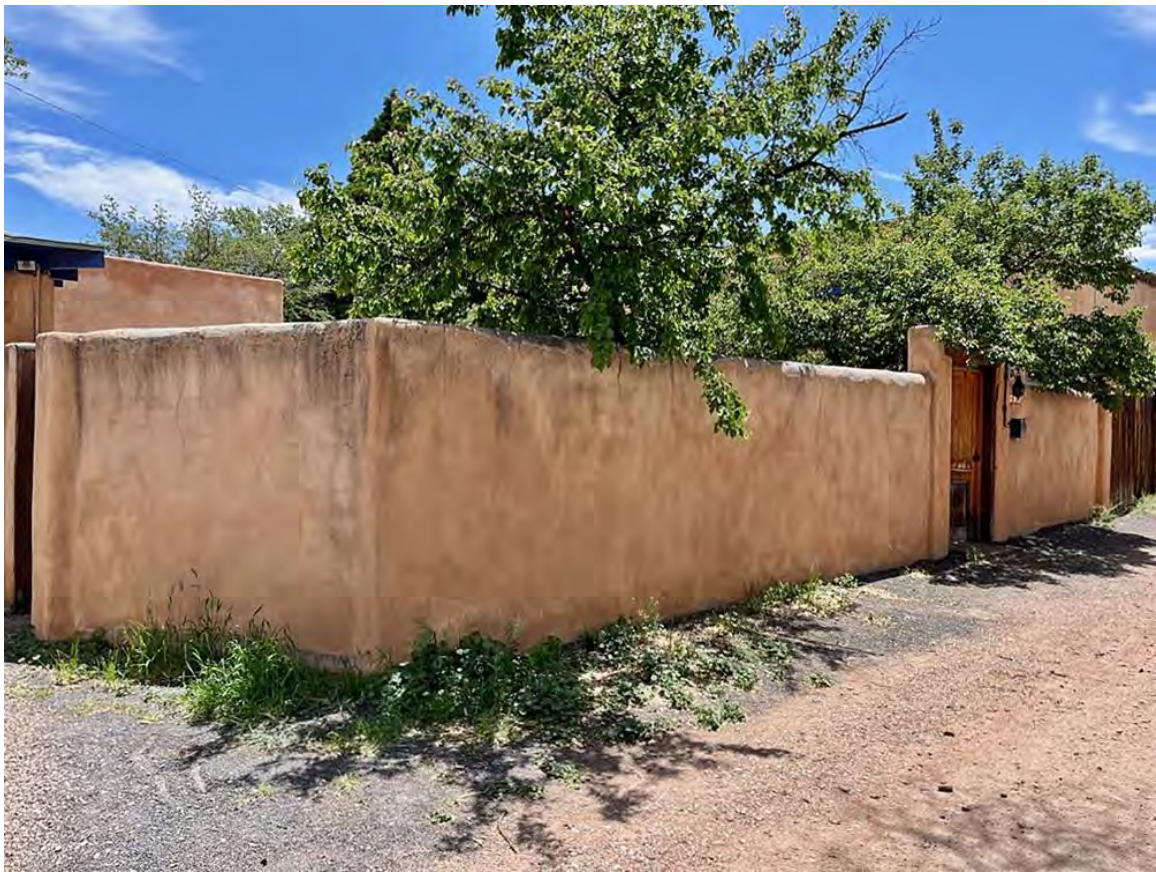
Photo 2: West yard/privacy wall. Camera facing southeast.
