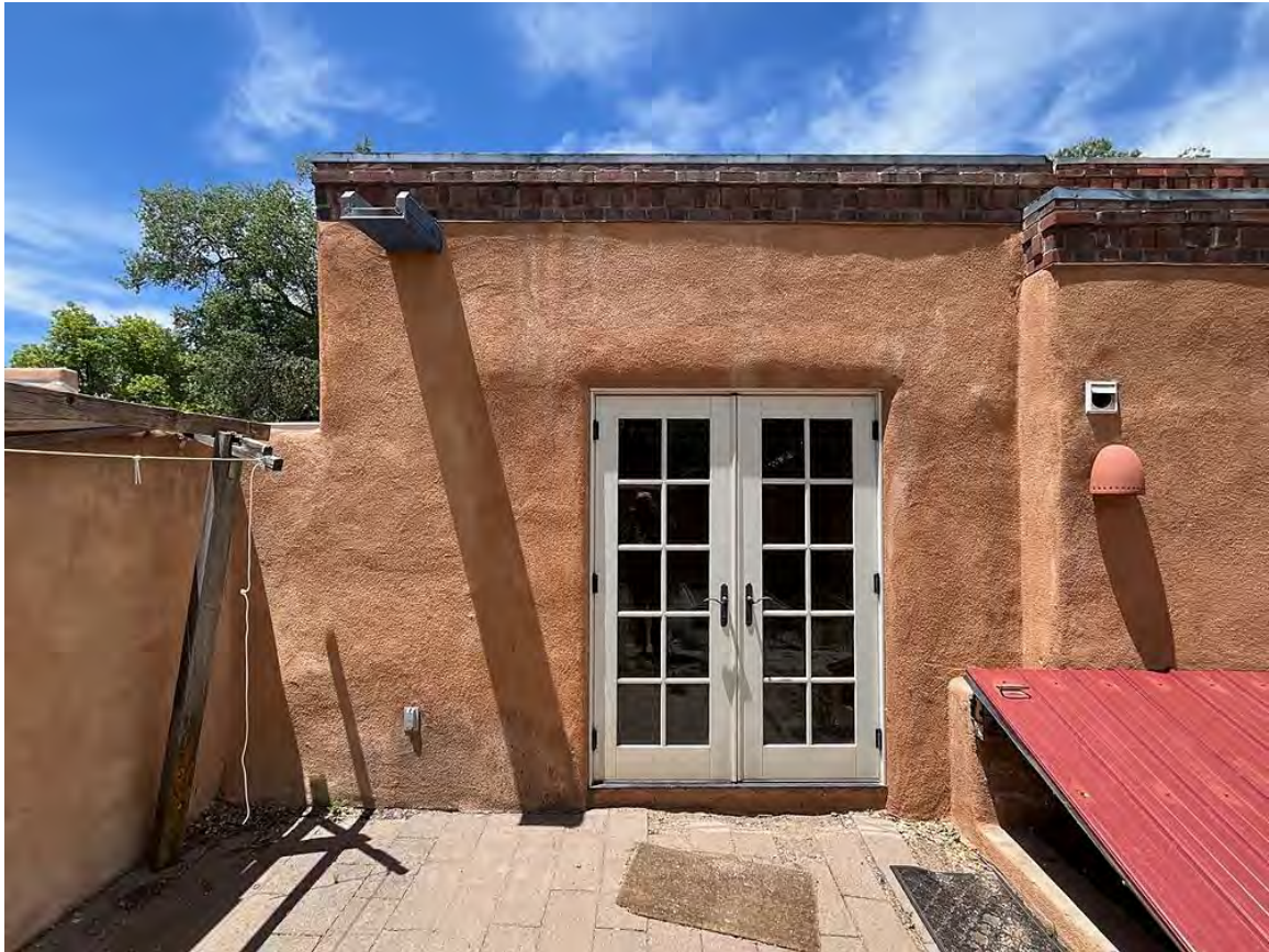
Photo 17: Primary House, east elevation. Entry to kitchen. Camera facing west.
