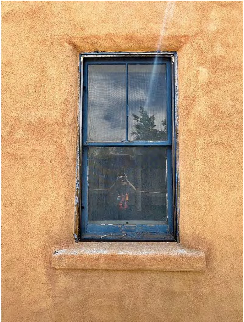
Photo 12: Primary House, west elevation. South windows. Camera facing east.
