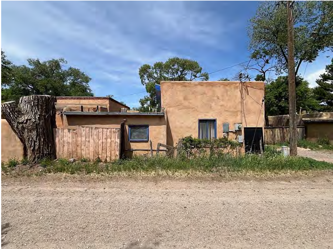
Photo 27: Guesthouse, north elevation. Camera facing west.
