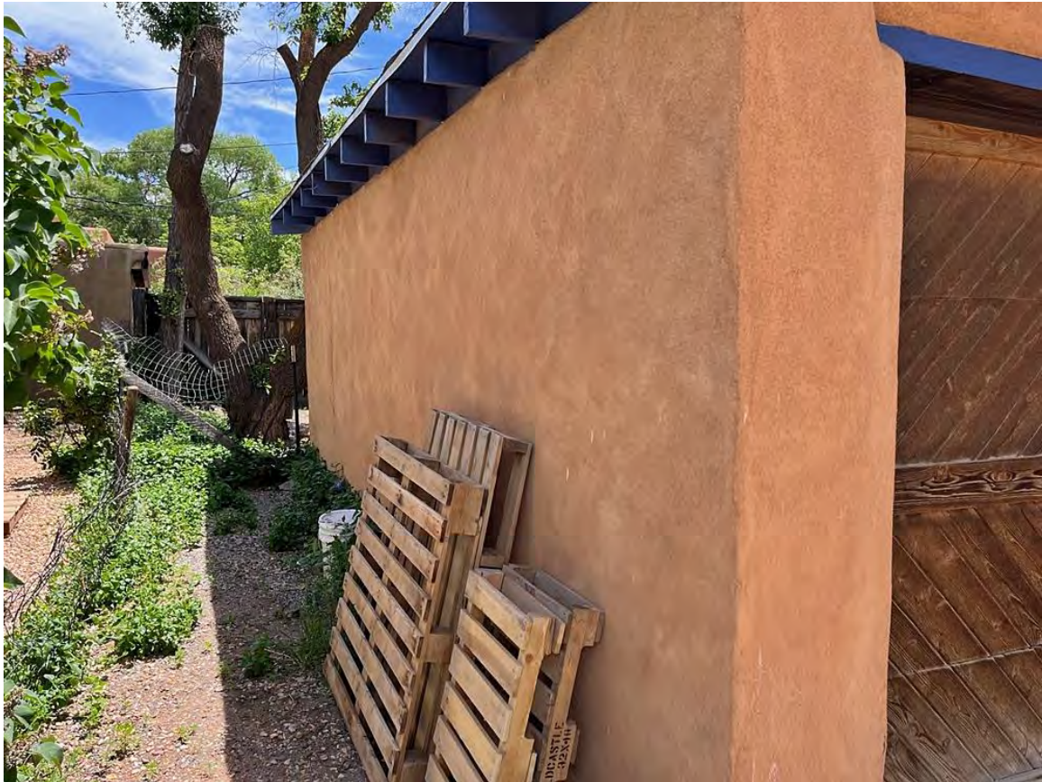
Photo 33: Garage, north elevation. Camera facing southeast.
