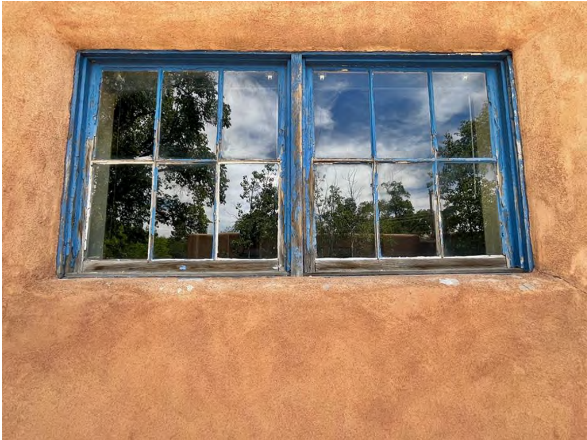
Photo 11: Primary House, west elevation. North windows. Camera facing east.
