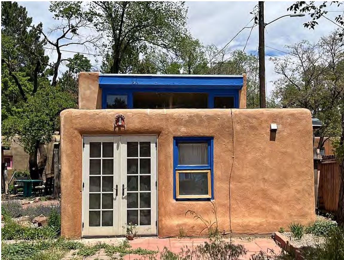
Photo 26: Guesthouse, south elevation. Camera facing north.
