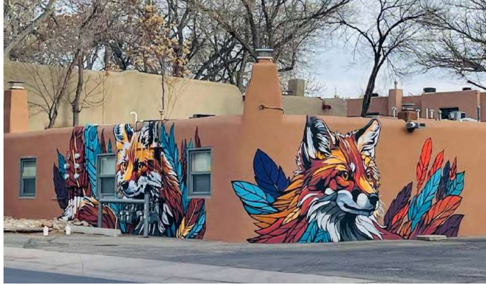
Figure 1. North and West publicly facing facades on Paseo de Peralta.
