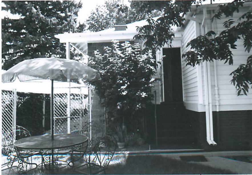
#35 west elevation, N end
