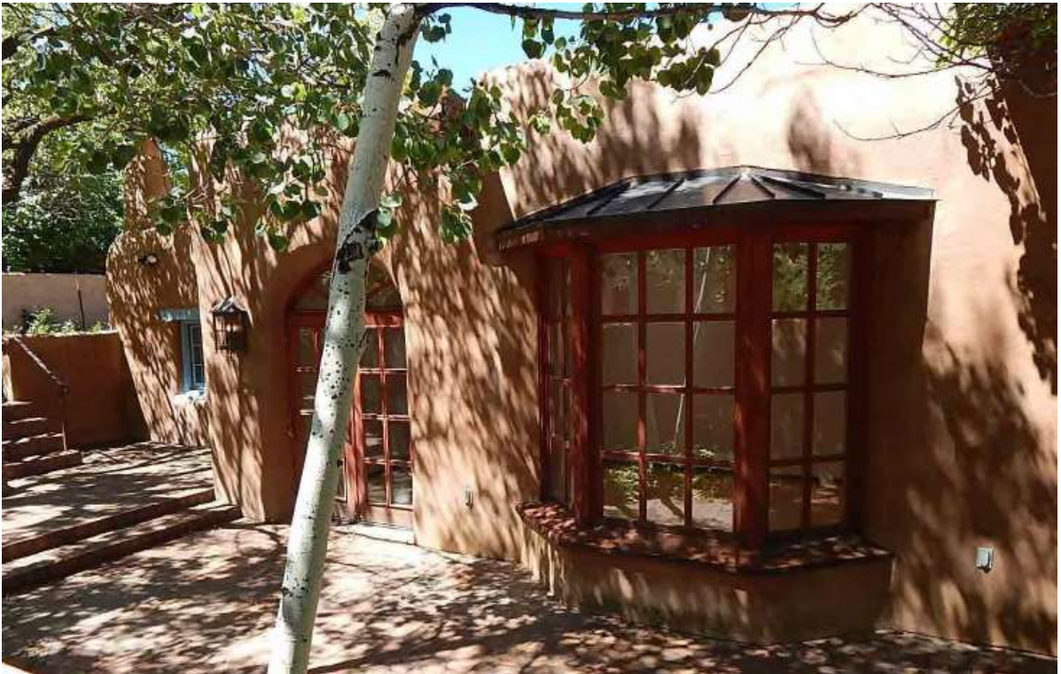
Figure 3. East Facade III.
