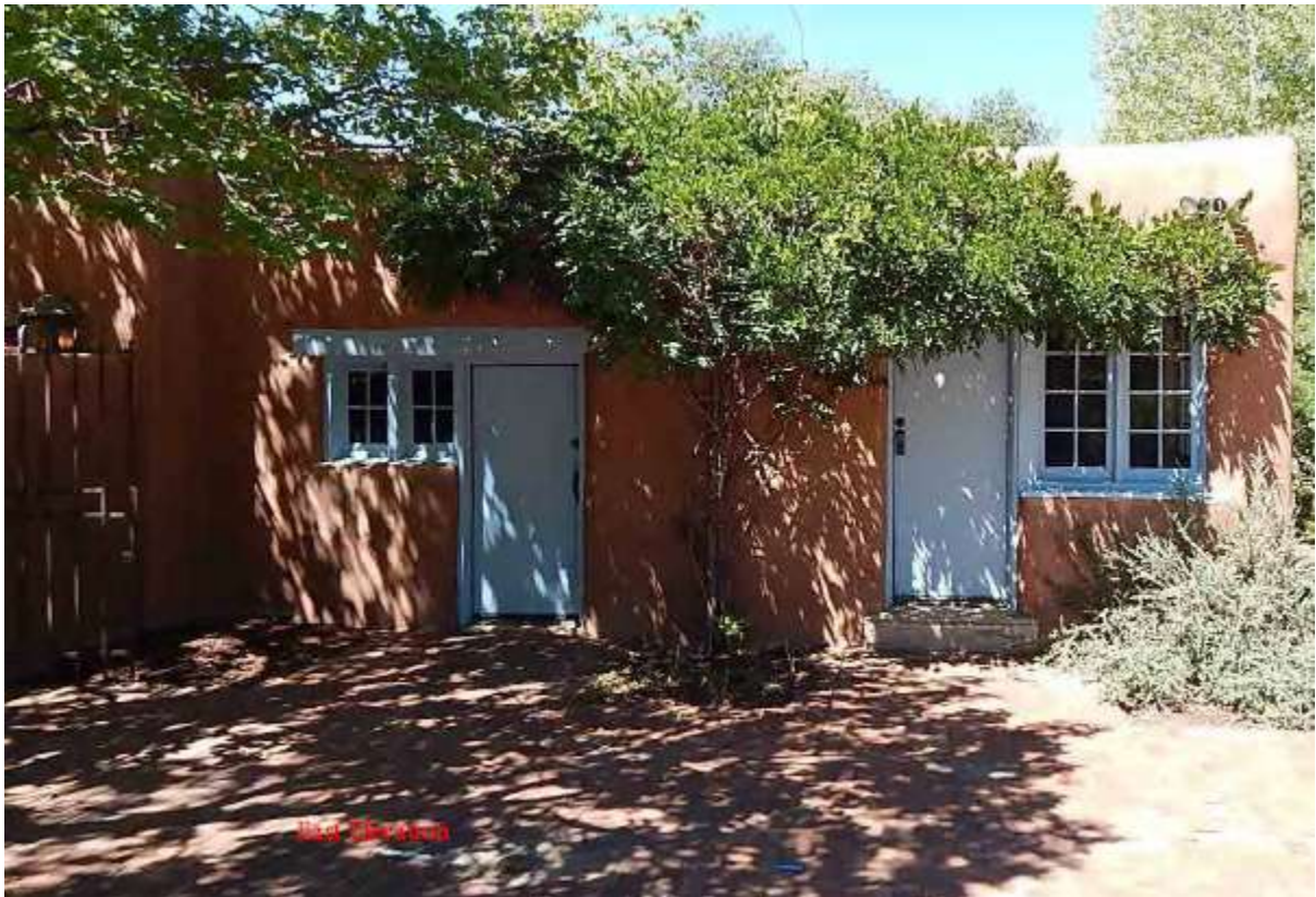
Figure 1. East Facade I.
