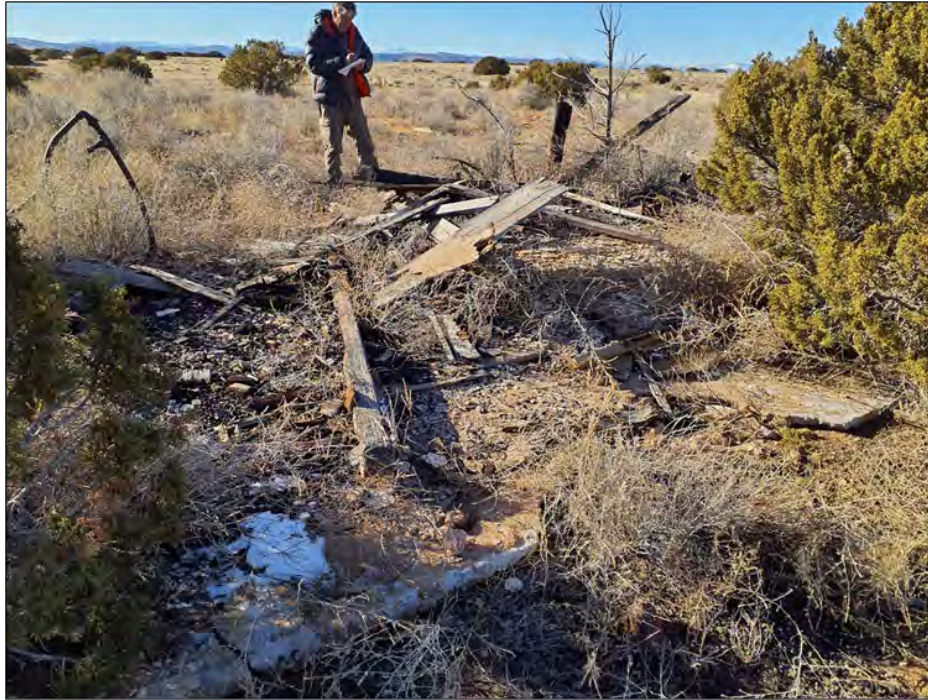
Figure 4-35. LA 54783, Feature 1 (F1), remnants of a two-room structure made from stucco and a stick frame. The structure was burnt. The concrete pad measures approximately 12 feet × 25 feet; view facing northwest (Frame T05-2464).
