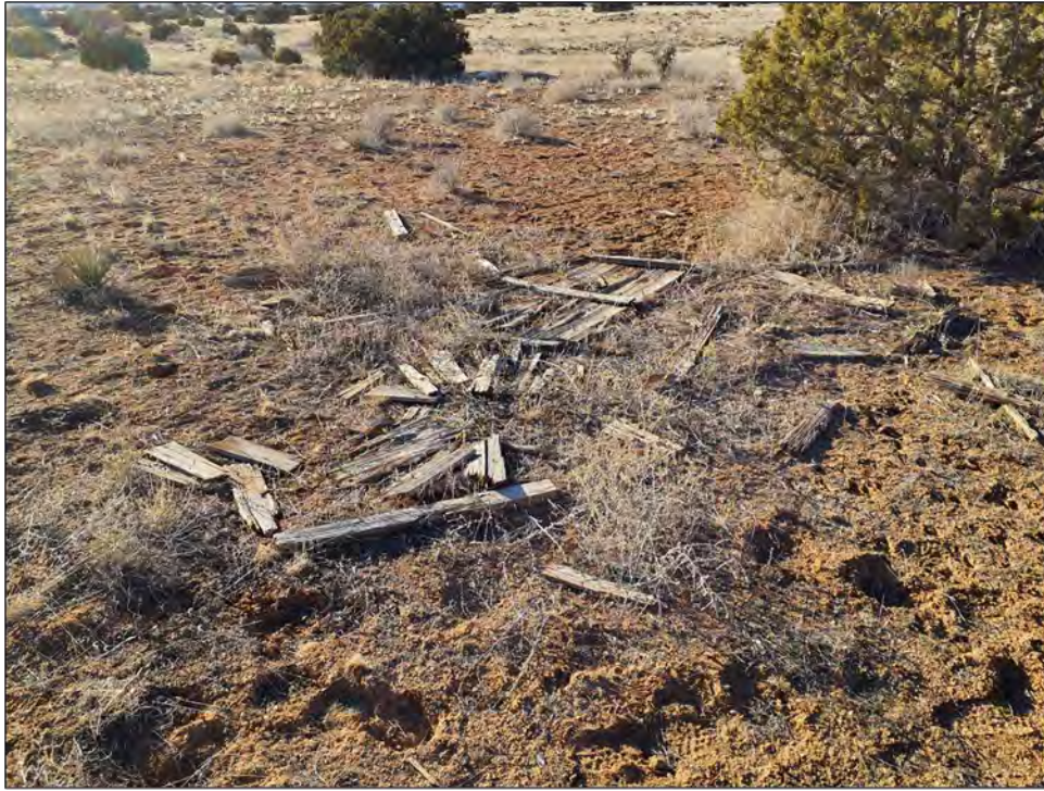
Figure 4-37. LA 54783, Feature 3 (F3), collapsed structure/outbuilding (possible outhouse); view facing northwest (Frame T05-9454).
