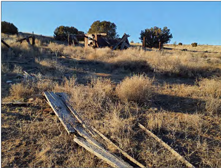
Figure 4-40. LA 54783, Feature 6 (F6), series of collapsed and partially collapsed outbuildings, corrals; view facing northwest from east side of feature (Frame T05-8232).
