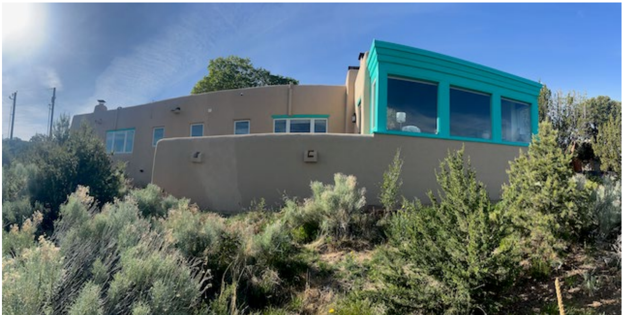
Photo of the northeast side (back) of home. Existing blue accent colors are legal nonconforming.
