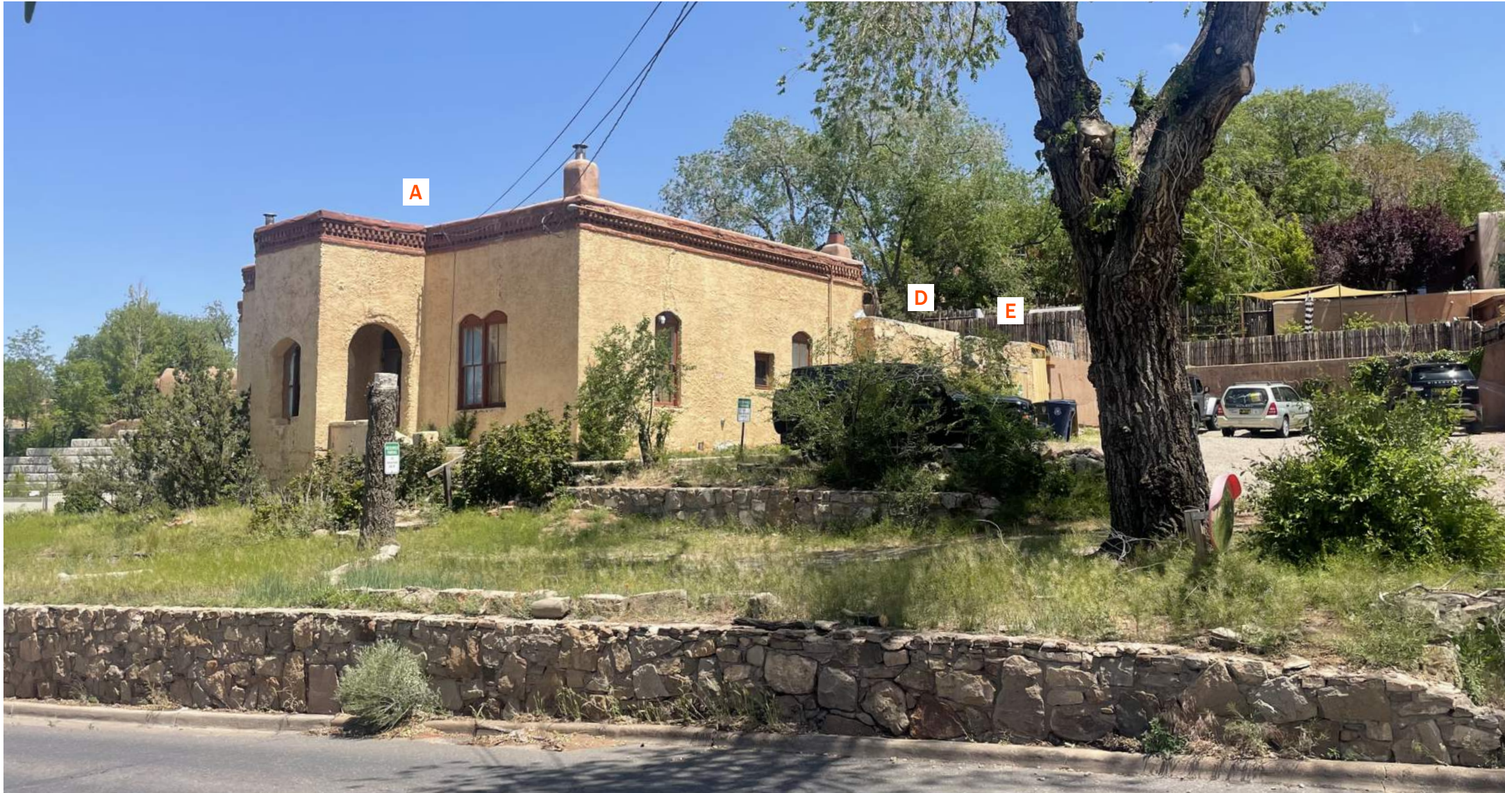
SITE FROM SOUTHEAST
