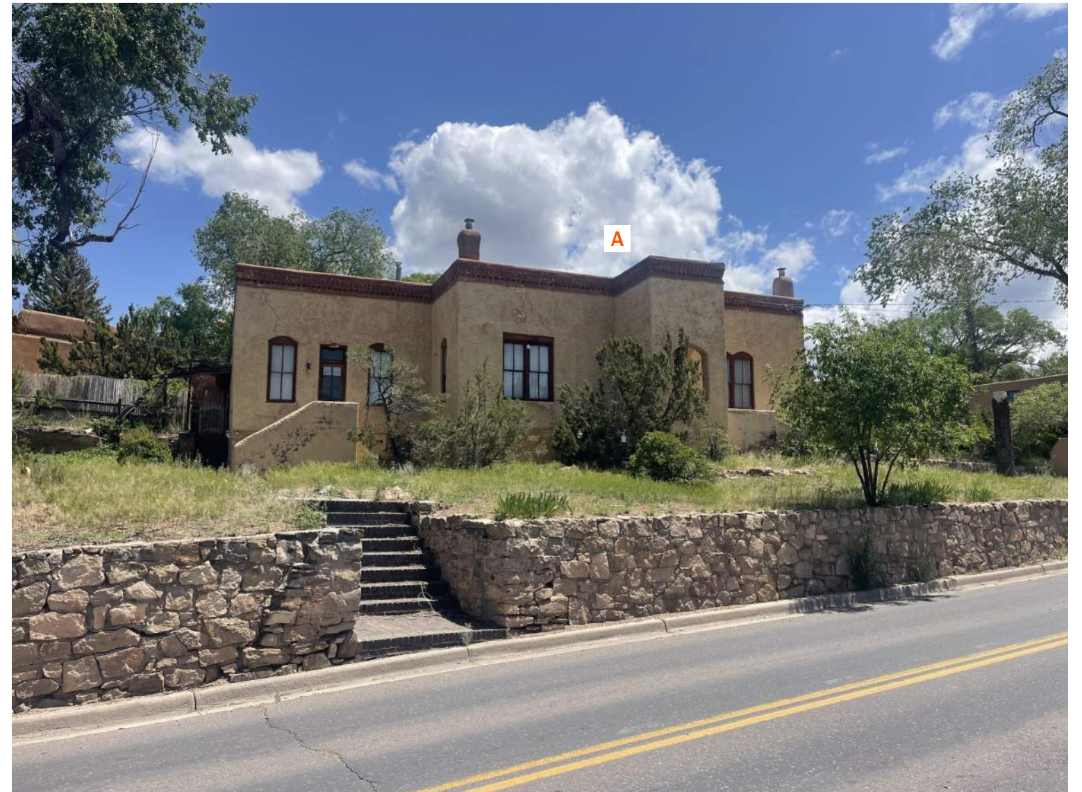
SITE FROM SOUTHWEST
