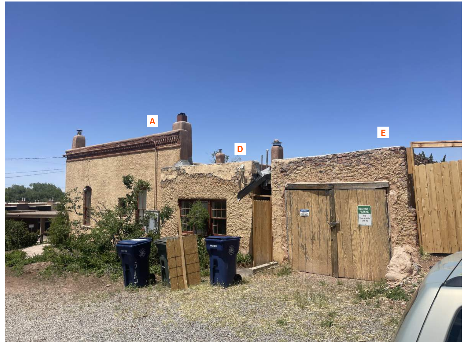
SITE FROM EAST
