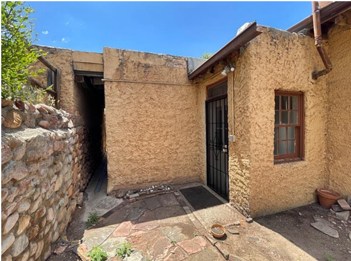
Photo 20: North retaining wall. Camera facing southeast.
