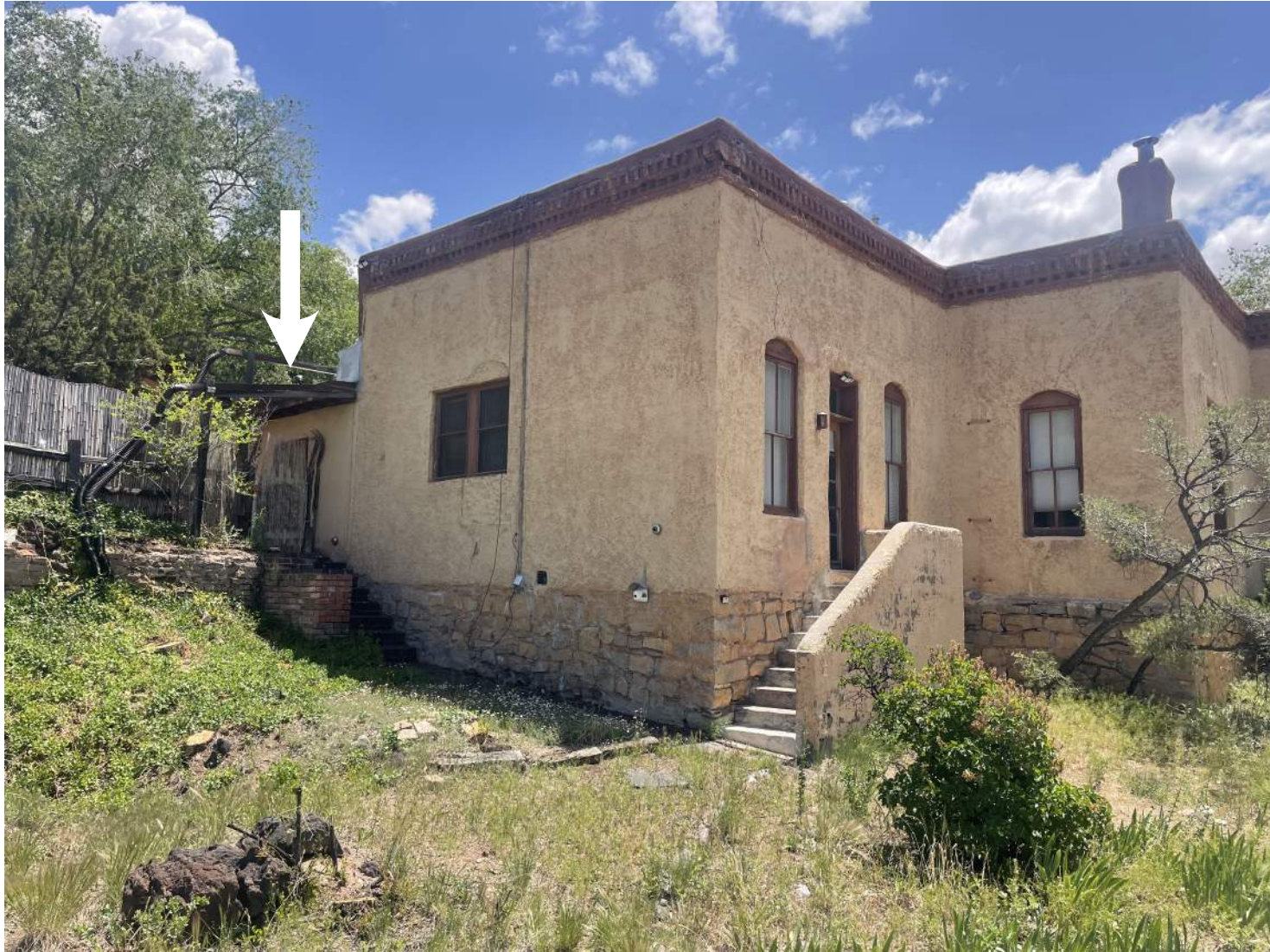
VIEW FROM SOUTH WEST
