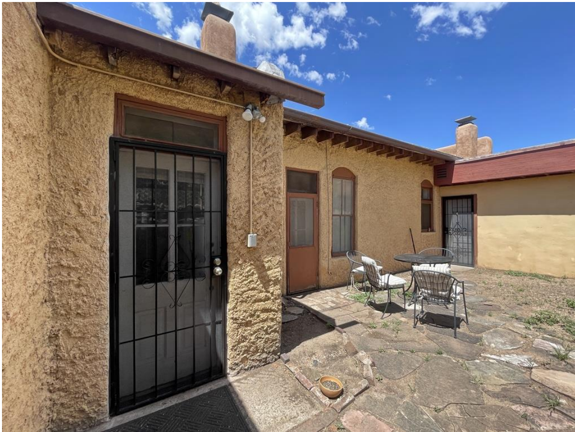
Photo 12: North elevation. Original garage (left); bedroom addition (right). Camera facing southeast.
