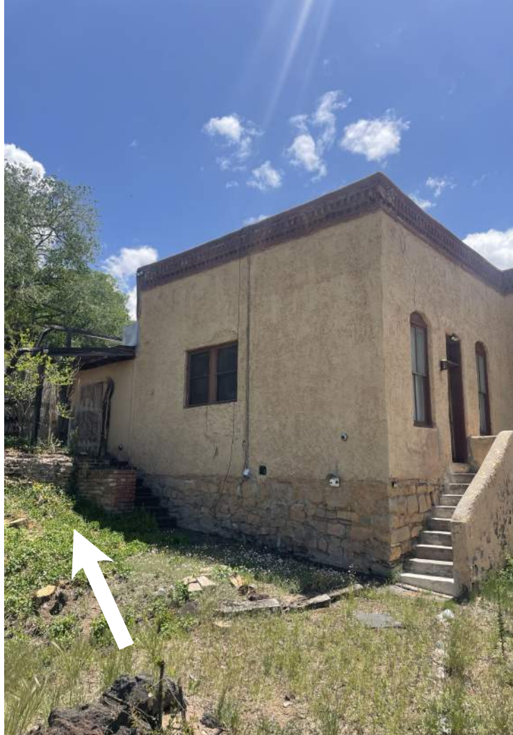
SITE WALL AT WEST ELEVATION
