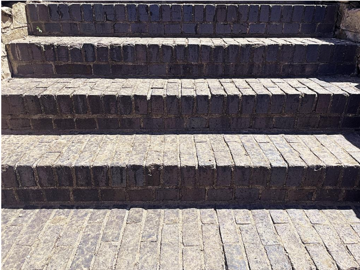
Photo 19: Brick stairs of street entry. Camera facing down.
