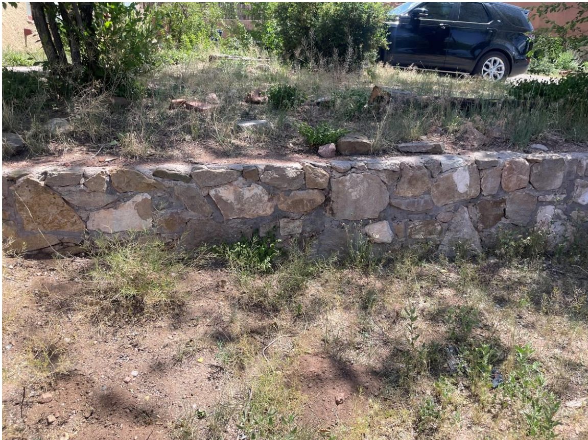
Photo 21: Minor retaining wall. Camera facing southeast.
