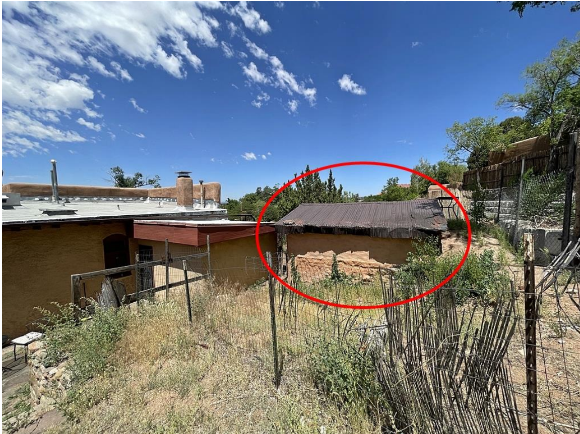
Photo 15: Shed. East elevation. Camera facing northwest.
