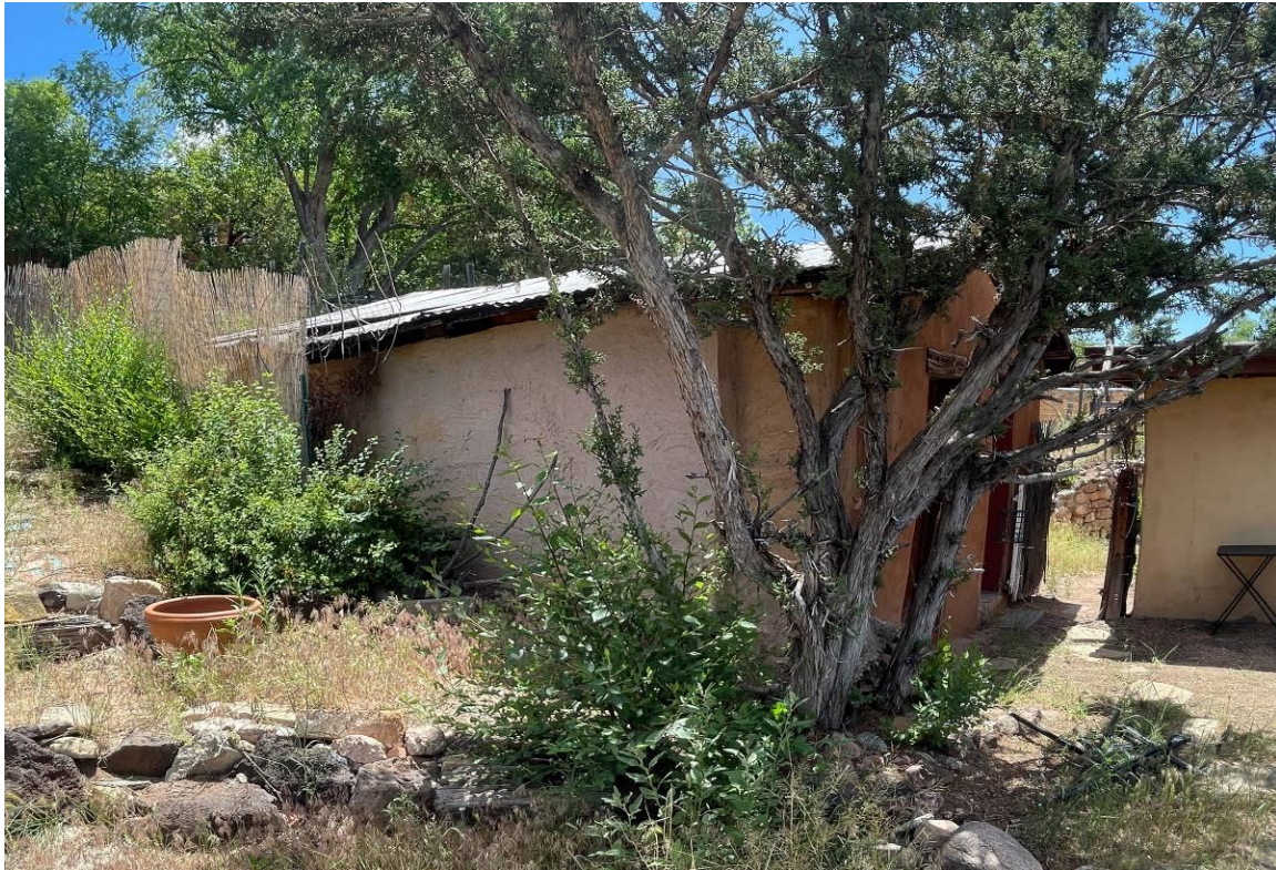
Photo 17: Shed. West elevation. Camera facing northeast.
