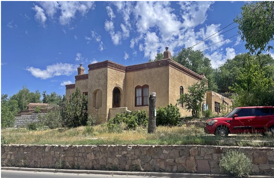
Photo 2: Setting. Camera facing northwest.
