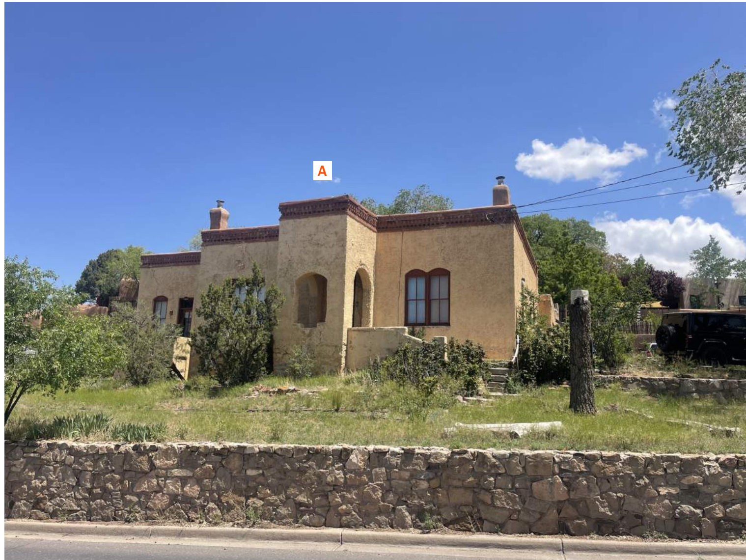
SITE FROM SOUTH
