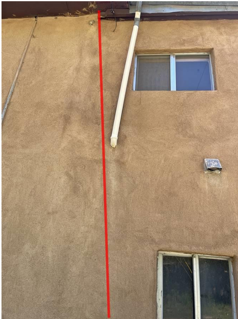
Photo 12: North elevation. Addition at northwest corner. Camera facing up.
