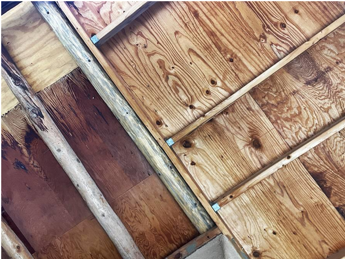
Figure 5: Joining of two non-historic porches at southwest corner of south (front) elevation. Camera facing up.
