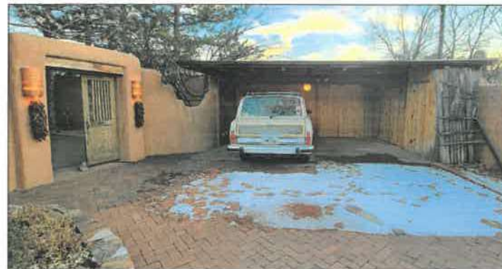
EXISTING CONDITIONS FOR CARPORT CONVERSION TO A GUESTHOUSE.
