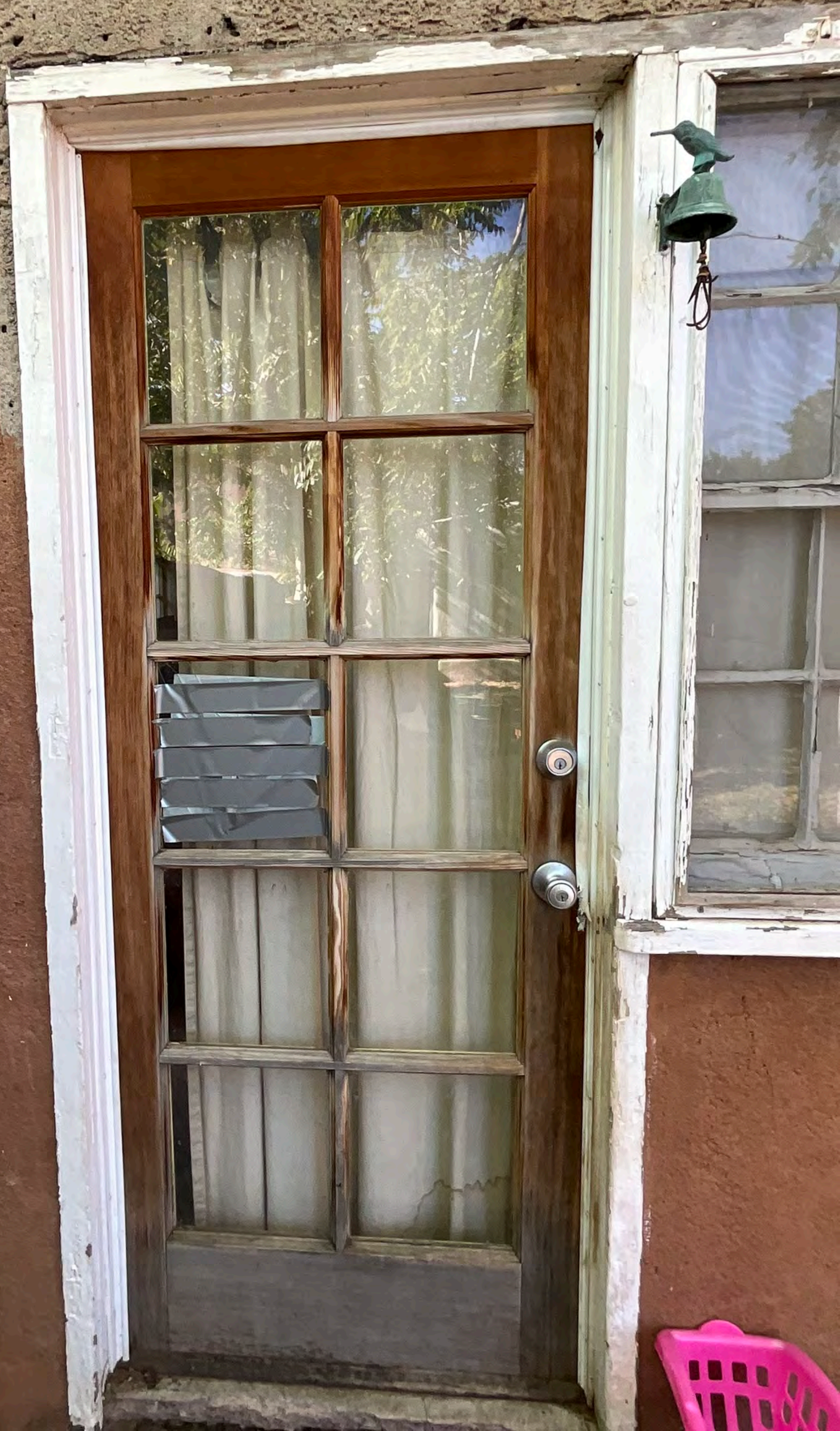
North Elevation Door #2
