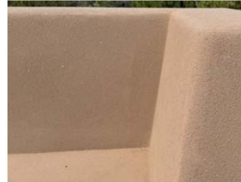
Proposed integrally colored stucco will match the color and texture of the existing Botanical Garden.
