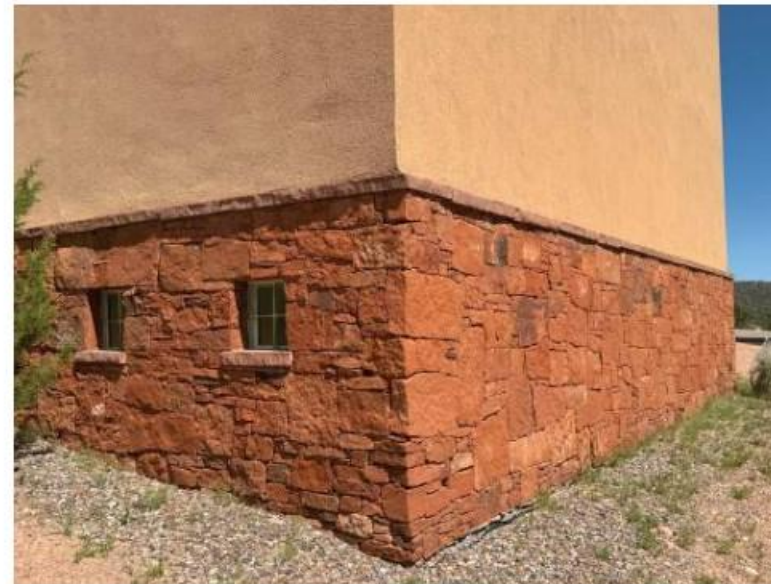
Integrally colored stucco walls at the adjacent Museum of International Folk Art.
