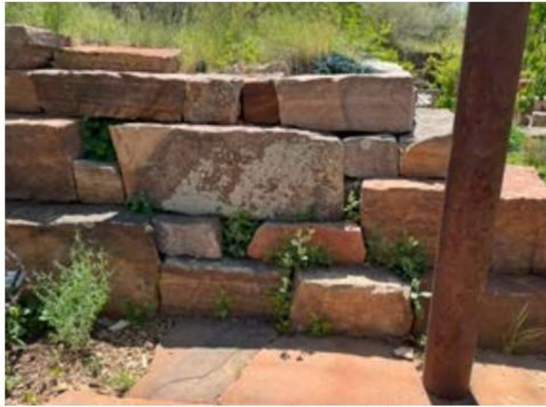
Existing moss rock masonry walls found throughout the Santa Fe Botanical Garden.
