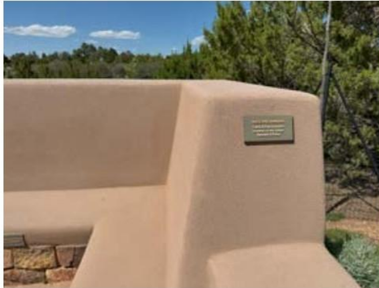
Existing integrally colored stucco site walls found in the Santa Fe Botanical Garden.
