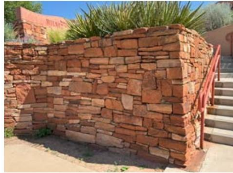
Stone masonry walls at the adjacent Museum of New Mexico Milner Plaza.
