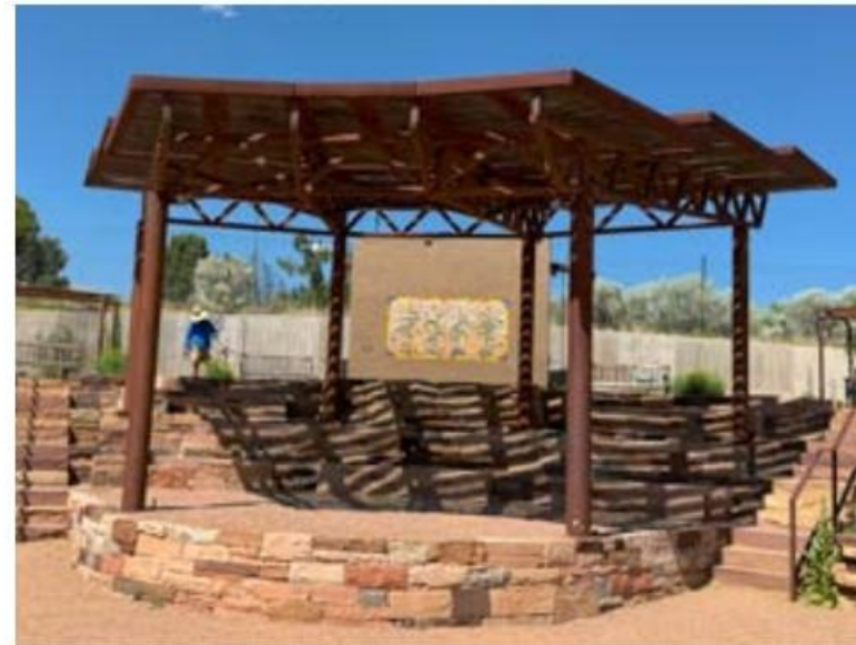
Existing weathered steel shed ramadas located at the Ojos y Manos within the Santa Fe Botanical Garden.
