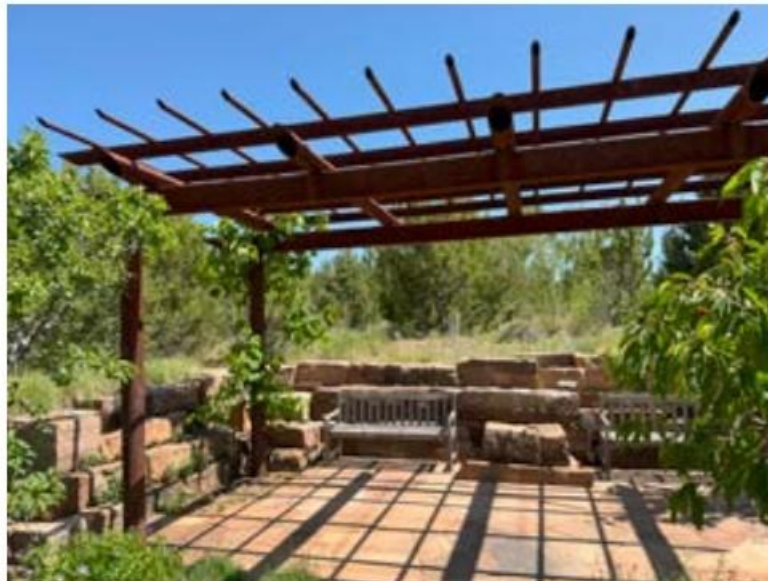
Existing weathered steel ramadas located at the Orchard Gardens within the Santa Fe Botanical Garden.
