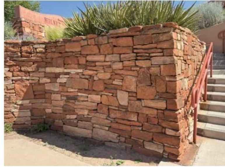
Stone masonry walls at the adjacent Museum of New Mexico Milner Plaza.
