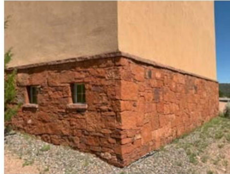
Integrally colored stucco walls at the adjacent Museum of International Folk Art.
