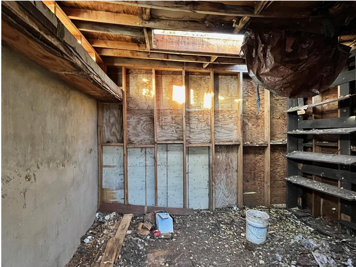
Photo 26: Photo 25: Shop. Addition, interior. Camera facing north.
