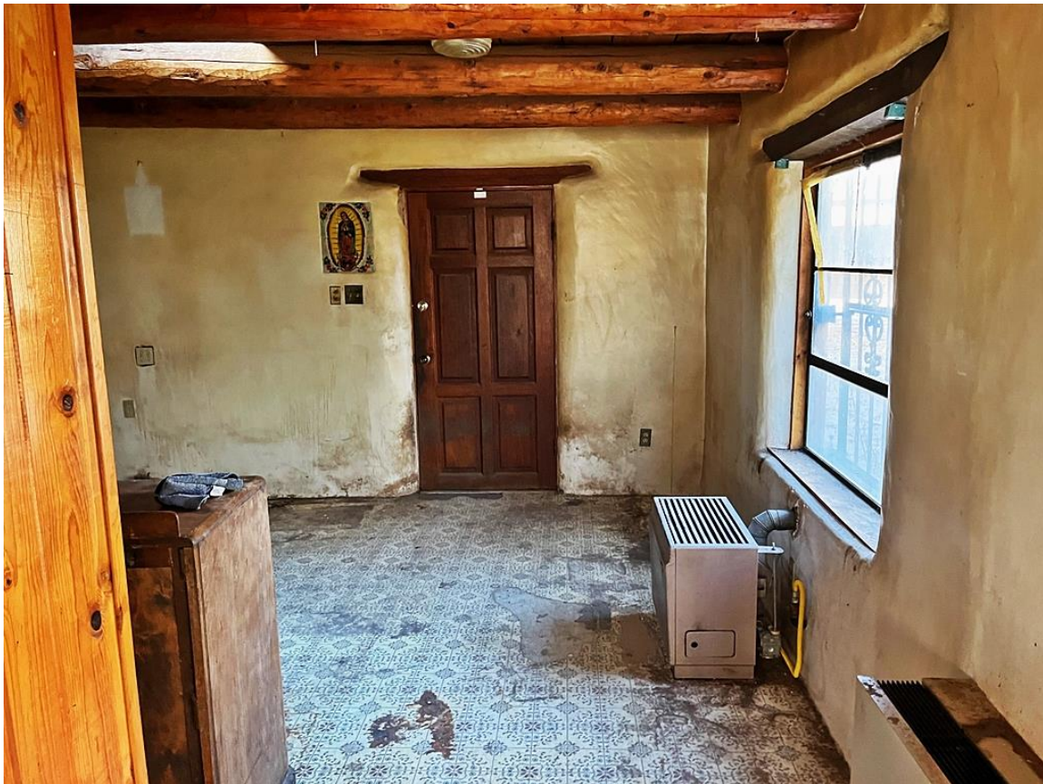
Photo 22: 1980s addition. Camera facing north.
