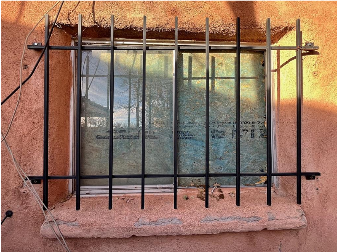
Photo 14: South elevation. Window of southeast room of the original core. Camera facing north.
