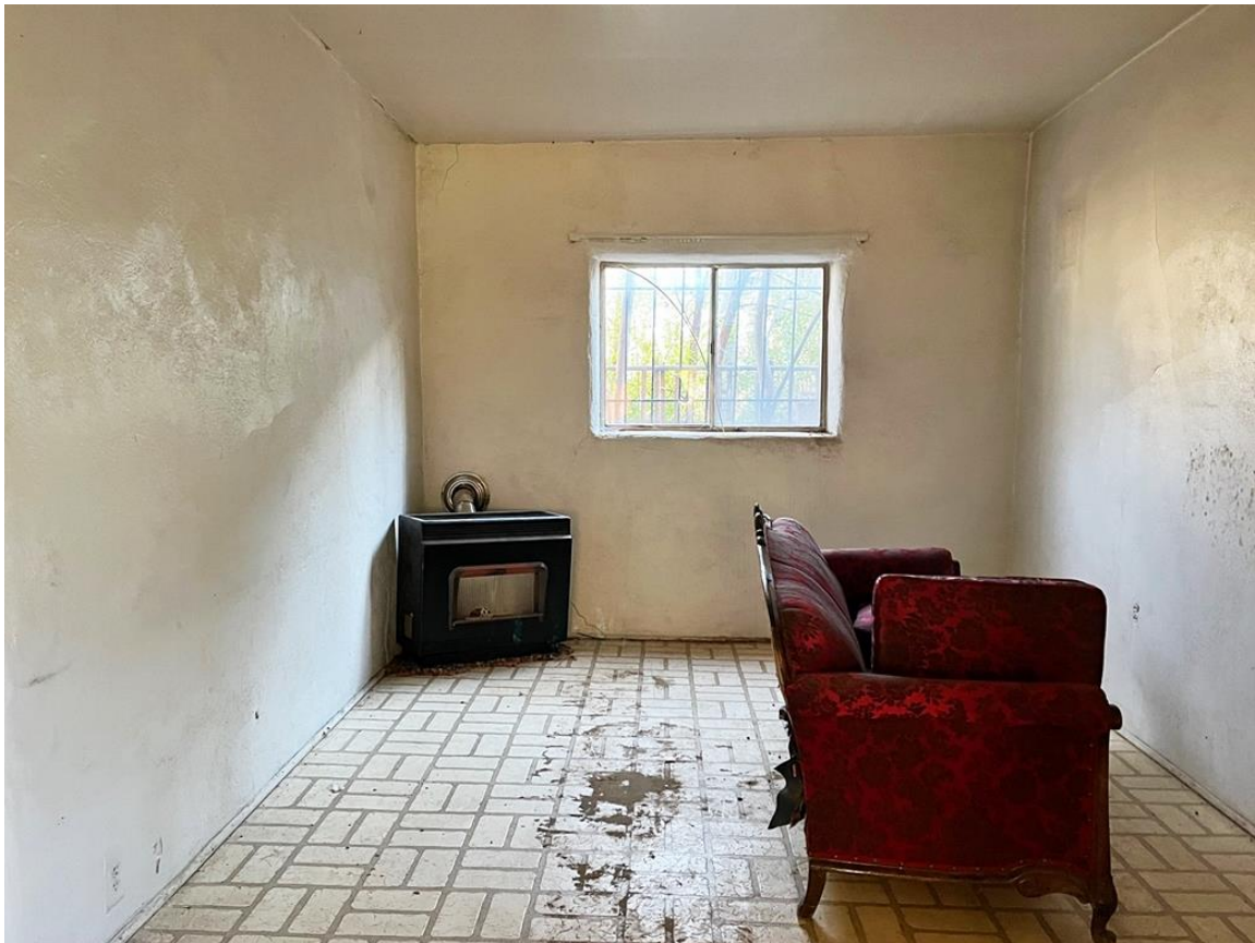
Photo 19: Southwest room of the original core. Camera facing south.
