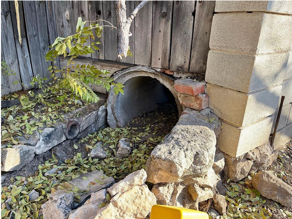
Photo 4: Assumed acequia segment tracing east side of property. Camera facing southeast.
