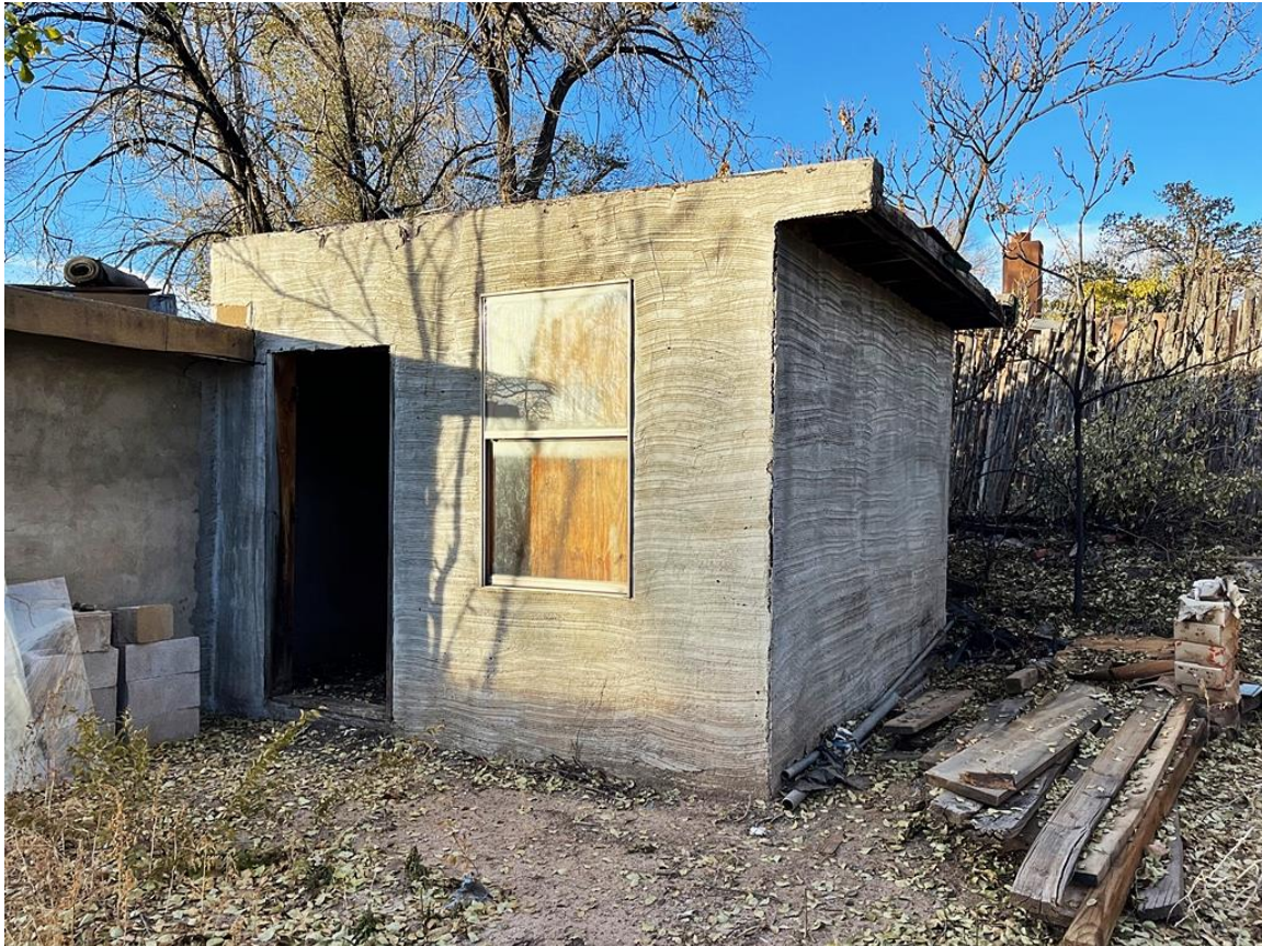
Photo 25: Shop. Addition. Camera facing northwest.
