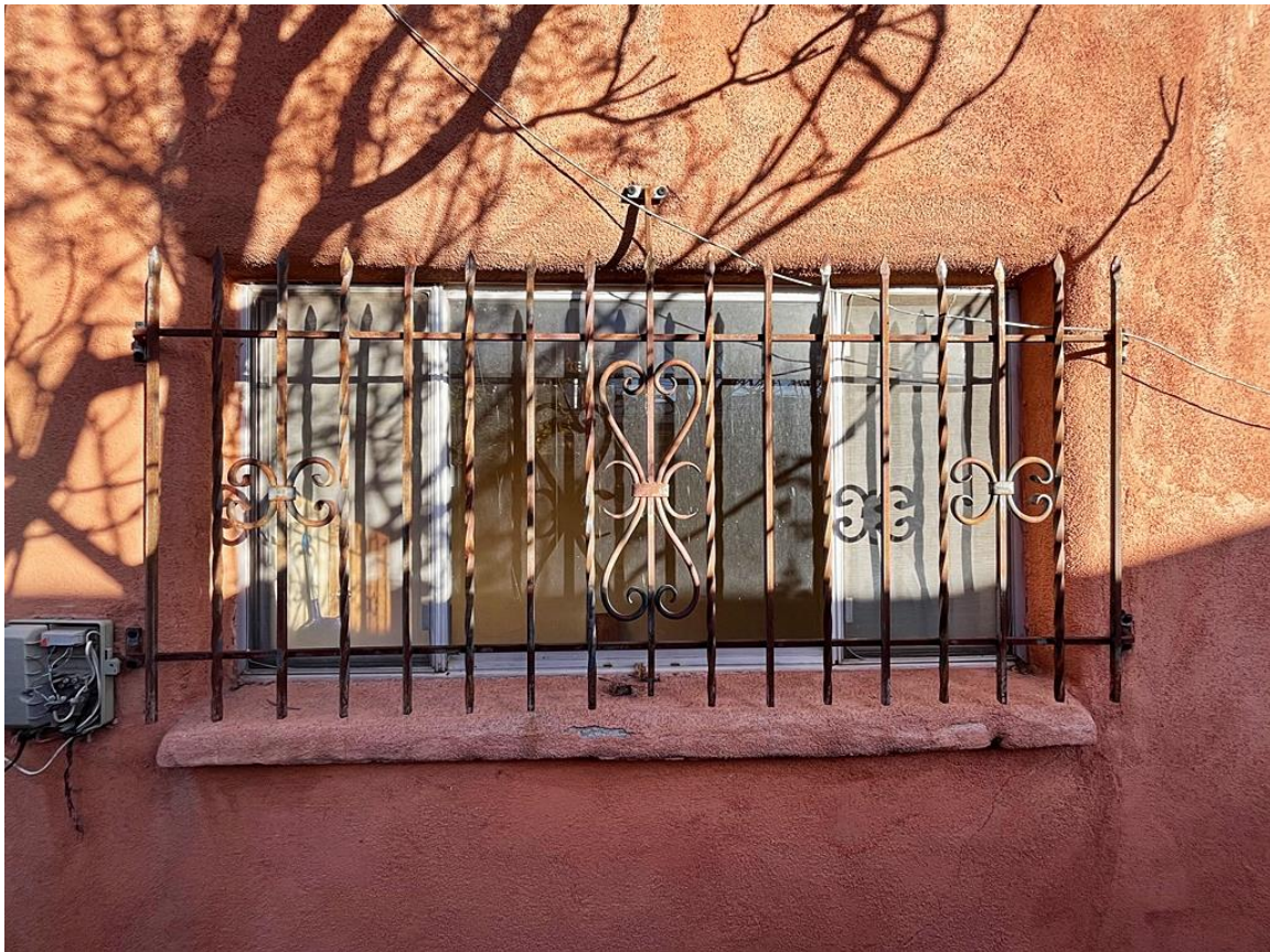
Photo 17: West elevation. Window of northwest room of the original core. Camera facing east.
