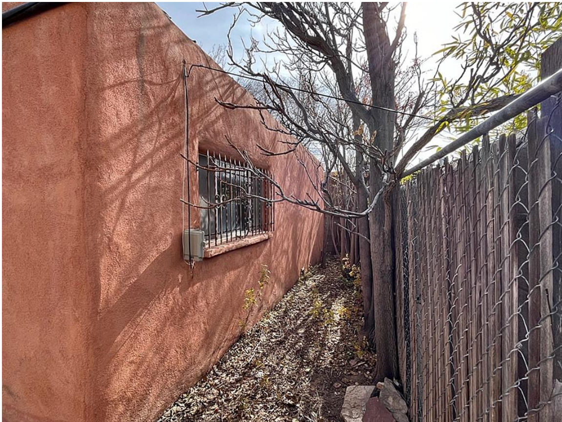
Photo 16: West elevation. Camera facing southeast.
