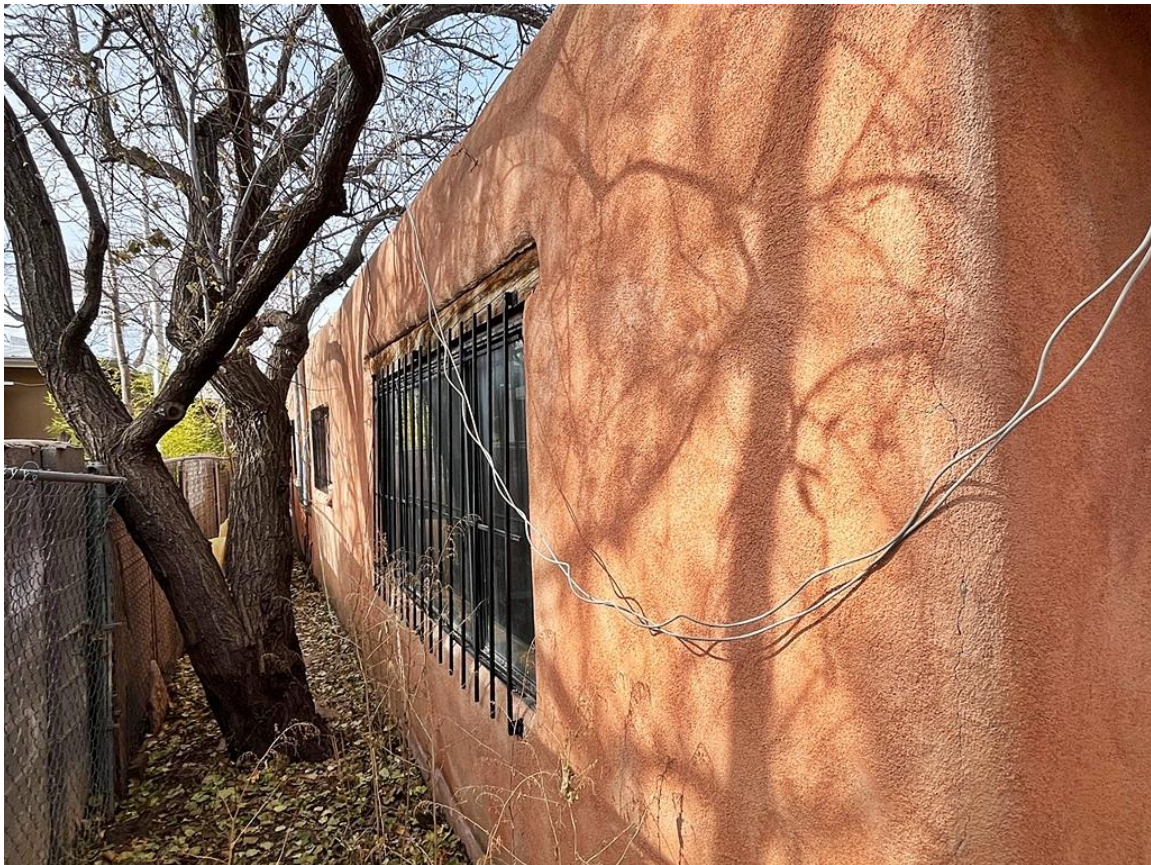
Photo 11: South elevation. Camera facing northwest.
