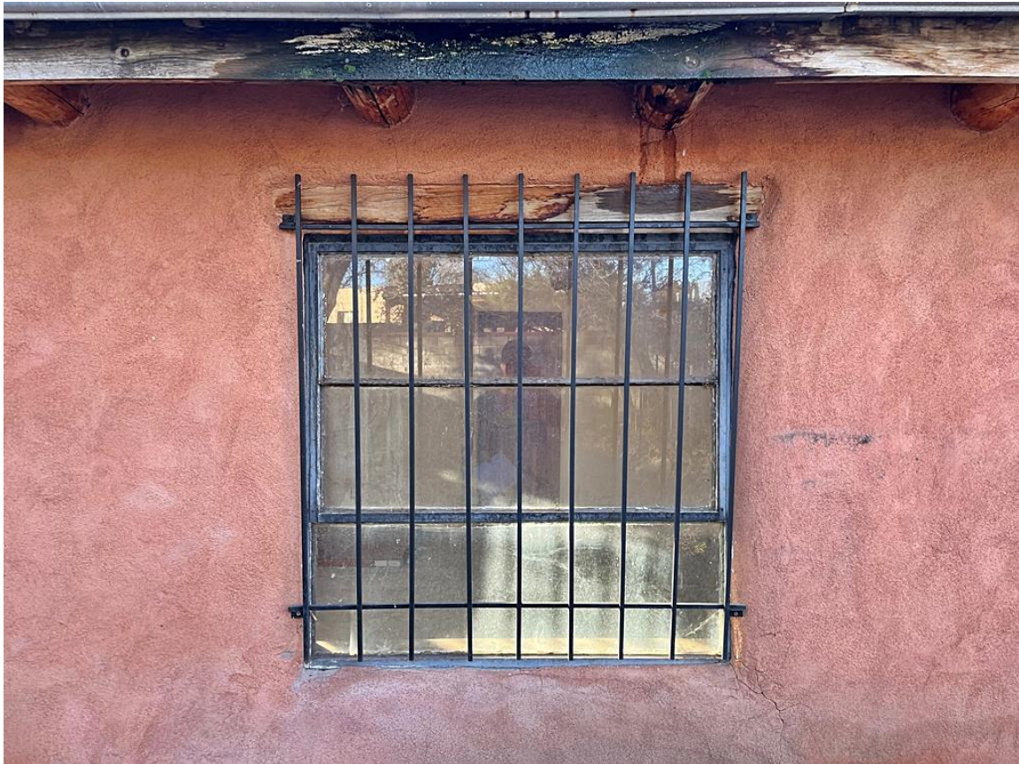
Photo 10: East elevation at 1980s addition. Window detail. Camera facing west.
