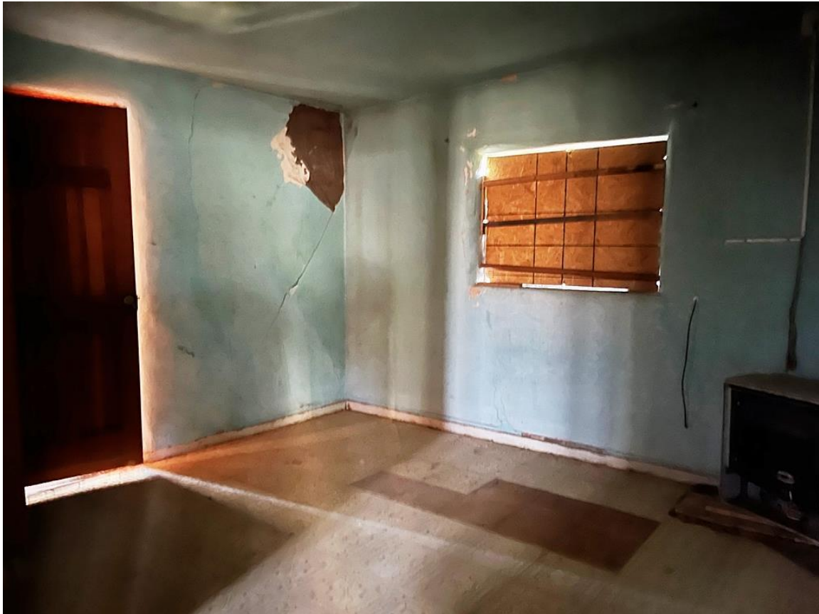
Photo 20: Southeast room of the original core. Camera facing southeast.
