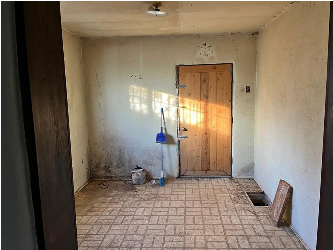
Photo 18: Northwest room of the original core. Camera facing north.
