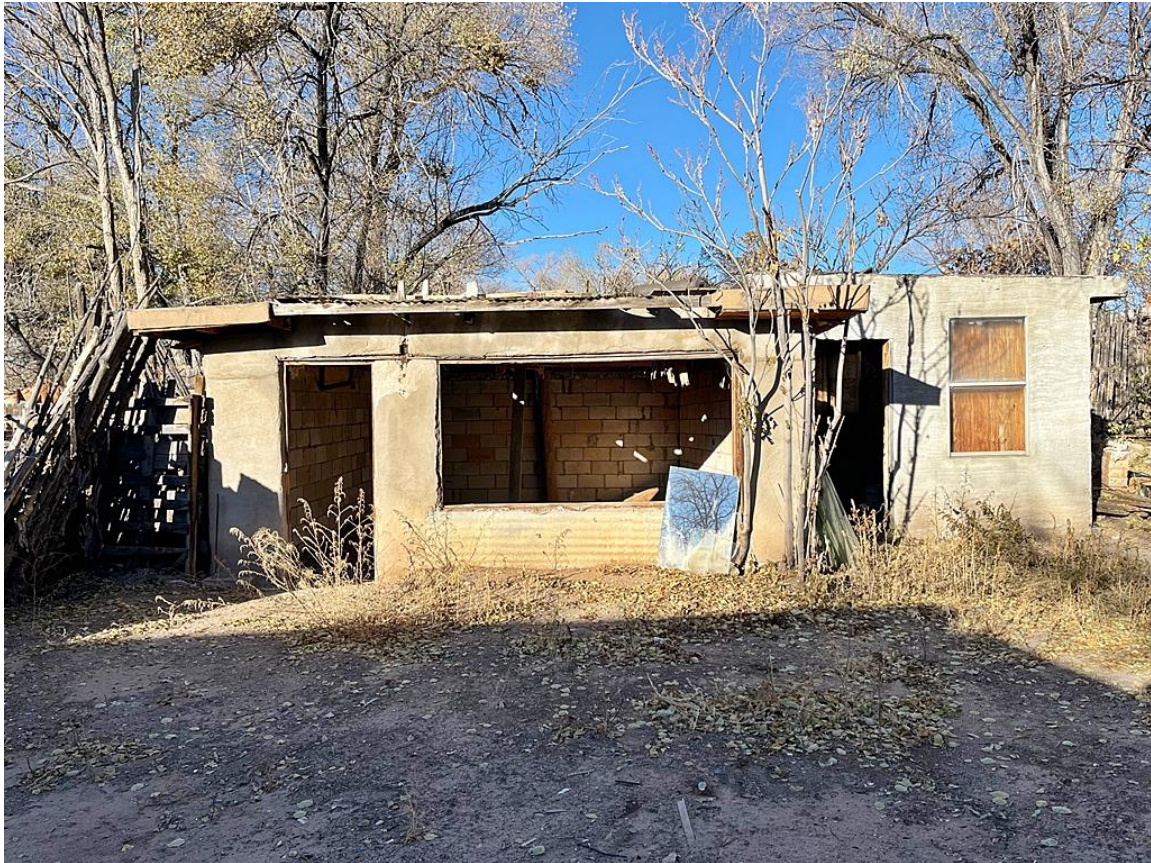
Photo 23: Shop. South elevation. Camera facing north.
