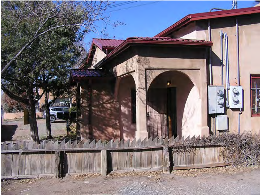
5 - East Façade (southeast corner)
