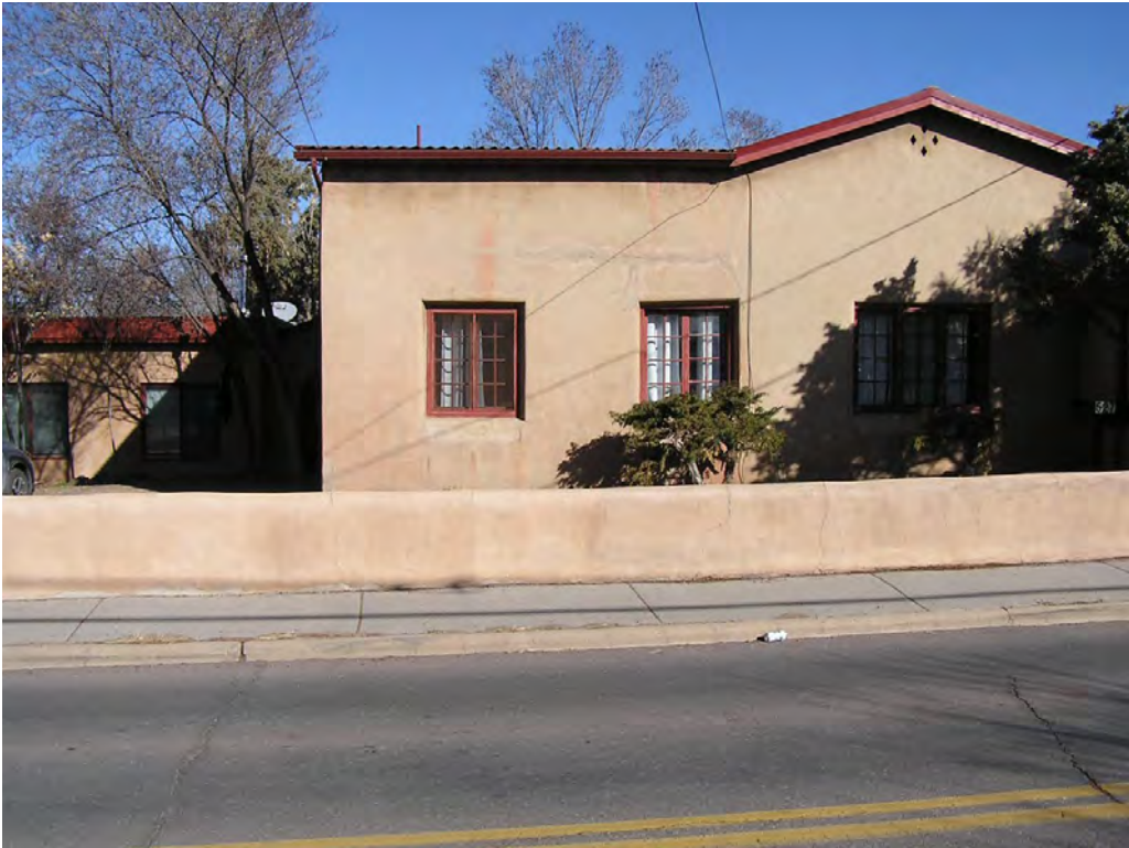
3 - South Façade (facing Agua Fria)
