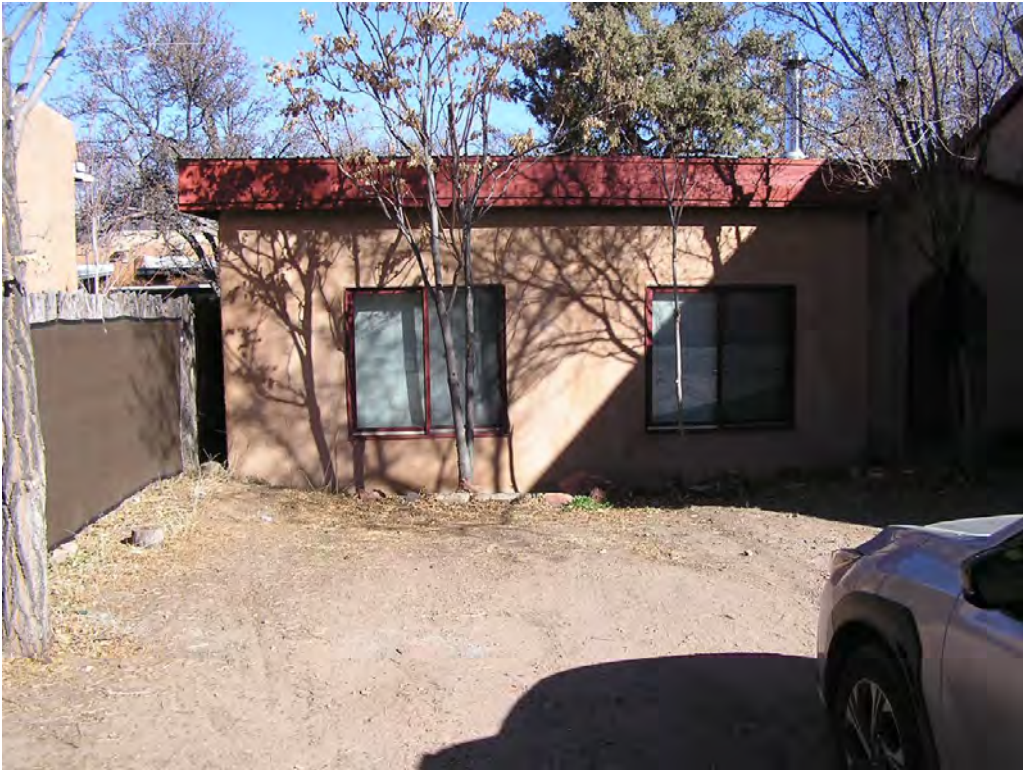
1 - South Façade (facing Agua Fria)
