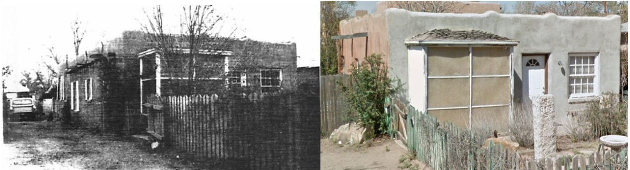
Figure 2: South and West Facades in 1985 (HCPI photo) and 2025.
