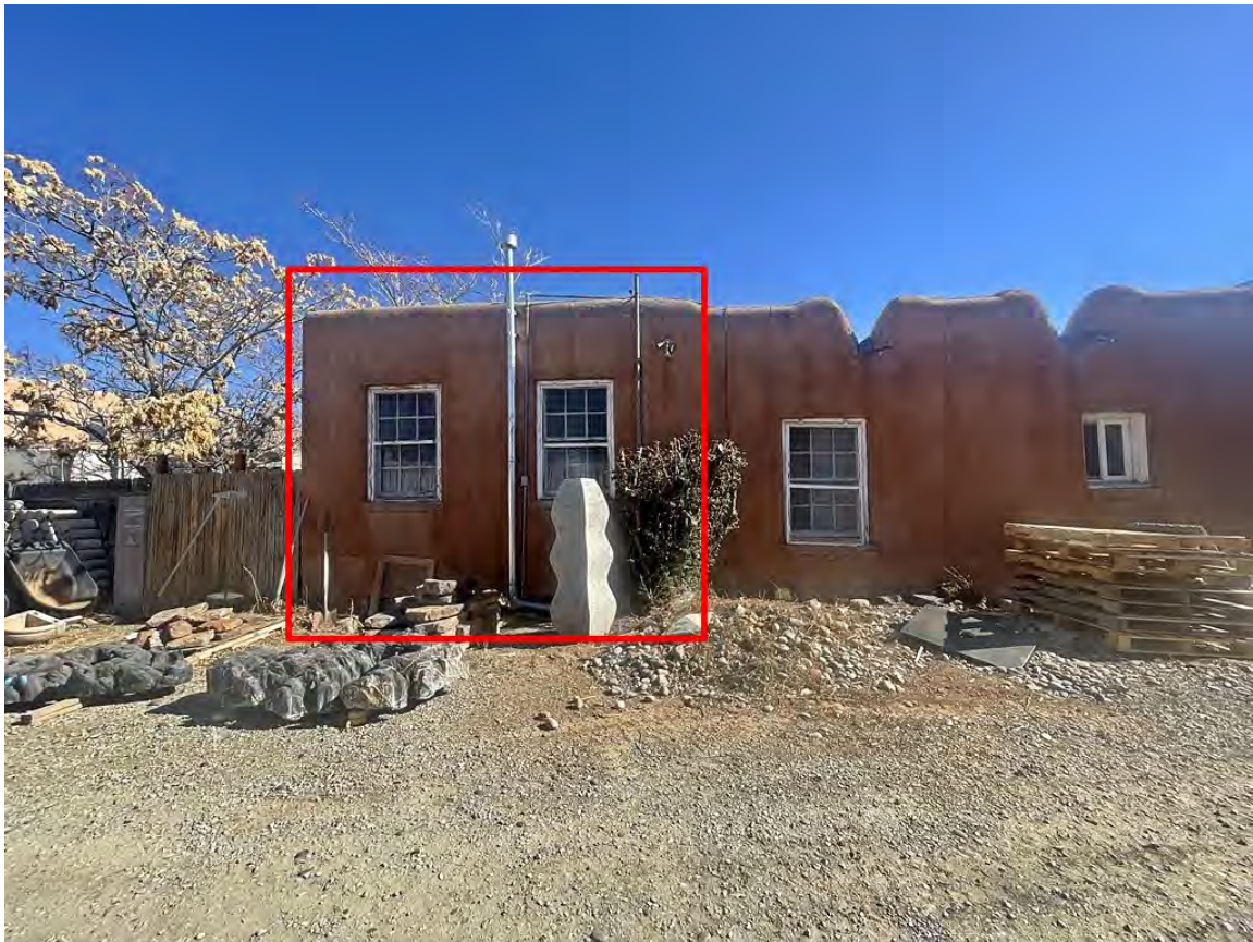
Photo 9: West elevation. Mudroom addition highlighted in red. Camera facing east.
