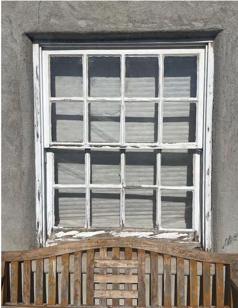
Photo 5: South (front) façade. Detail of east window. Camera facing north.
