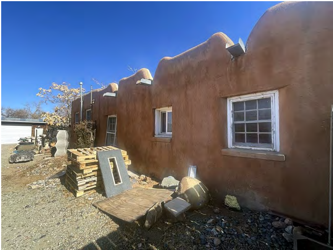
Photo 6: West elevation oblique. Camera facing northeast.
