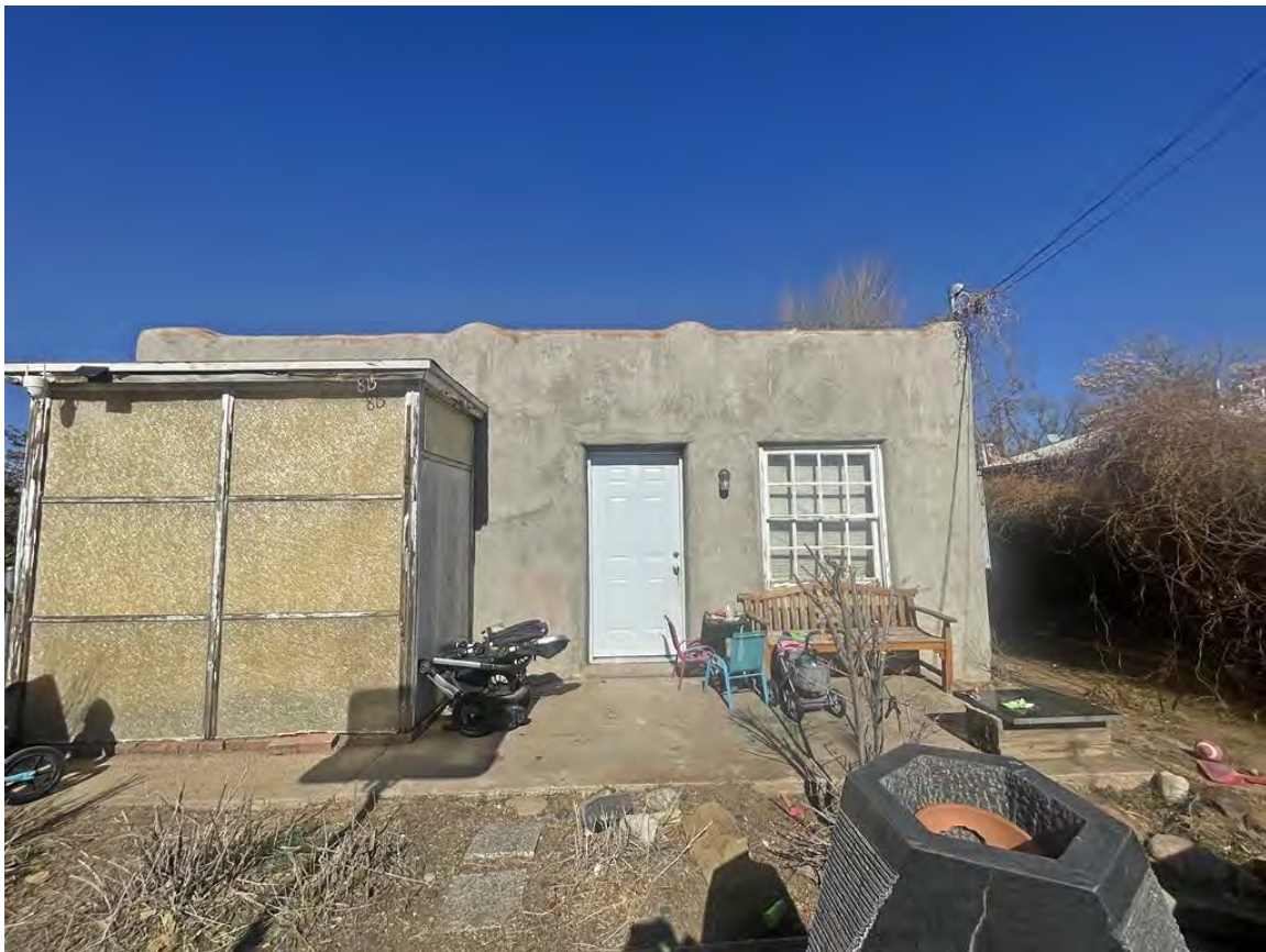
Photo 2: South (front) façade. Camera facing north.
