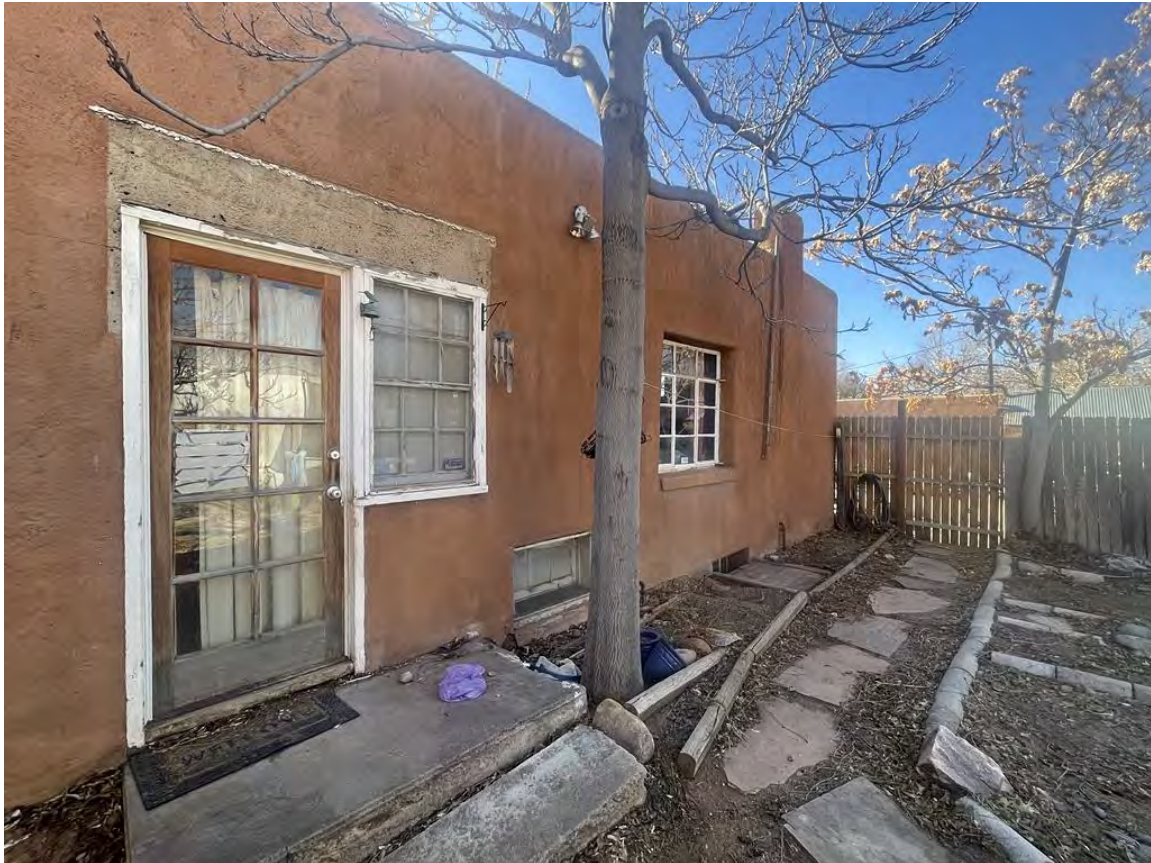
Photo 10: North elevation oblique. Camera facing southwest.
