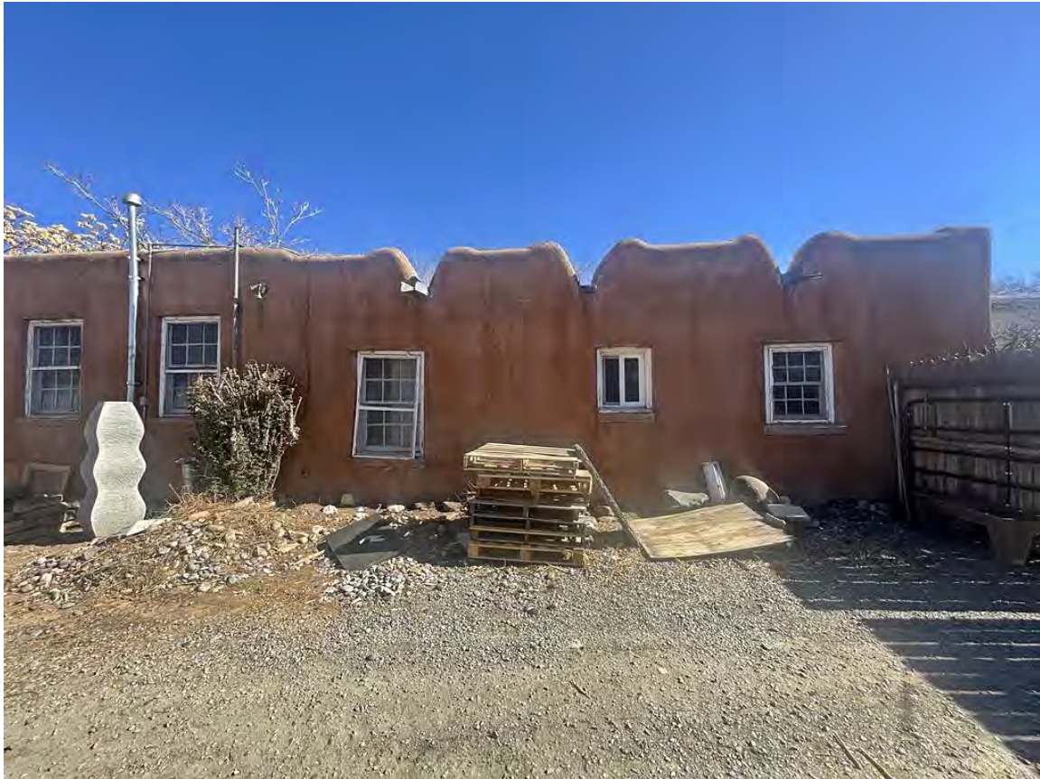
Photo 7: West elevation. Camera facing east.
